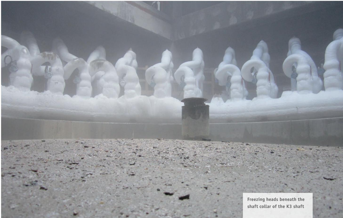
Freezing heads beneath the shaft collar of the K3 shaft
