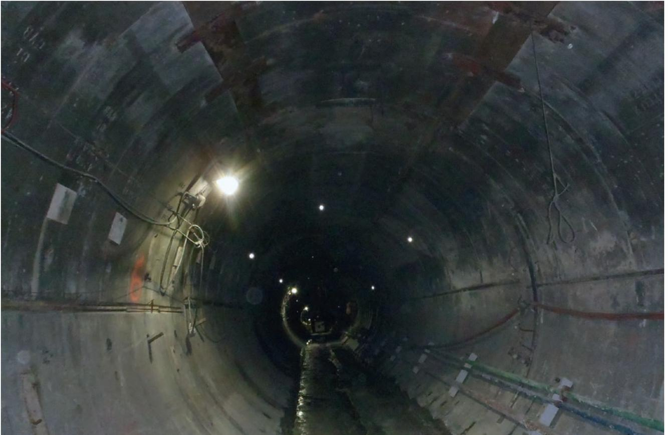
The primary MDS-tunnel with concrete-segment lining
