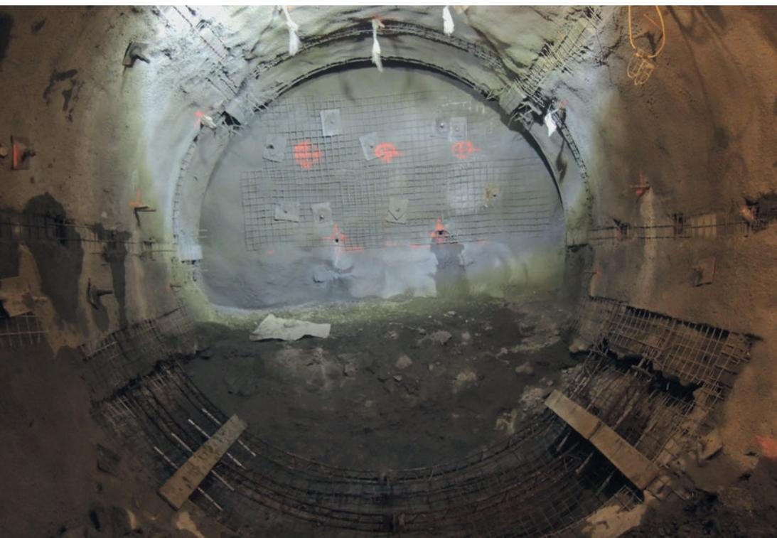
Full assembled steel mesh, ready to applicate shotcrete
