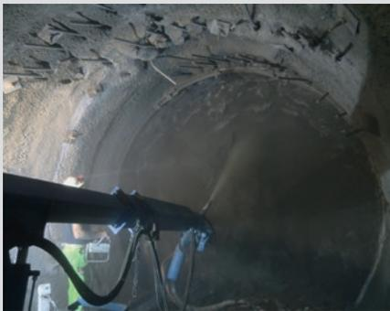
Shotcrete manipulator MEYCO Oruga with telescopic arm applicator the first support layer
