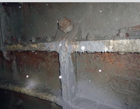
Leakage of grouting material between tubbings
