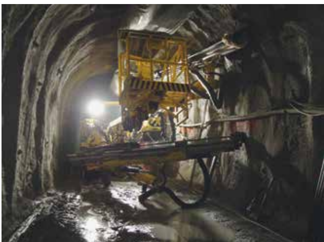
Drilling with Atlas Copco drilling jumbo
