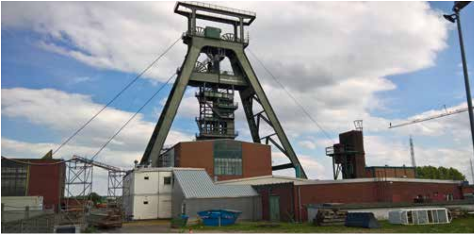
Shaft tower Konrad shaft I, view from west
