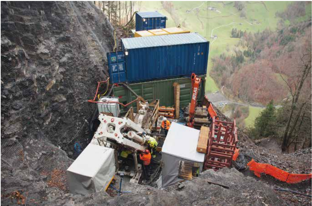
Raise boring site
