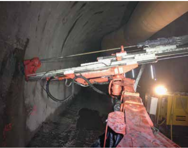
Installation of the support system with jumbo
