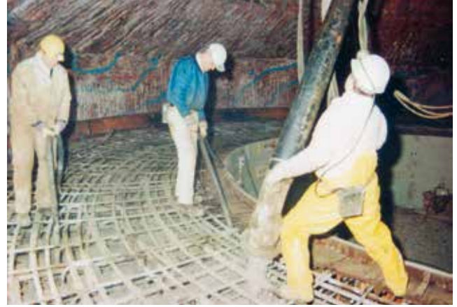
Constructing the foundation for the sliding shaft lining
