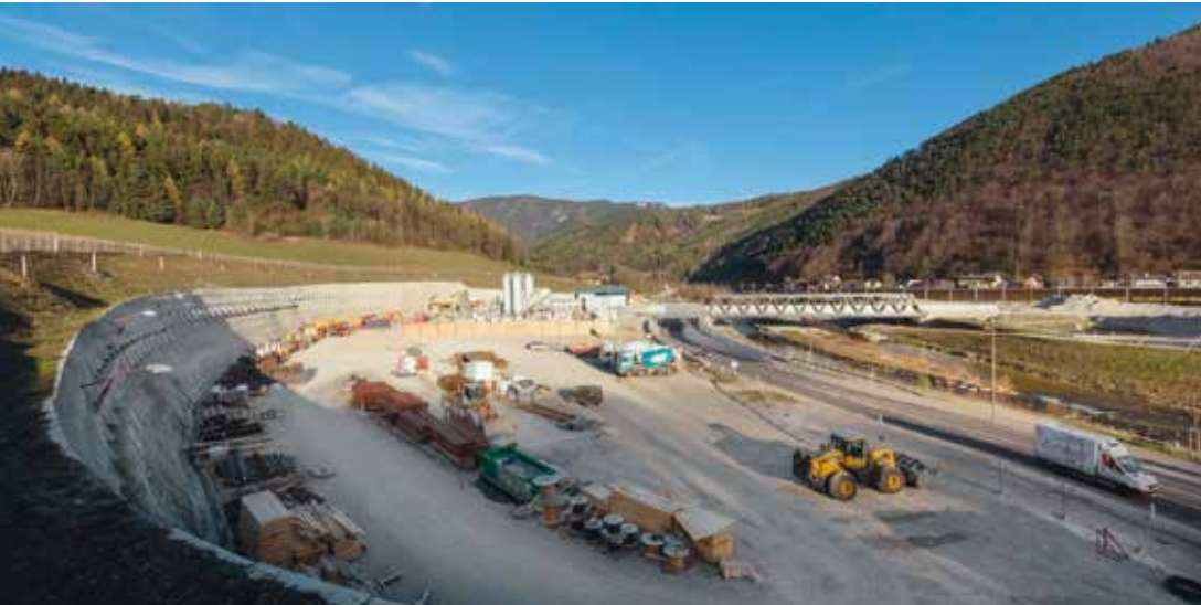
Gloggnitz construction site
