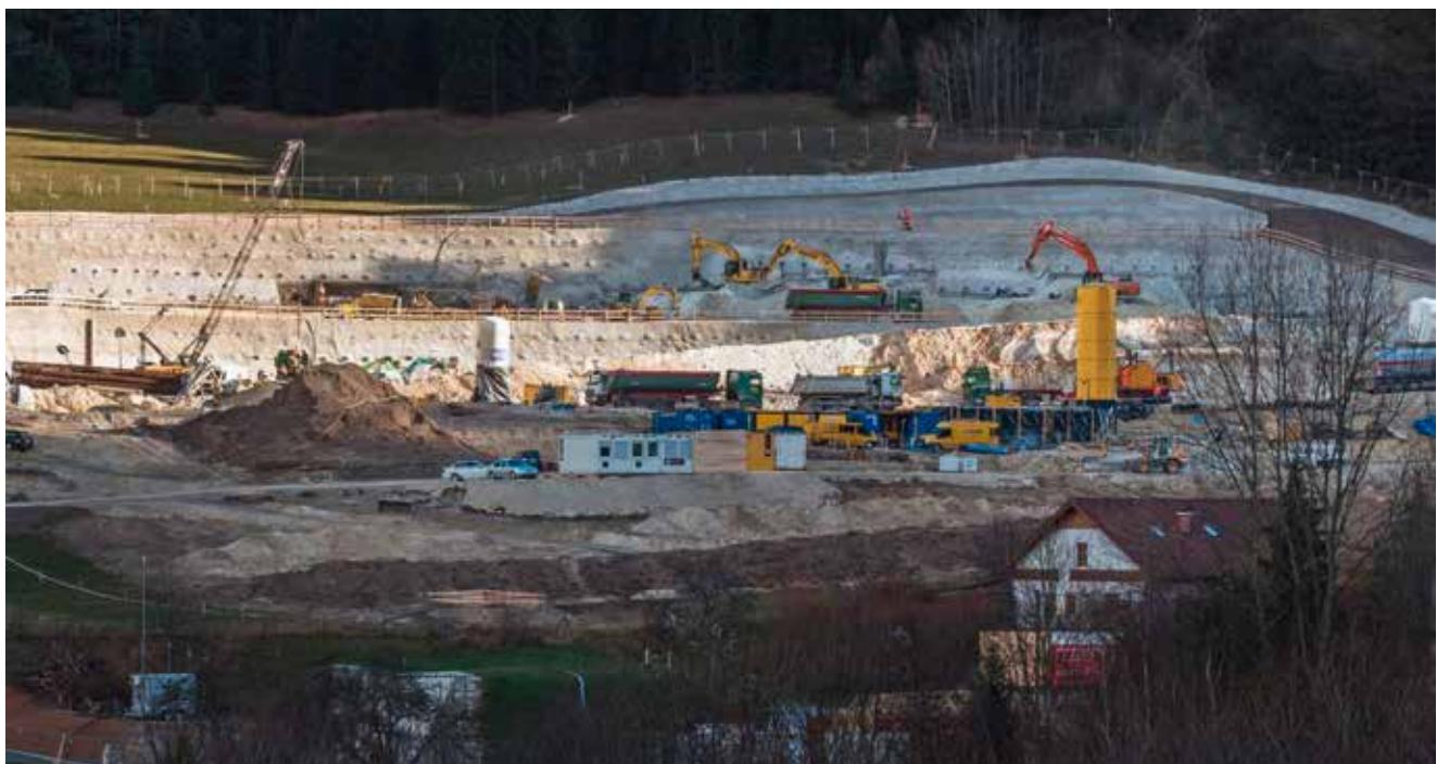
Earthworks and specialist civil engineering work for the Göstritz pre-cut
