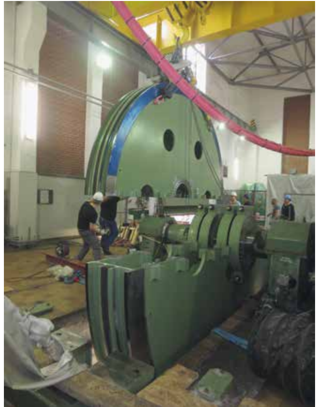
Erecting the second half of the single-rope winder
