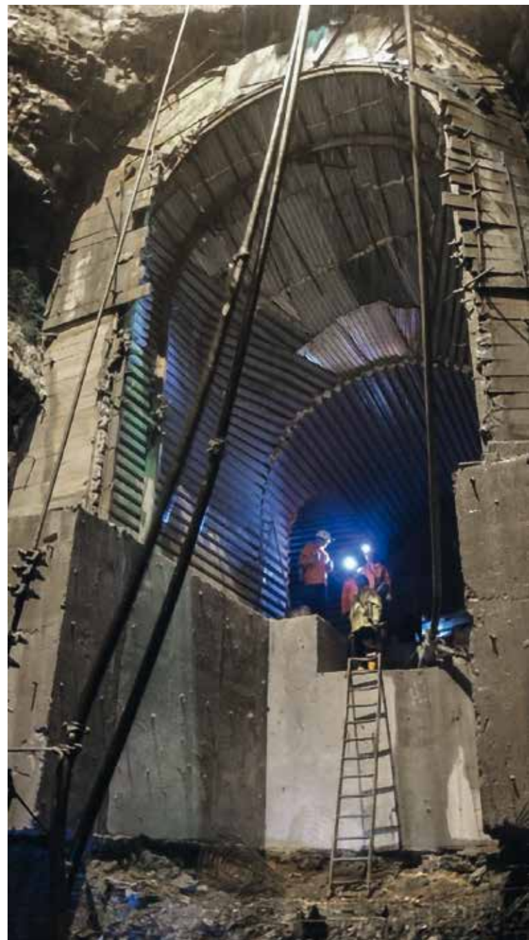
Concrete supports in the pump chamber
