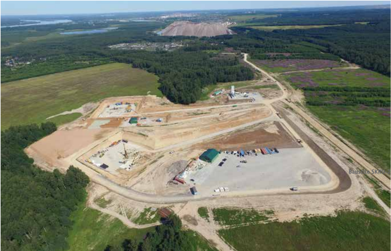
The SKRU-2 shaft site. State of work July 2016 (7 months after procurement). In the background can be seen the salt spoil tip for SKRU-2 mine, the town of Solikamsk and the river Kama. Copyright Uralkali
