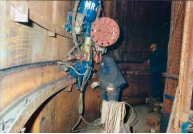
Automated welding of the steel casing before the construction of the inner lining
