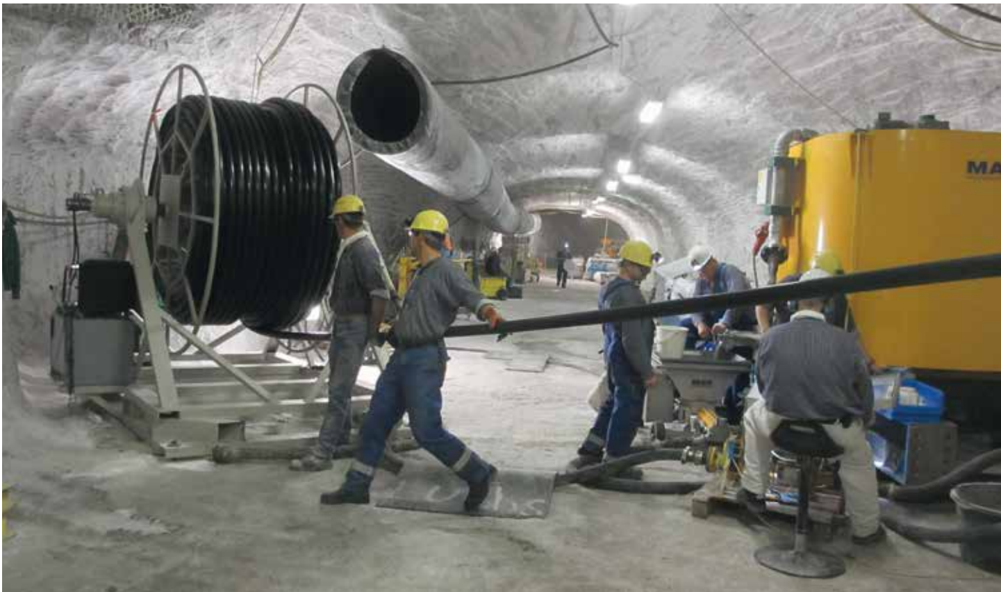
Deep borehole filling with PE hose coil
