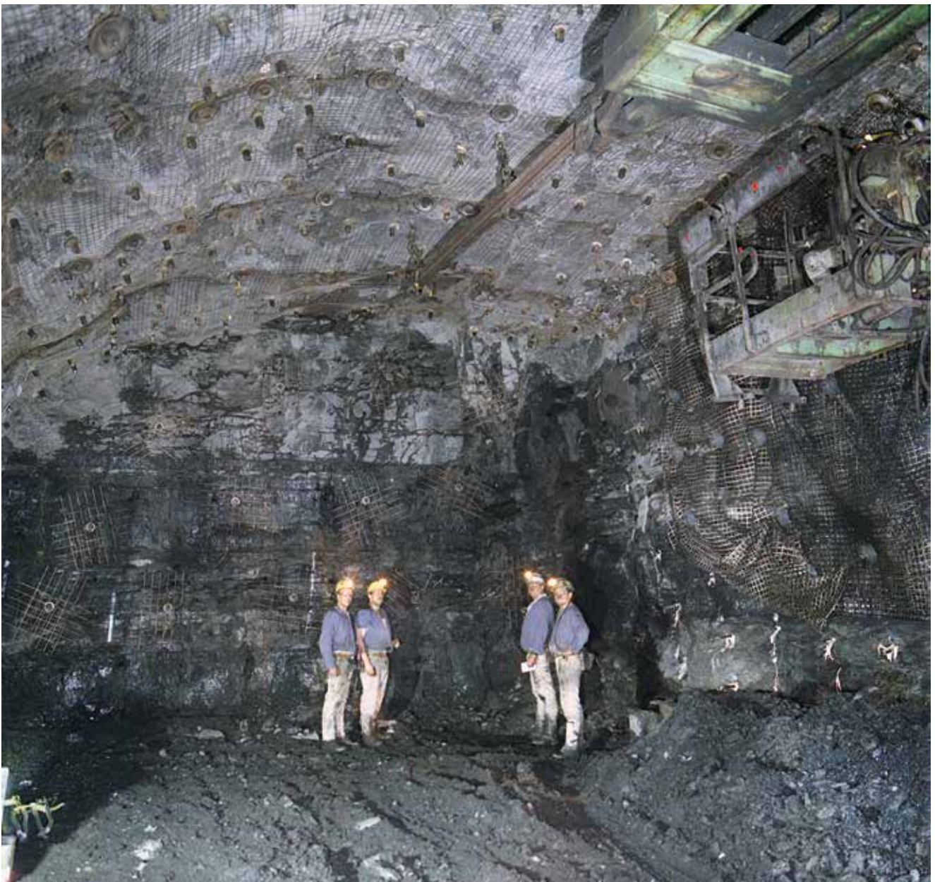
Roofbolt supports in the pre-heading
