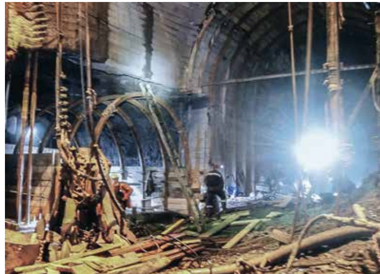
Installing the concrete formwork in the inset area
