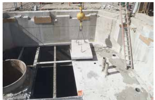
Removal of existing collar and sub-collar concrete and steel beams
