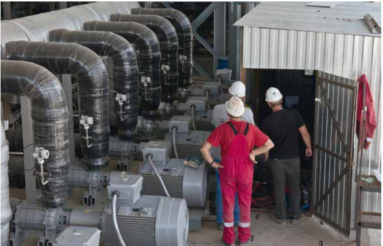
TS employees controlling the freeze plant
