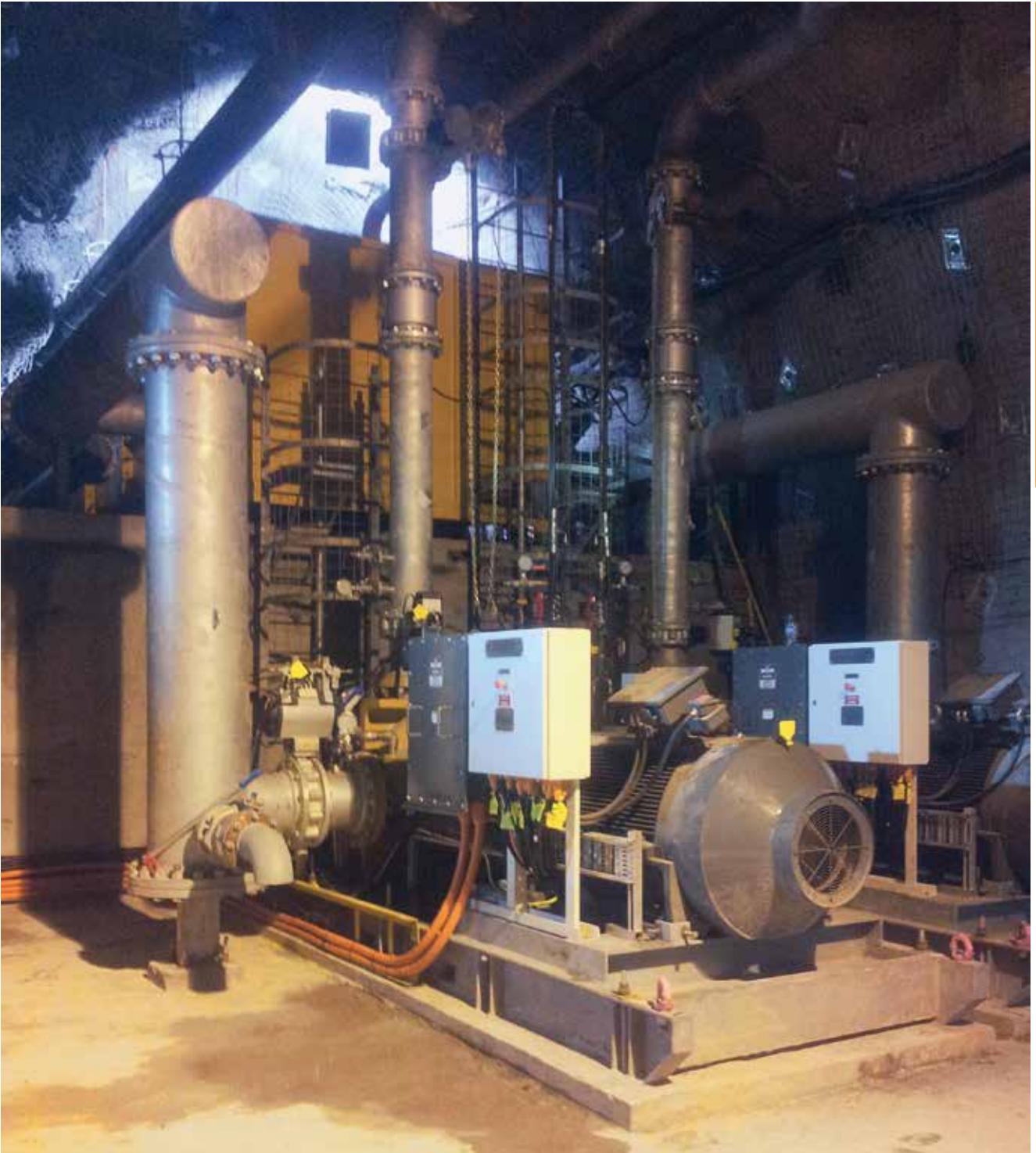
Underground mine dewatering system
