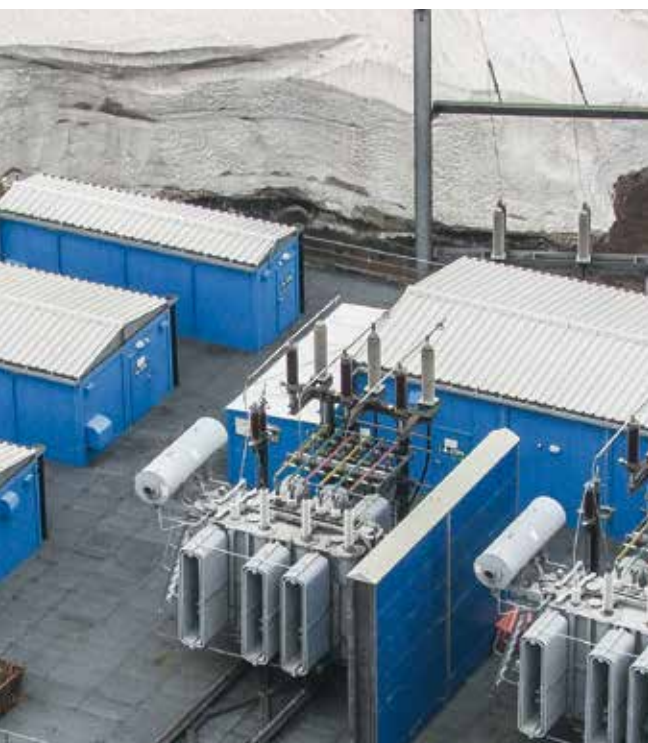
Main electrical substation
