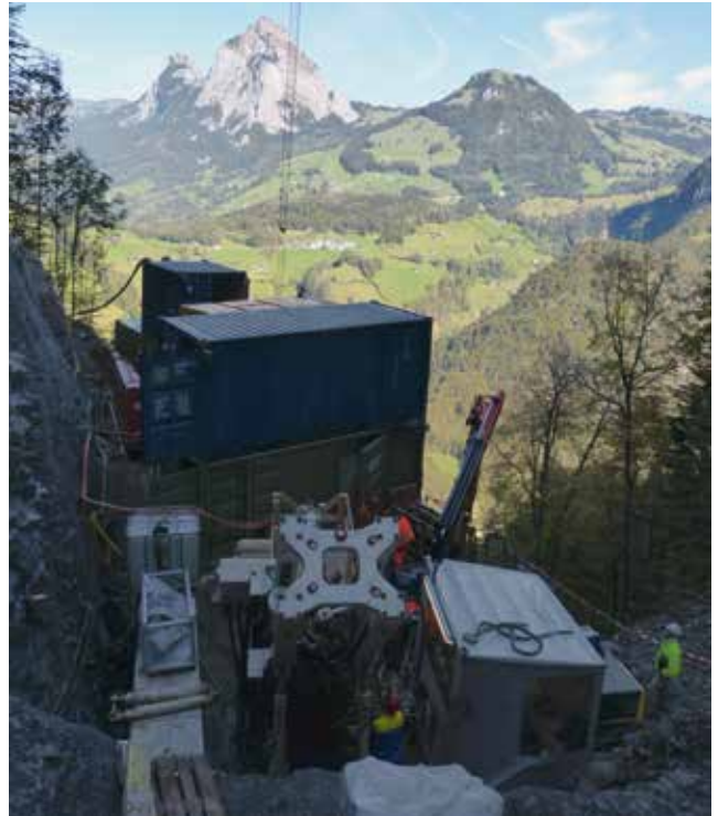
A great challenge: The installation of the raisebore machine in the rock face
