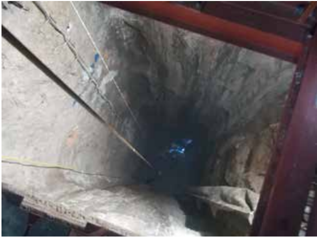
Square cross-section of the shaft
