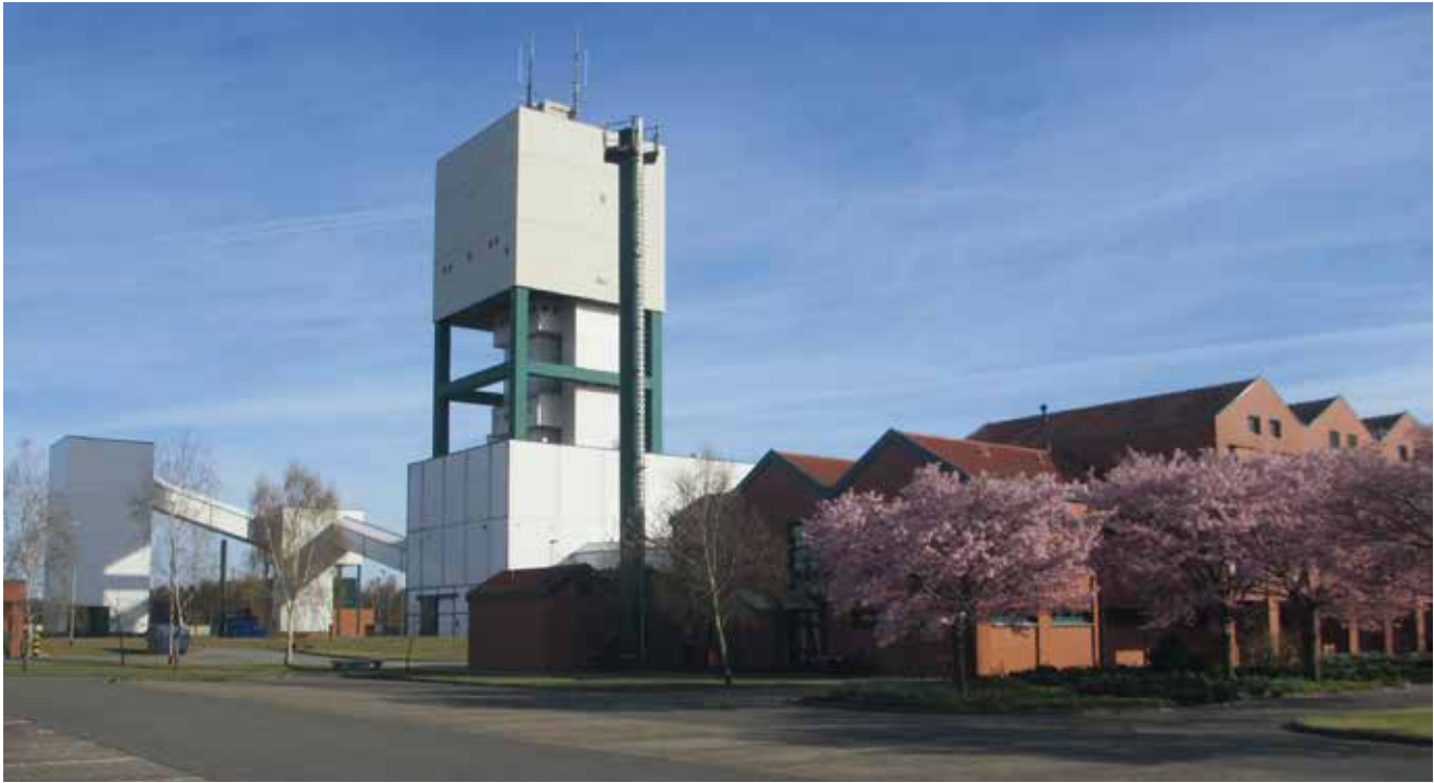
Gorleben no. 1 shaft
