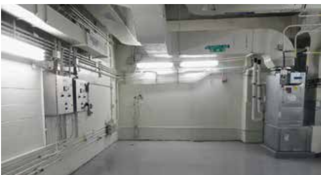
Concrete covering after successful grouting work
