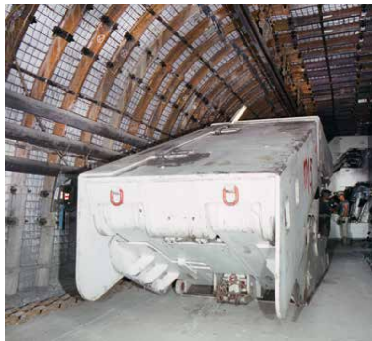
Complete shield unit at the face entry point
