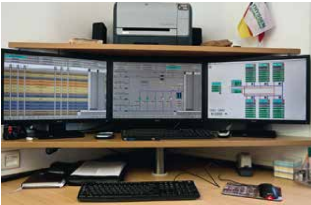
Operator's position for the controlling and timing of the freeze plant
