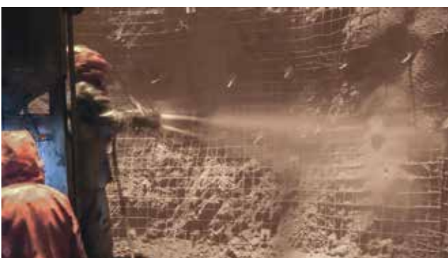
Shotcrete support for the shaft walls
