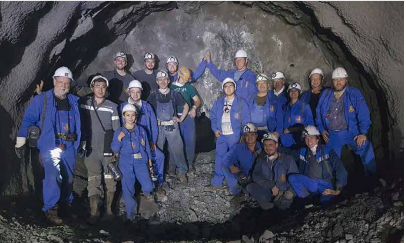
Roadheading team celebrate the breakthrough to the ventilation shaft in the company of visitors from home
