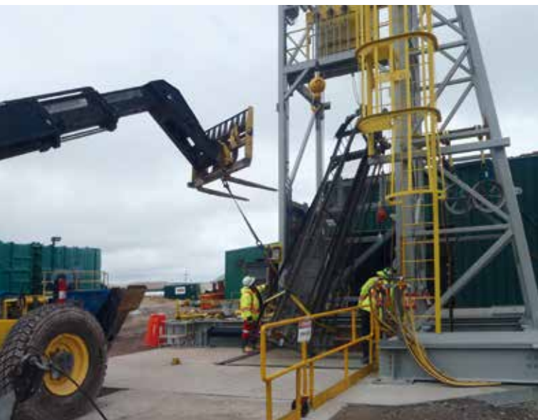
Shaft furnishings hoisted to surface and removed
