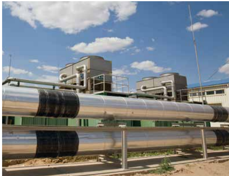
Isolated distribution pipes between freeze machines and shaft
