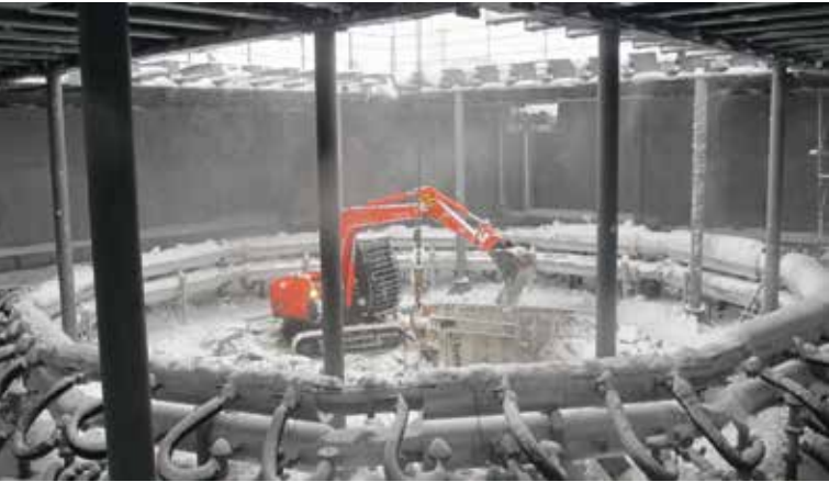
Start of building: Producing the shaft collar 13,5 m below ground level
