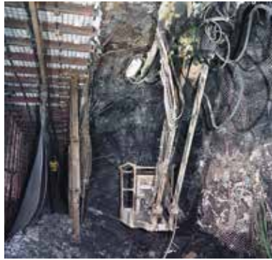
Excavating the parallel entry with the aid of a safety screen and roofbolting platform
