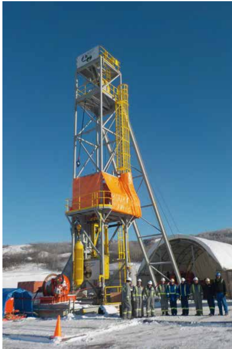
The company & Alberta Energy Regulators Group – site visit after installation of the portable headframe and hoisting plant
