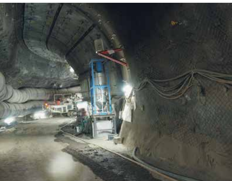
Road Section profile with bolted support
