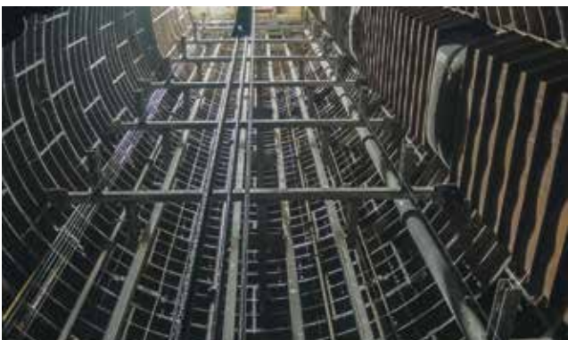
Guide fittings and tubbing supports in WS-10 shaft
