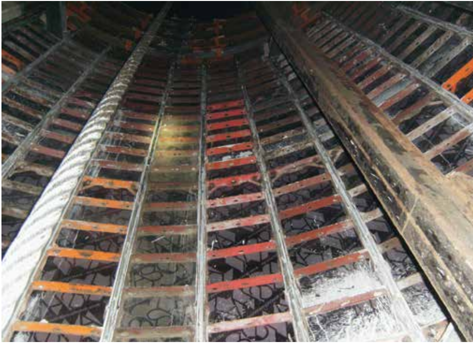
System formwork for the construction of the concrete shaft liner
