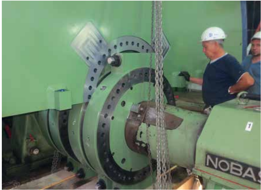
Erecting the first single-rope winder on the axle
