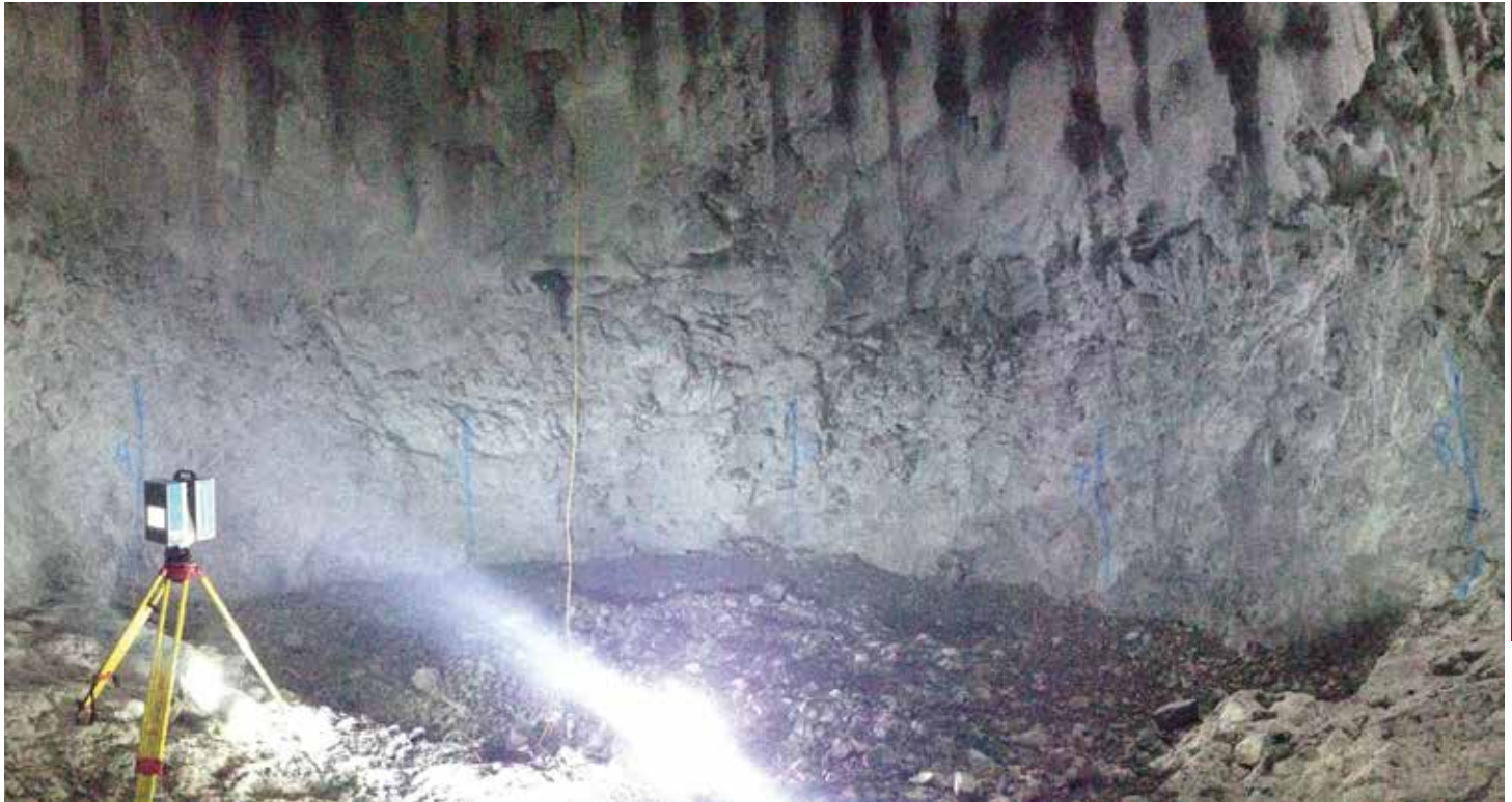
LIDAR Scanner set up on shaft bottom
