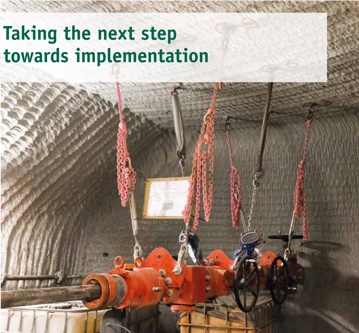
Preventer stack for the underground exploratory holes for the planning of the shaft bottom at Asse 5
