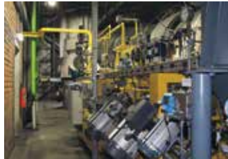
Control station HGE
