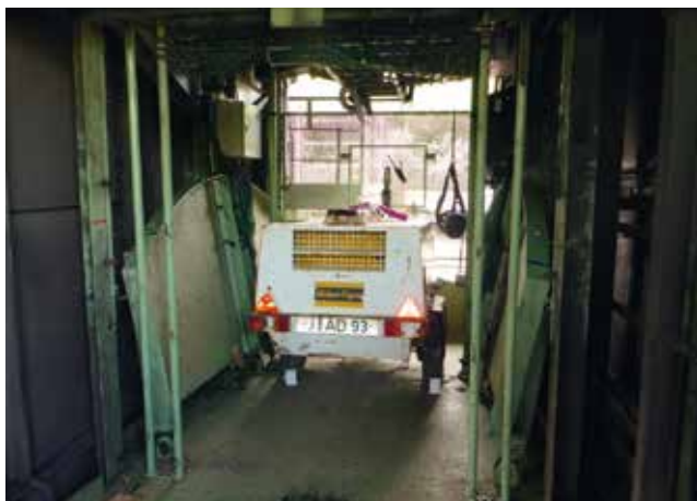
Shaft working platform with compressor at pit-bank level
