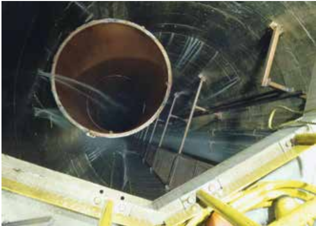
View from galloway – existing water inflow and steel furnishings
