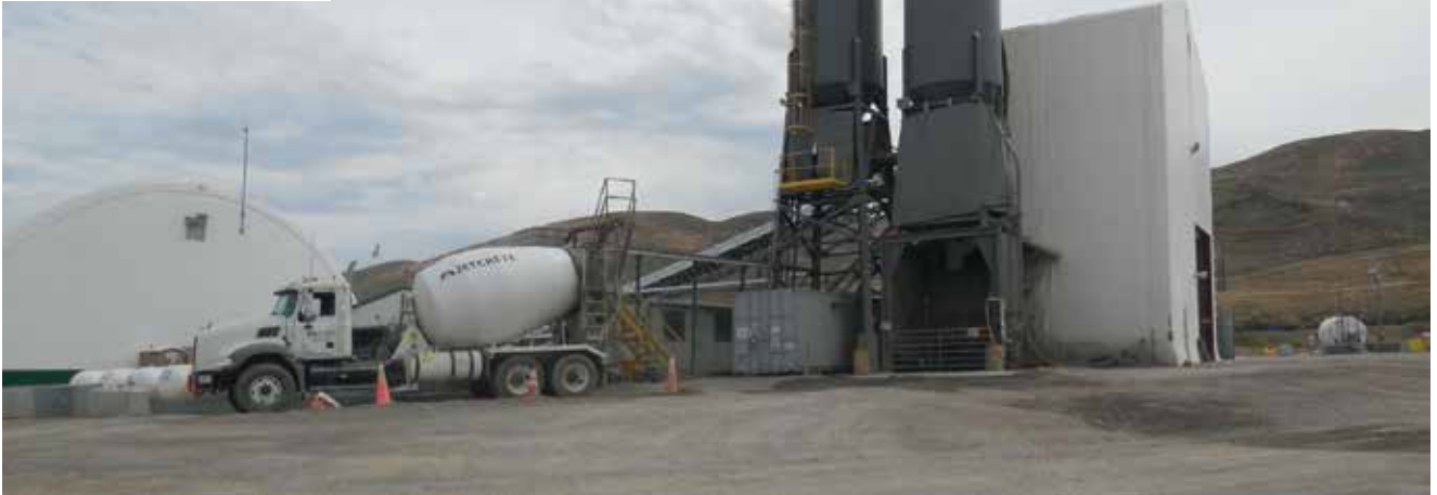
State of the art batch plant at Leeville mine, Nevada
