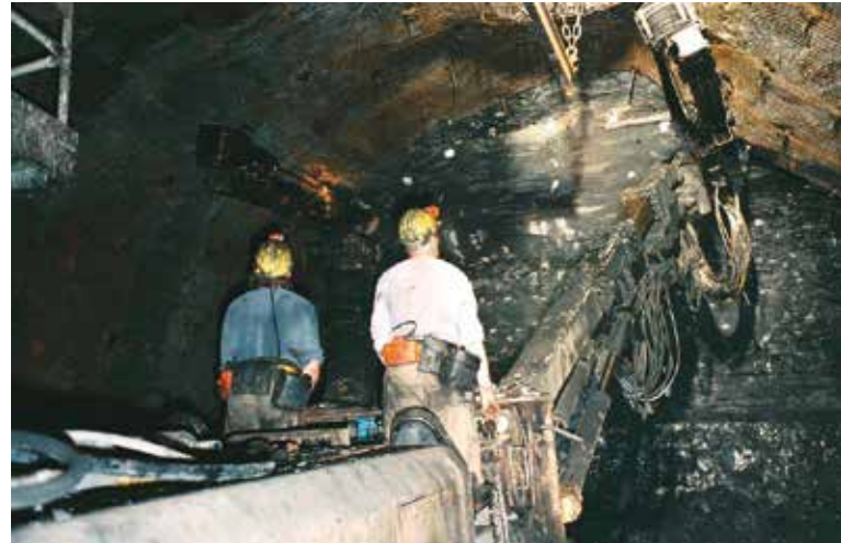
Conventional roadway drivage with blast hole drilling
