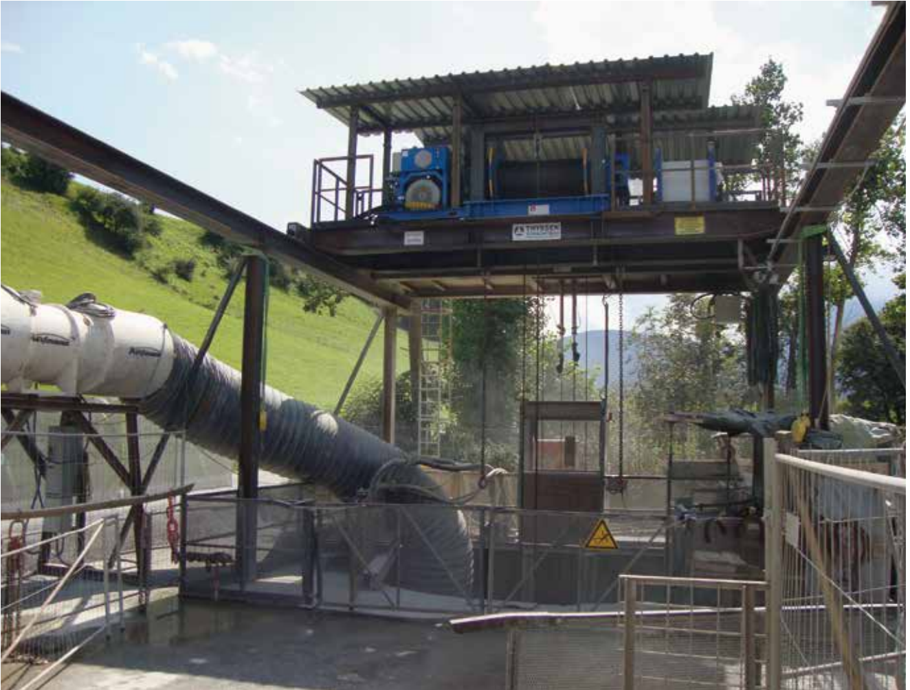
Shaft head including crane facility
