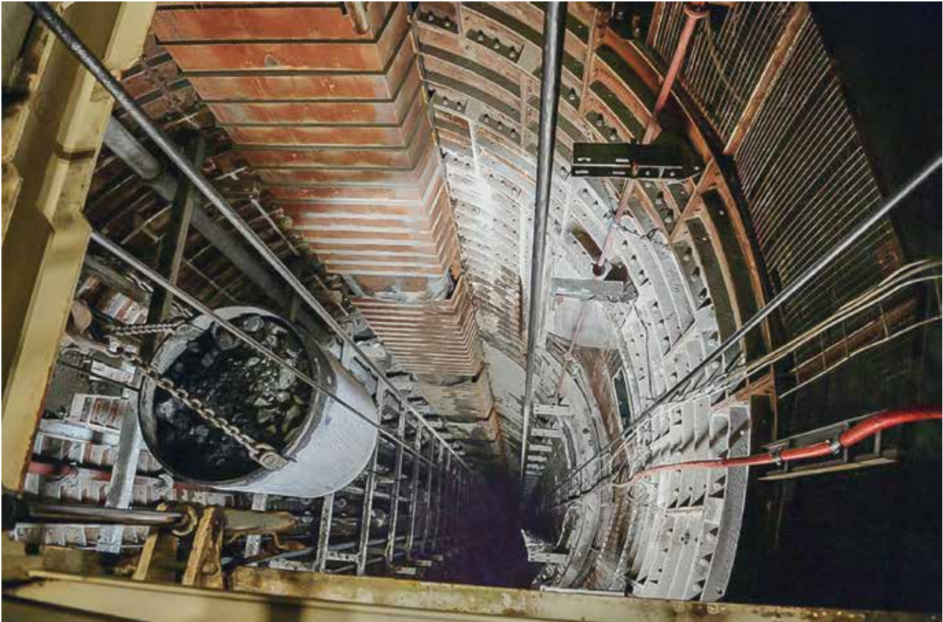
Look into the shaft with its sinking kibble
