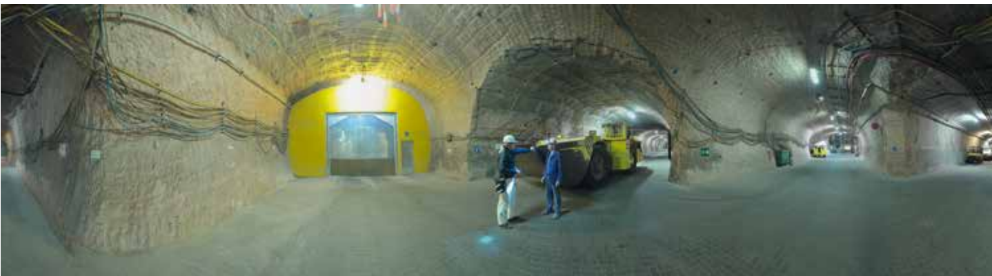
Infrastructure: Roadways at the 840 m-level
