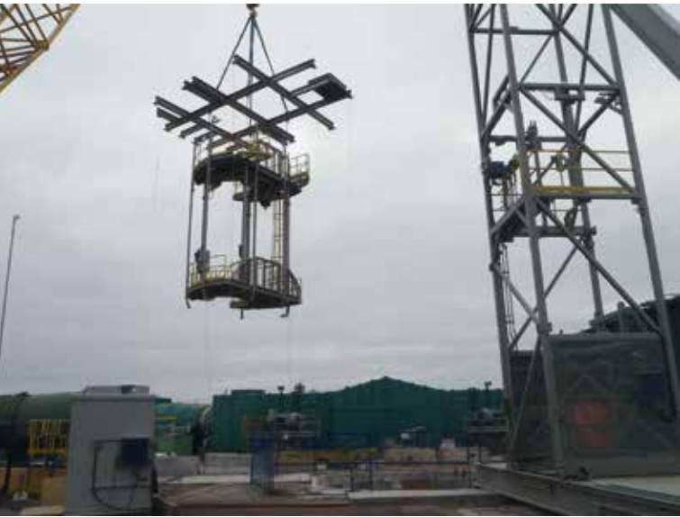
Installation of permanent collar steel and galloway work stage at shaft #2
