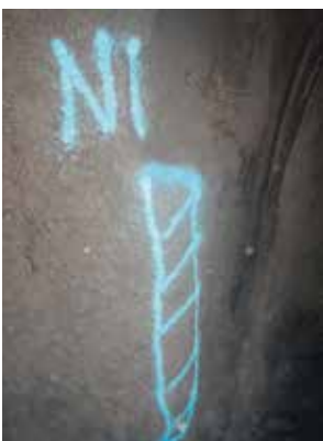
Area of excavation requiring further material removal
