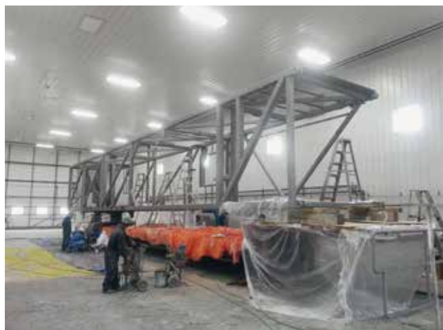
New portable headframe structure at paint shop
