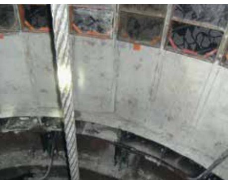
Support ring and 1st concrete block after stripping of the formwork
