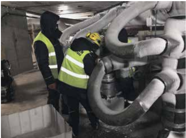
Ice formation at the freeze pipe heads
