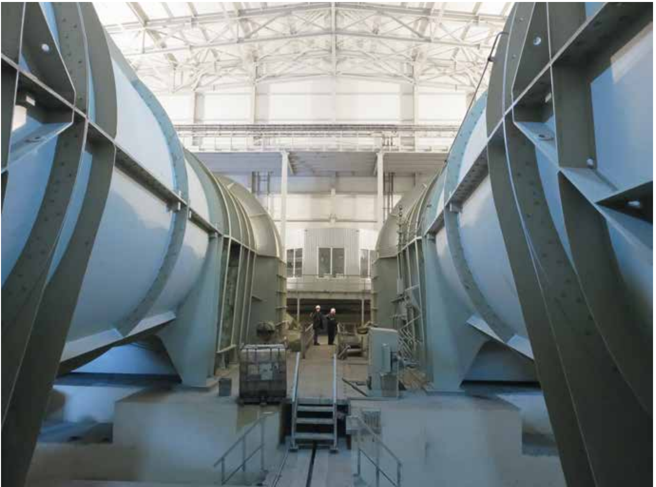
Ventilation system for the underground mine WS-10, Norilsk Nickel
