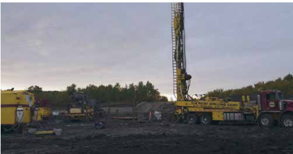
Elk point drill rig setup and ready to drill
