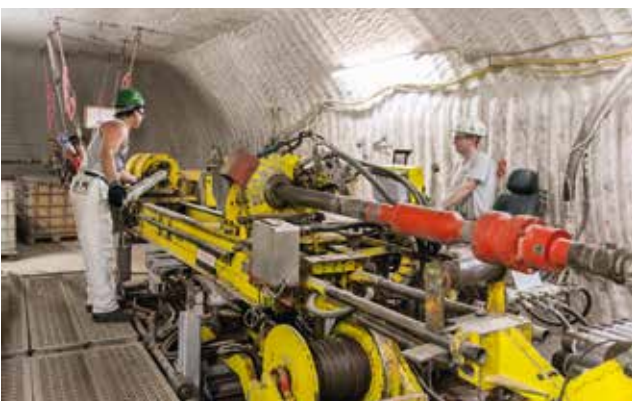
Resetting the drill pipe during drilling operation on the 574 m-level
