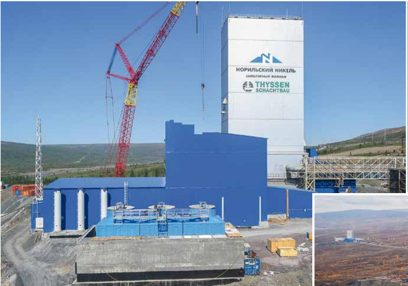
Surface infrastructure at SKS-1 shaft
