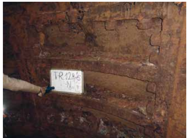
Cast-iron tubbing plate after the cleaning
