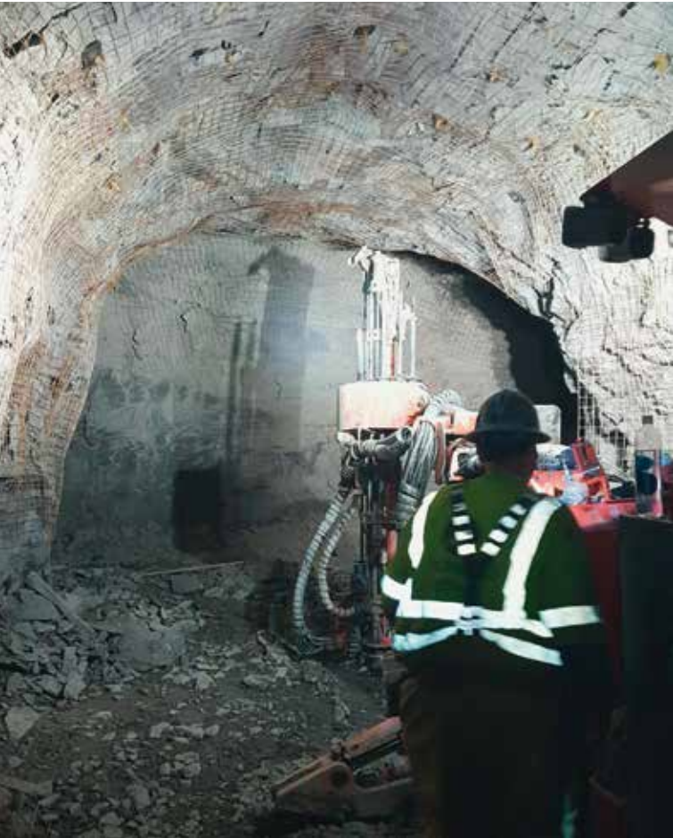
Installing Ground Support
