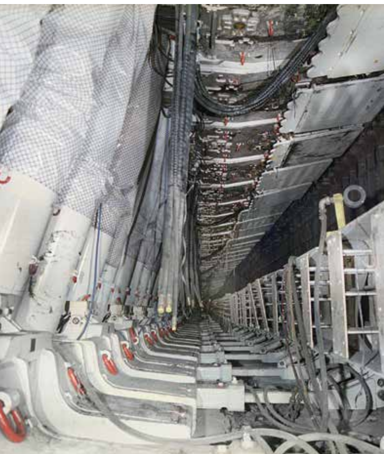
View of fully assembled face installation
