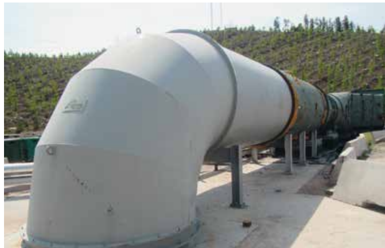
De-mobilization and elbow installation
