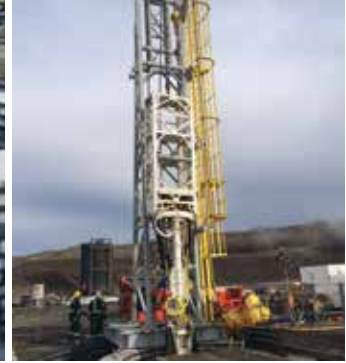
Clam tower structure used during pre-sink
