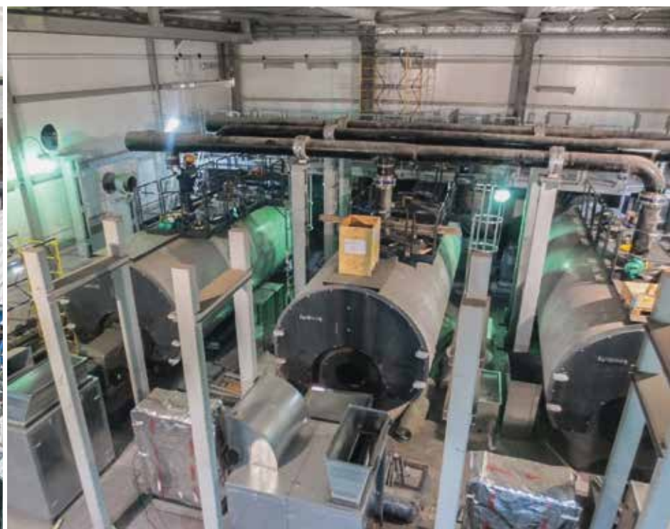
Mine air-conditioning plant
