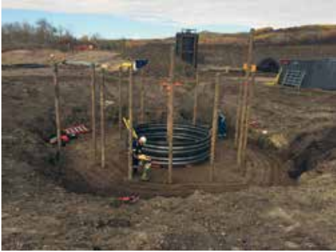
Beginning of the construction for the freeze cellar
