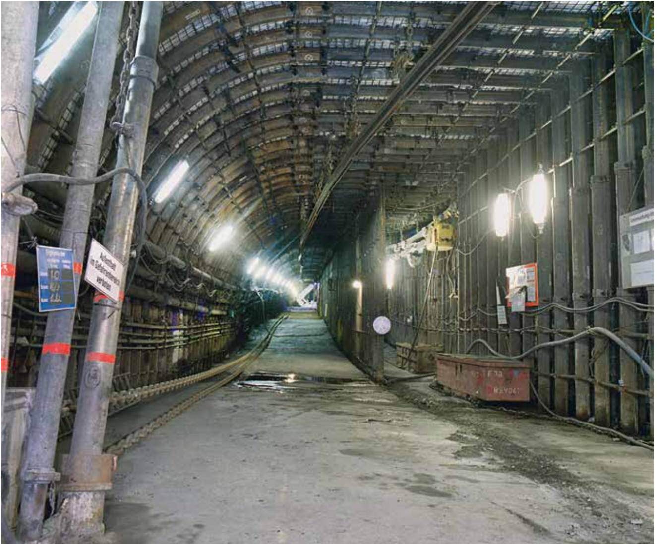
Entry track in the pre-heading has been set up and is ready for manoeuvring the shield units
