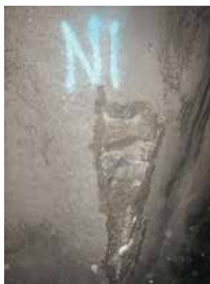
Same area of excavation as above after material removal
