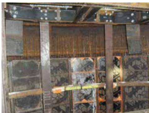
Top level of the system formwork and overlapping reinforcement
