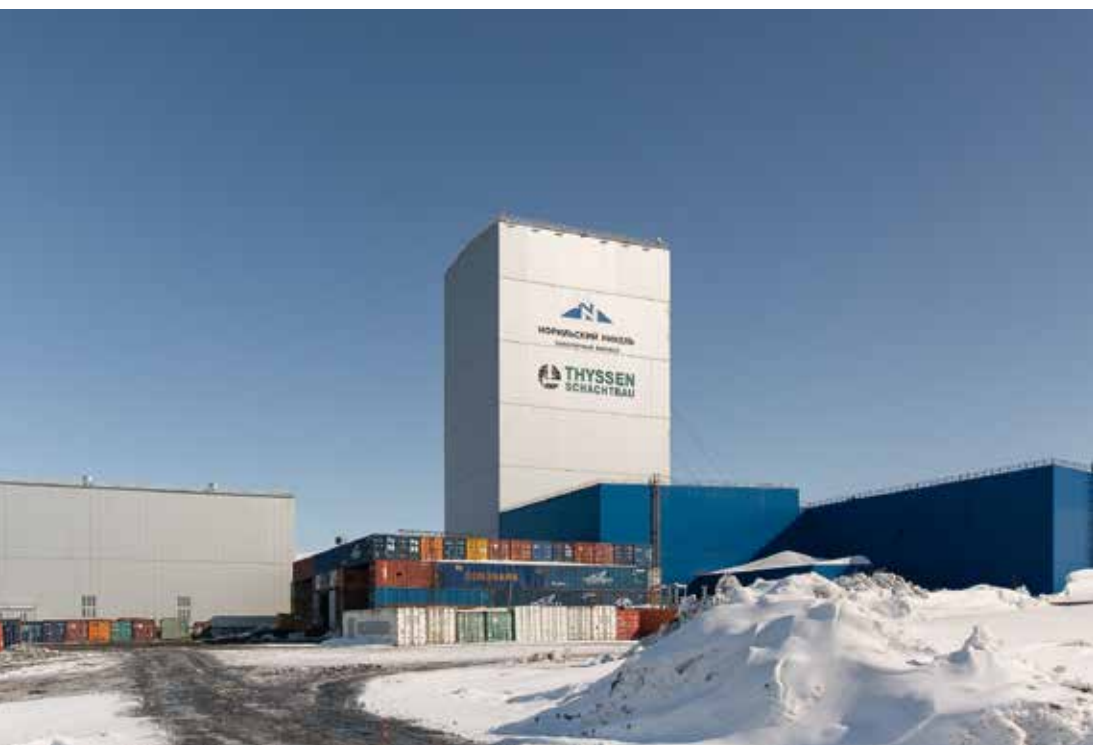
Shaft surface buildings
