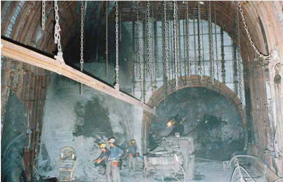
Construction of a roadway junction
