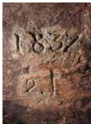
The date and the tunnelshield in the Kaltwasser drift
