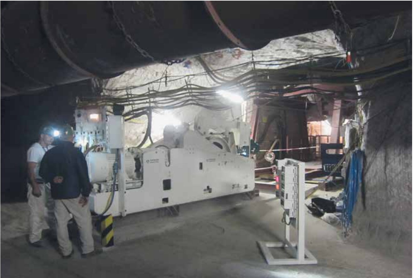
Winching systems at the shaft top
