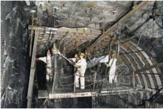
Working platform set up as a pontoon
