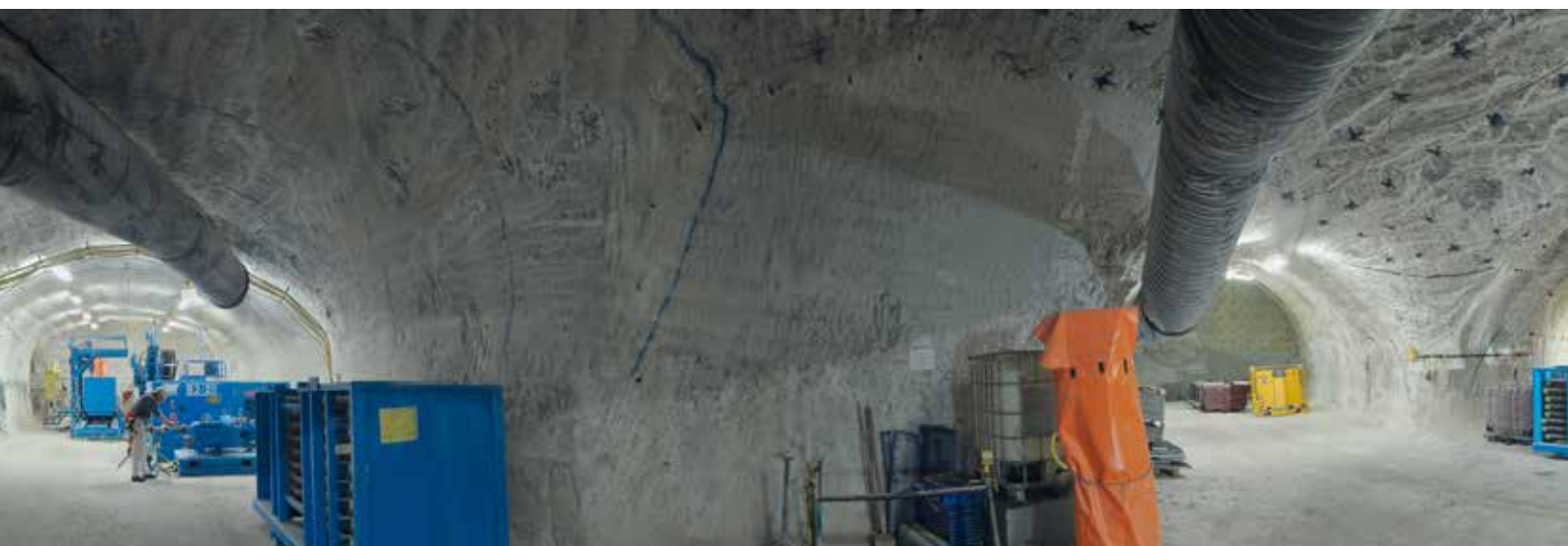
Infrastructure chambers at the 840 m-level
