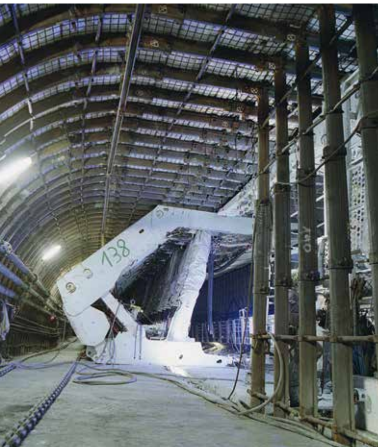
Shield in its final position
