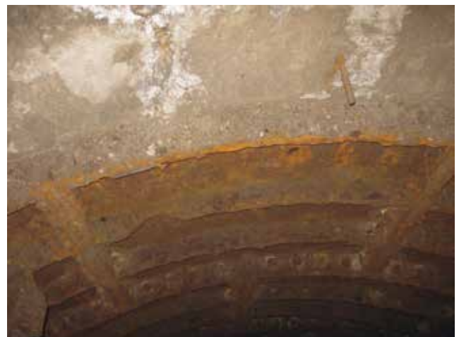
Cast-iron tubbing plate after the cleaning
