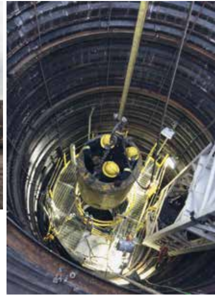
Picture right: Shaft during main sink
