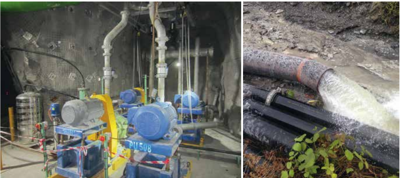
Two line sections with two 8/6 Warman pumps connected in series at the place of installation
