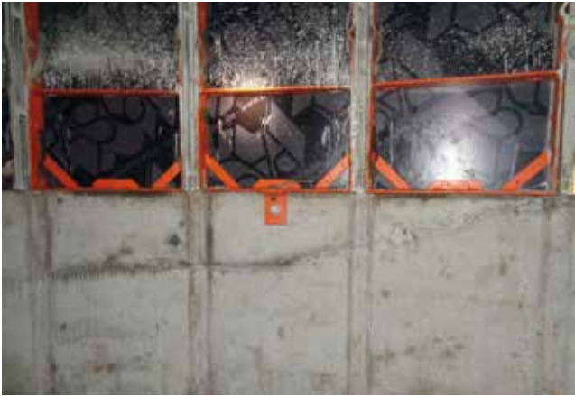
1st concrete block of the support reinforcement shaft 2 after the stripping of the formwork
