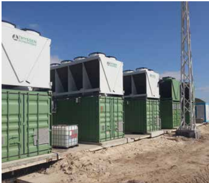
Freeze machine containers
