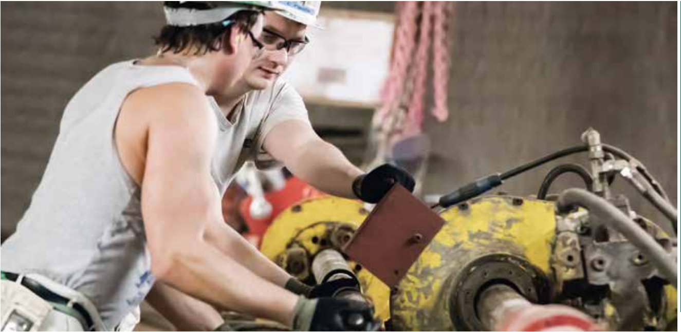
Inserting the inner core barrel into the drill string for water jetting into the depth
