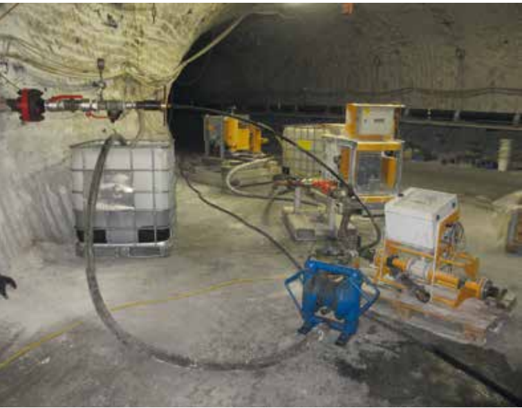
Equipment used for sealing the shallow boreholes
