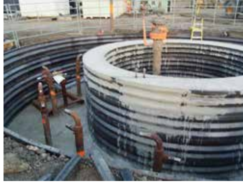
Shaft collar foundation and freeze cellar
