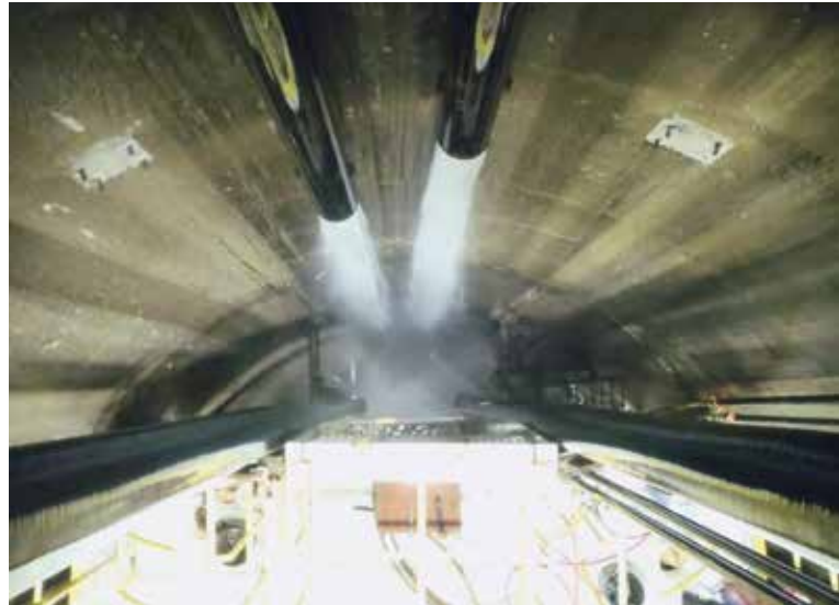
View from galloway – water capture system near shaft bottom
