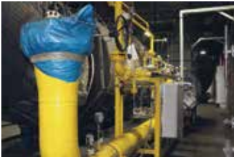
Control station with gas connection
