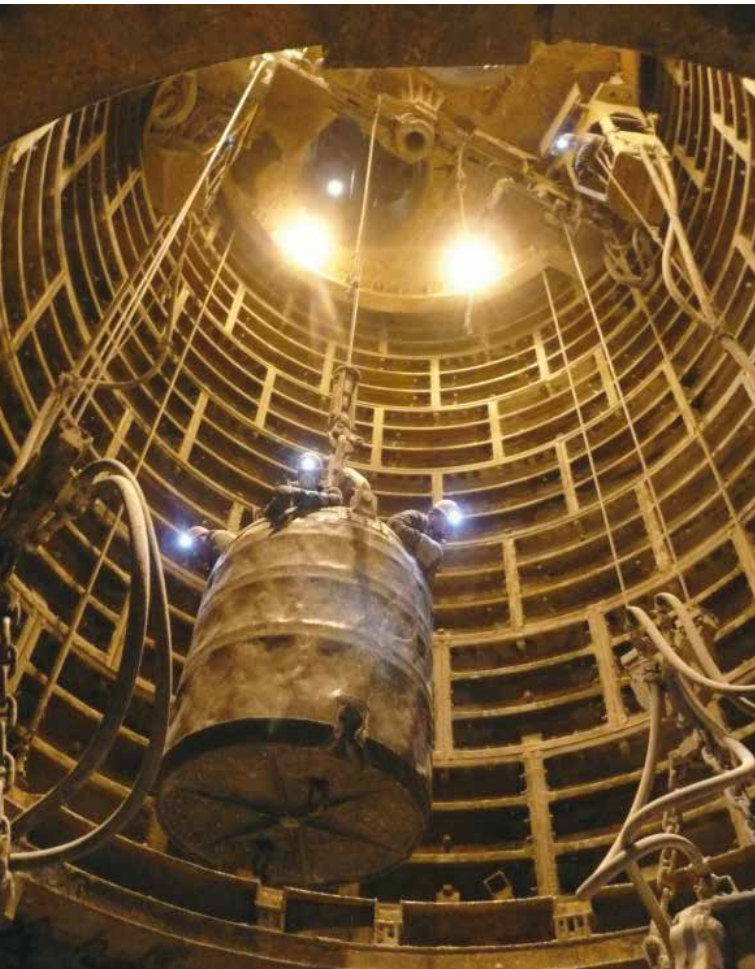
View from the tubbing shaft bottom to the sinking stage
