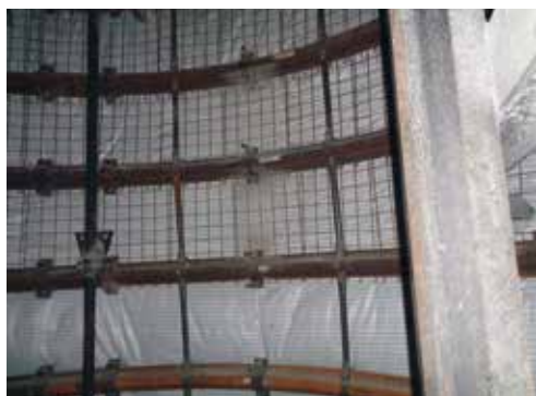
Steel ring support Shaft Borth 1
