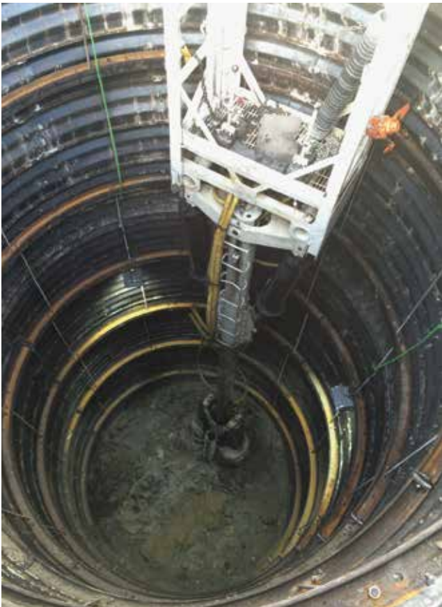
Shaft during the pre-sink phasis
