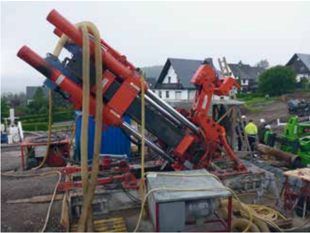
Inclined bored connection with raisebore machine Rhino 2007 DC to connect the Kaltwasser with the Commun drift
