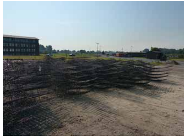
Reinforcement cages at the side for the construction of the support reinforcement
