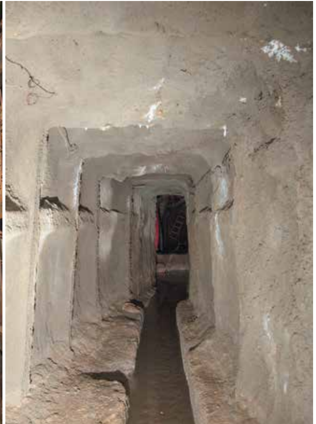
Steel support and shotcrete secured with crosscut in the pumping shaft
