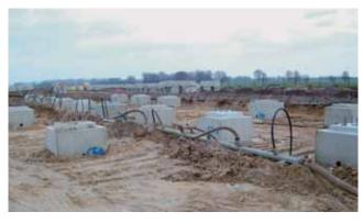
P. 74: Floating-in the needle filters for groundwater lowering with steel portals for receiving the transformers
