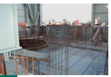
Some 2,800 m<sup>3</sup> concrete installation preparation work for the shaft cellar in parallel to the final headframe installation
