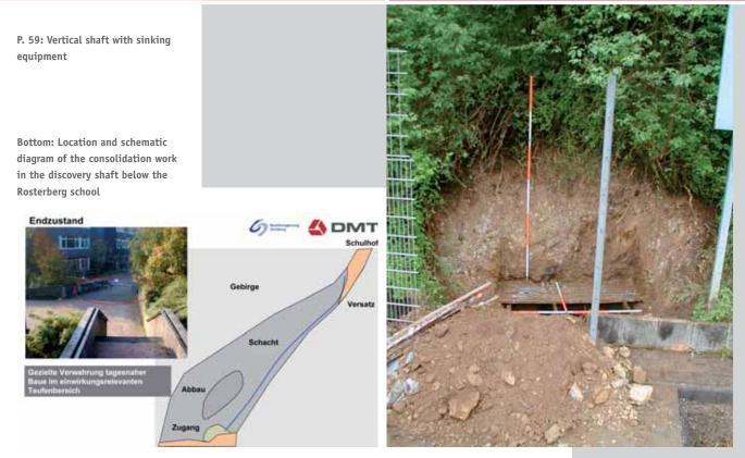
provide an abutment for the subsequent filling operation, the rest of the cavity was completely filled in. A total of some 150 m<sup>3</sup> of hydraulic setting mixture was pumped by pipeline into the open shaft and old workings leading from it. None of the suspension escaped into others parts of the mine.
