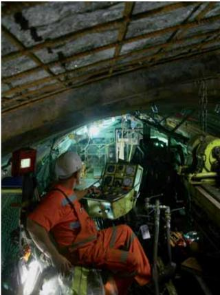
Preliminary drilling was carried out during the drivage phase for better geological reconnaissance and in order to verify, confirm and/or modify the existing prognoses. Thanks to recent advances in drilling and strata-injection technologies tunnelling engineers now have access to preliminary exploration and strata reinforcement tools that can be employed effectively as the drivage advances.
