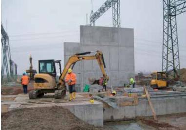
Top: Sheet piling for the largescale oil separator Middle: Foundation for transformer and fire walls
