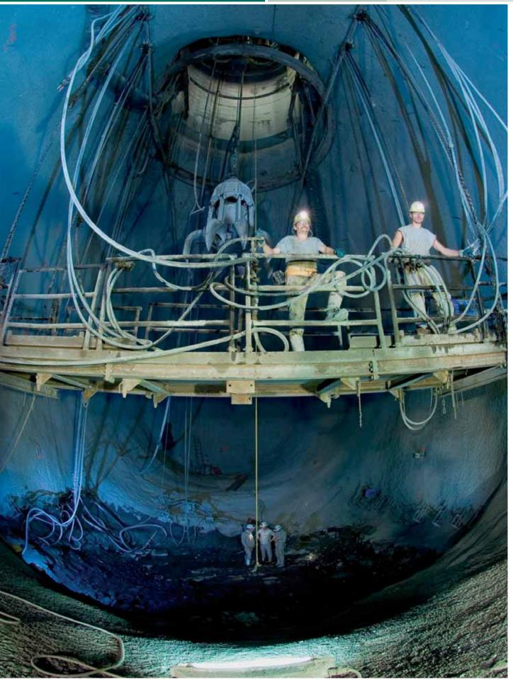
Shaft inset on mine level 7, steel-fibre shotcrete lining with systematic rockbolting
