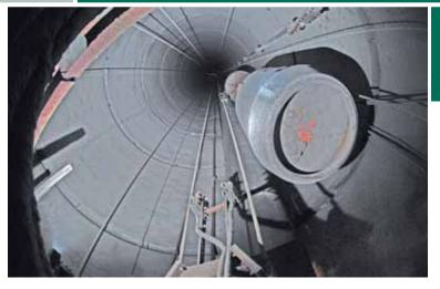
The decision to extend the much-used materials and manwinding shaft no. 10 at RAG's Prosper-Haniel colliery posed a particular challenge to the sinking team, especially as there was to be no interruption to the normal winding operations. The deeper shaft will play a crucial role in developing new panels containing some 120 mill. t of high-quality steam coal.
