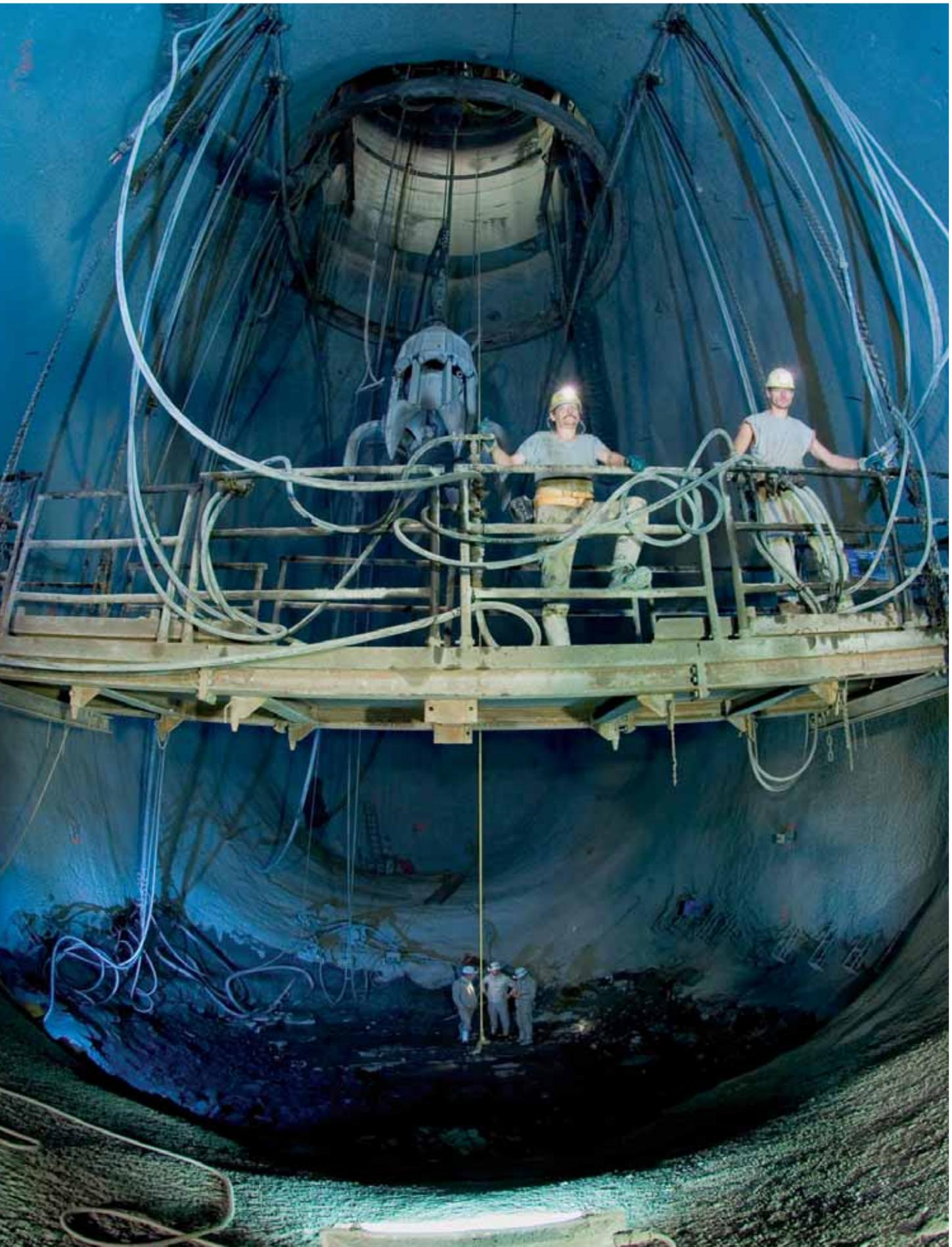
Shaft inset on mine level 7, steel-fibre shotcrete lining with systematic rockbolting
