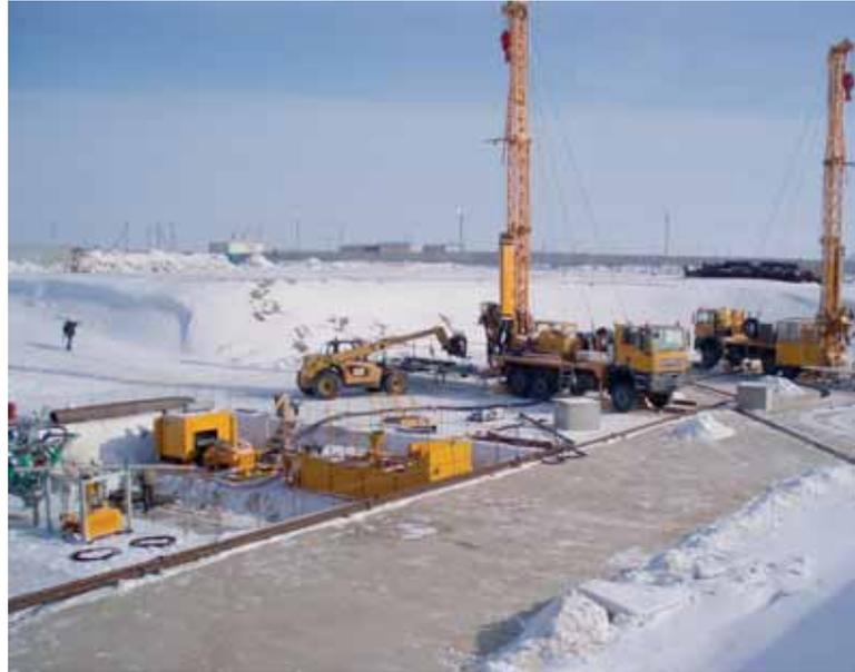
RB 50 rig being assembled prior to drilling the freeze holes in February 2009
