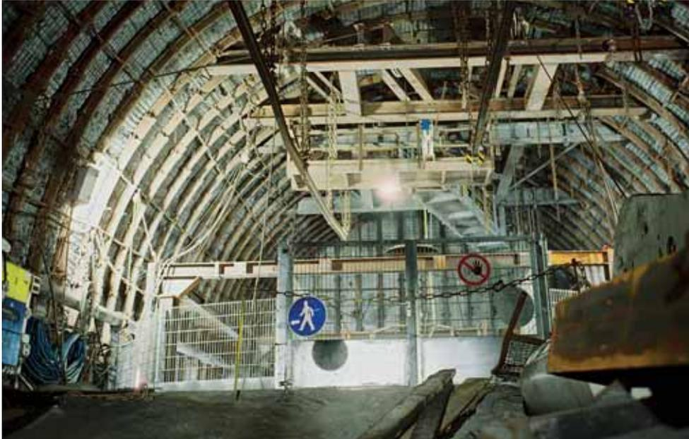
Sinking equipment at the head of the bunker with pulley frame, kibble winch and fall protection
