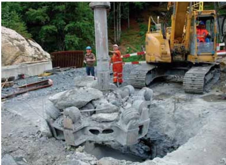
Top: The drift reaches the pilot hole and the drill bit can now be swapped over for the cutterhead
