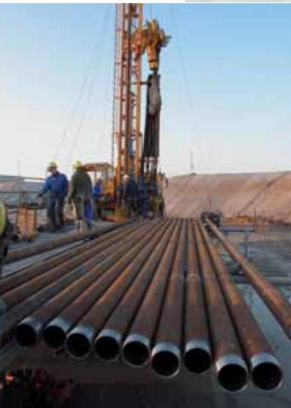
RB 50 drilling rig during freeze-pipe installation
