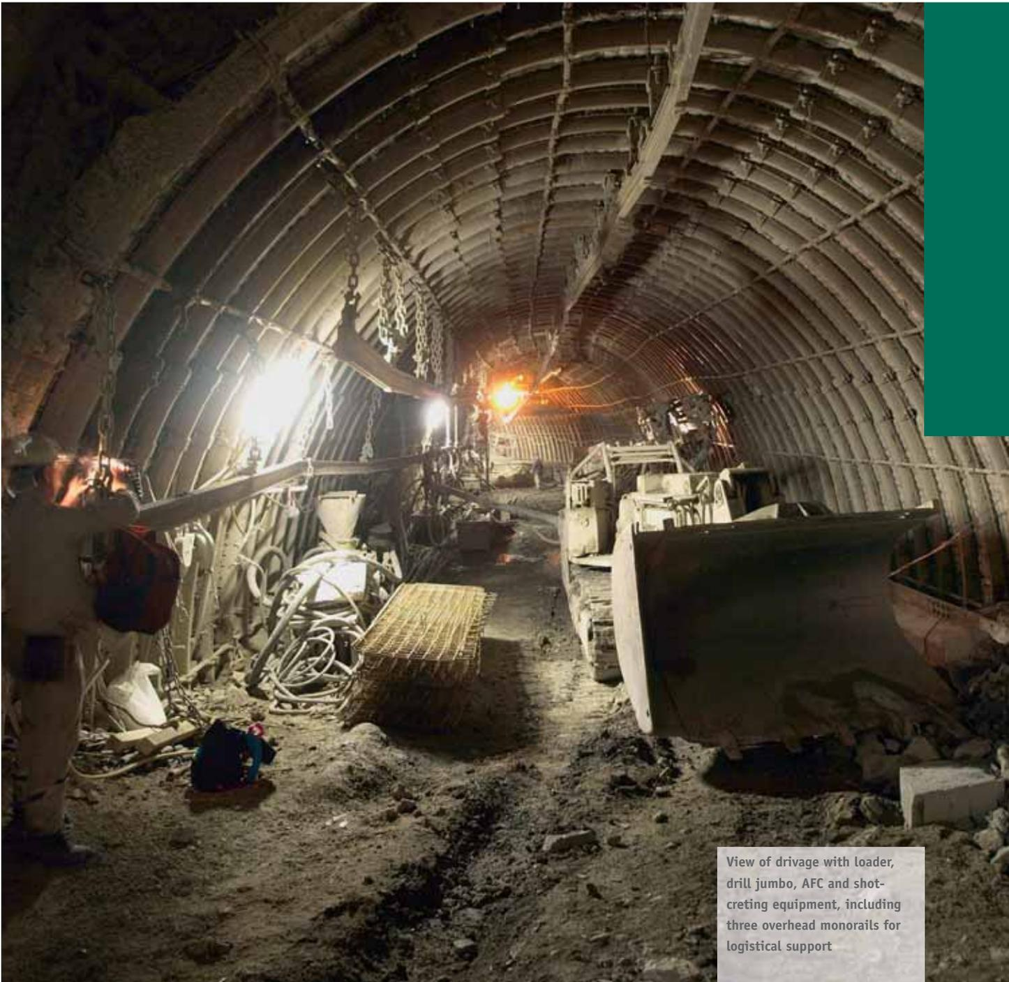
View of drivage with loader, drill jumbo, AFC and shot-creting equipment, including three overhead monorails for logistical support
