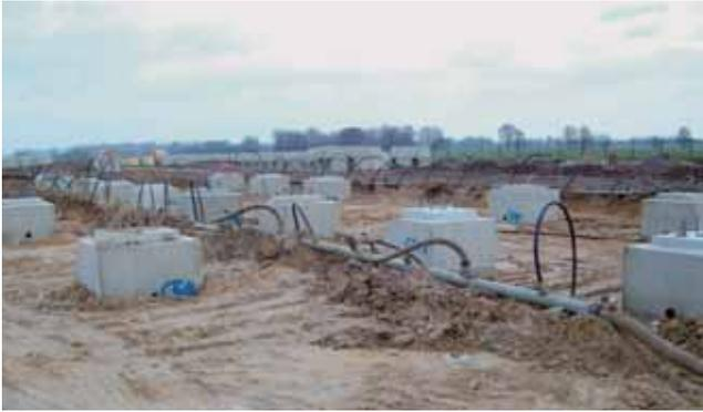
P. 74: Floating-in the needle filters for groundwater lowering with steel portals for receiving the transformers
