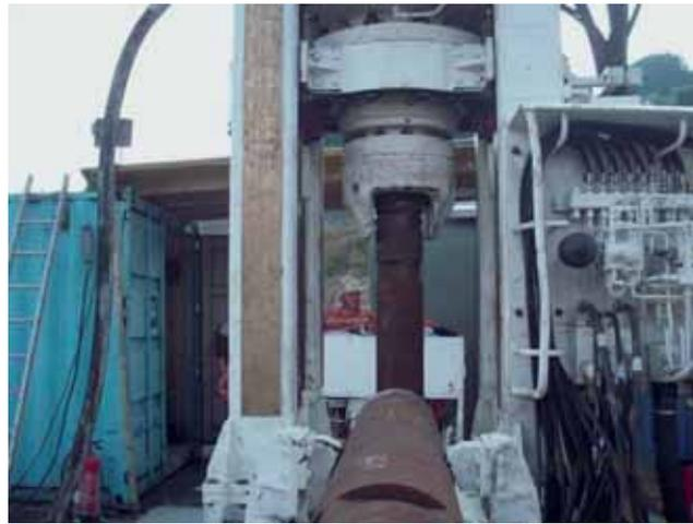
Right: Breakthrough for the pilot hole, reaming head fitted
