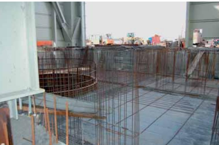
Some 2,800 m<sup>3</sup> concrete installation preparation work for the shaft cellar in parallel to the final headframe installation
