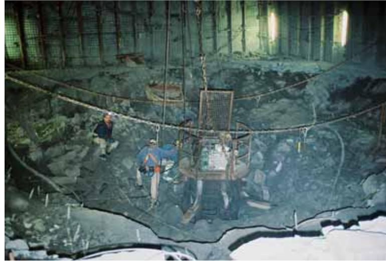
Sinking equipment with borehole fence and slusher system
