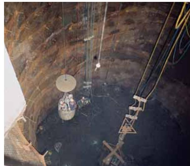
Top: Sinking operation with borehole fence, slusher system and transport kibble
