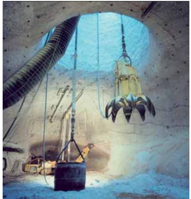
Inset for the exploration level, excavated by drilling and firing, profiling with cutting head
