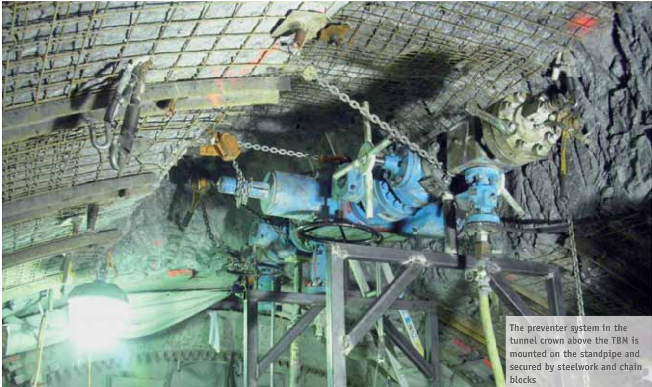
The preventer system in the tunnel crown above the TBM is mounted on the standpipe and secured by steelwork and chain blocks
