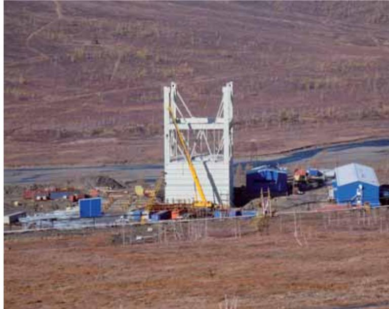
The shaft facility in September 2009; left to right: Basestructure of the 110 kV power station, 45 m of final 66 m of permanent headframe, 6 kV station, temporary ventilation building, temporary social building
