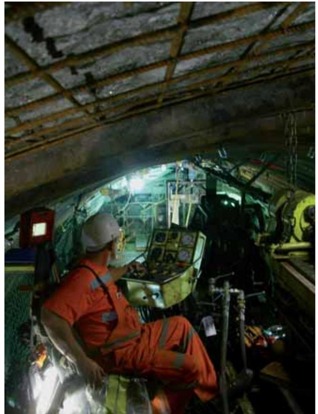
Preliminary drilling was carried out during the drive phase for better geological reconnaissance and in order to verify, confirm and/or modify the existing prognoses. Thanks to recent advances in drilling and strata-injection technologies tunnelling engineers now have access to preliminary exploration and strata reinforcement tools that can be employed effectively as the drive advances.
