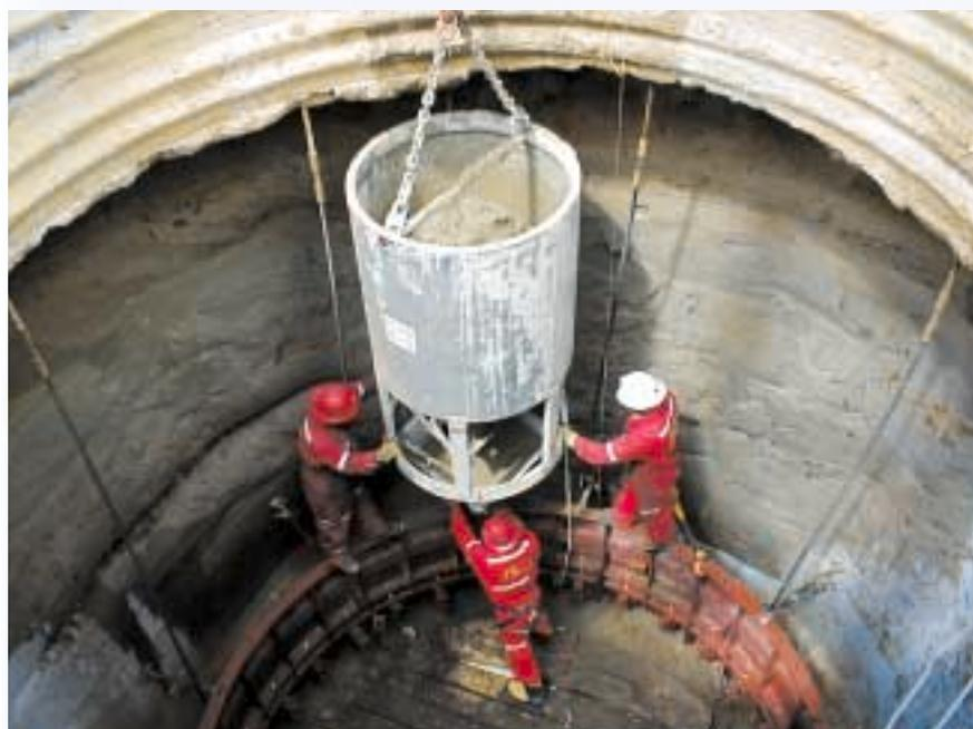
to the face after each round. Seams of mud and altered kimberlite were encountered which caused us to change our drilling and blasting pattern in an effort to reduce overbreak.
