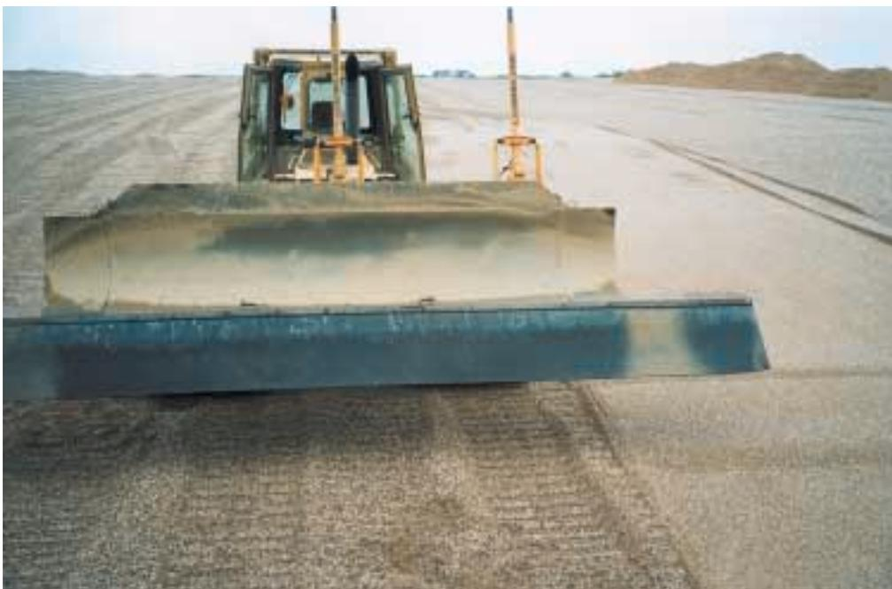
If any surface imperfection is detected the entire layer must be removed and the operation has to begin all over again. As this is a very expensive process, high-quality execution has to be the order of the day. To date some 18,000 m<sup>2</sup> of the total surface area of five hectares have already been completed without a flaw.
