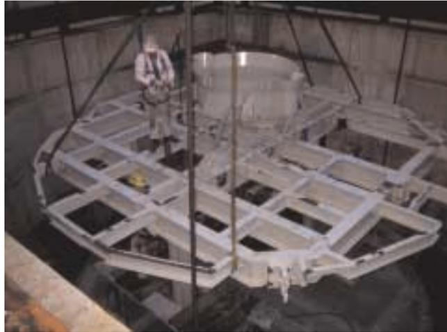
Picture left: Assembling the overhead protection with intake gate for the mini manwinder on the single-deck working platform at the mouth of the shaft
