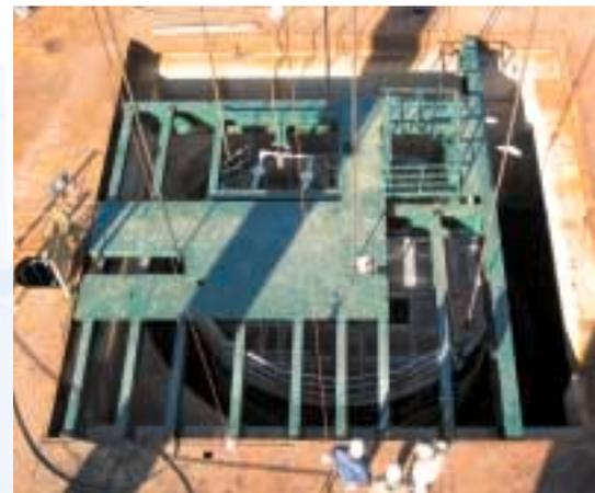
Installing the new shaft cover from the protective roof of the single-deck platform
