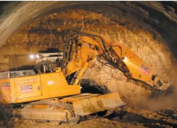
Tunnel excavator clearing the heading face (friable dolomite from the Upper Muschelkalk Series)
