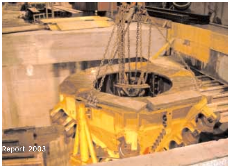
Installation of shaft boring machine
