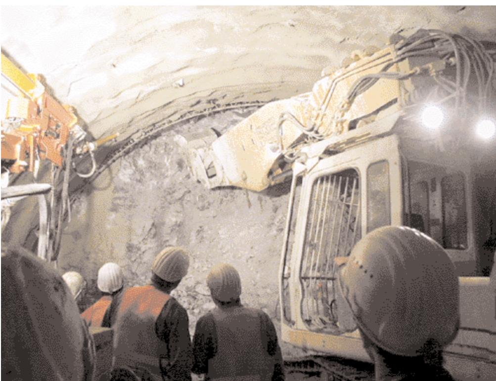
Excavator and shotcrete manipulator at the heading face
