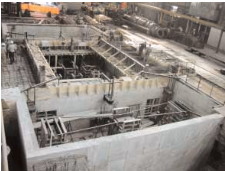
High-tech formwork systems for erecting bracket points and walls
