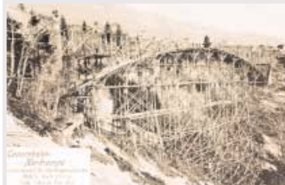
Bridge scaffolding over the Anger gorge
