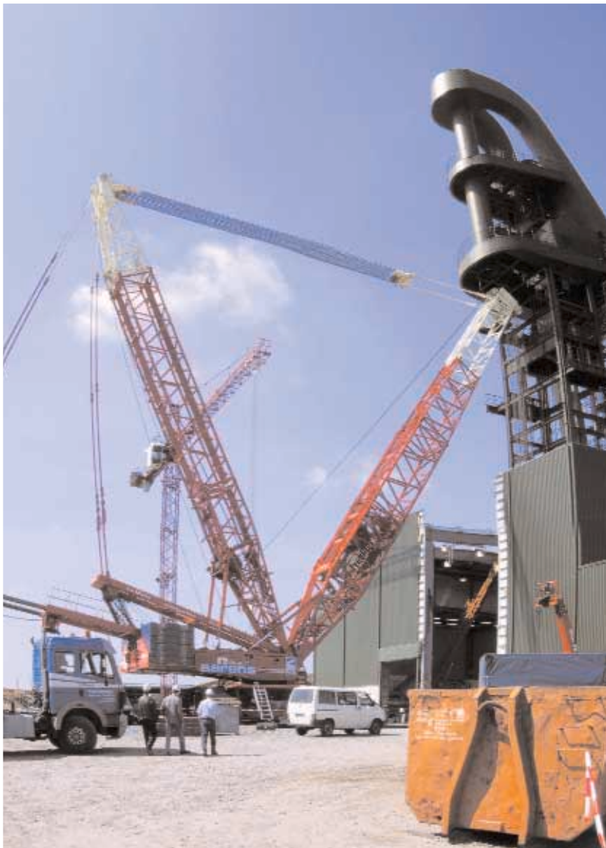
1,200-t-crane in action
