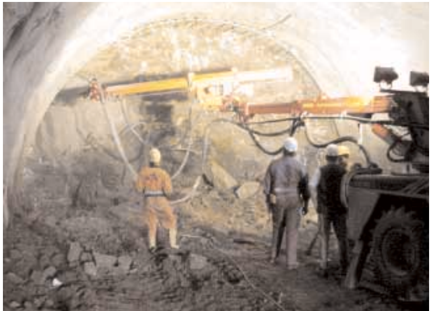
Sealing work at the heading face
