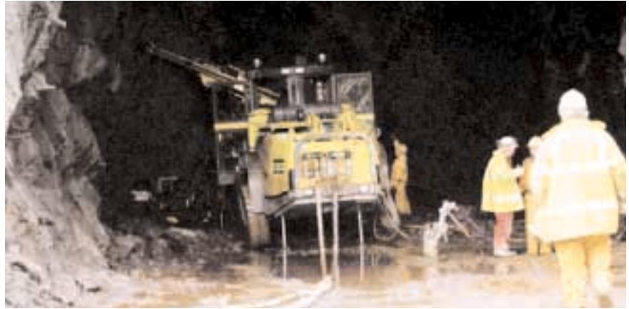
Tunnel Portal with Atlas Copco L2C Drilling Jumbo.
