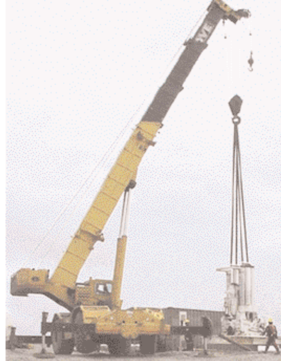
RBM7SPLH Raise Borer at EKATI Diamond Mine (August, 2002)
