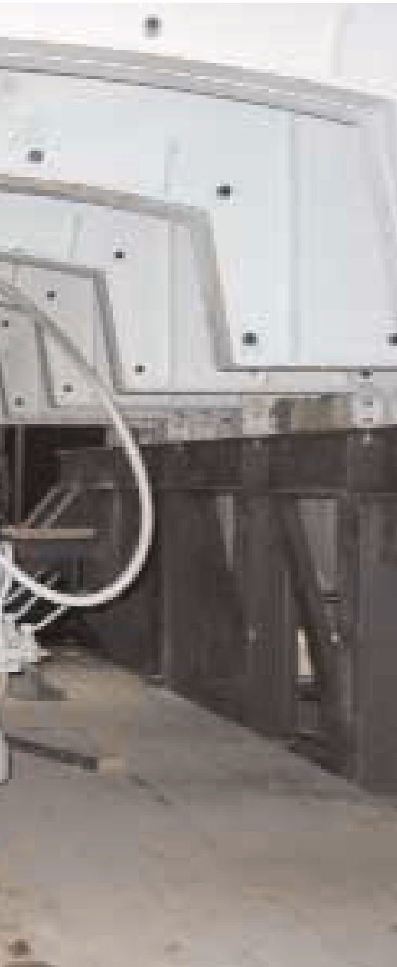
Formwork car with up-front reinforcement car in the pre-cut assembly chamber
