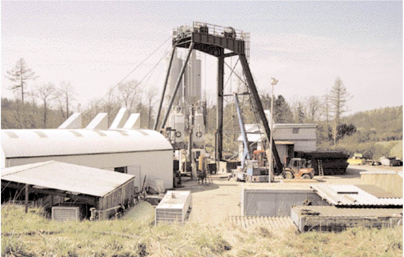
Sinking frame and surface installations
