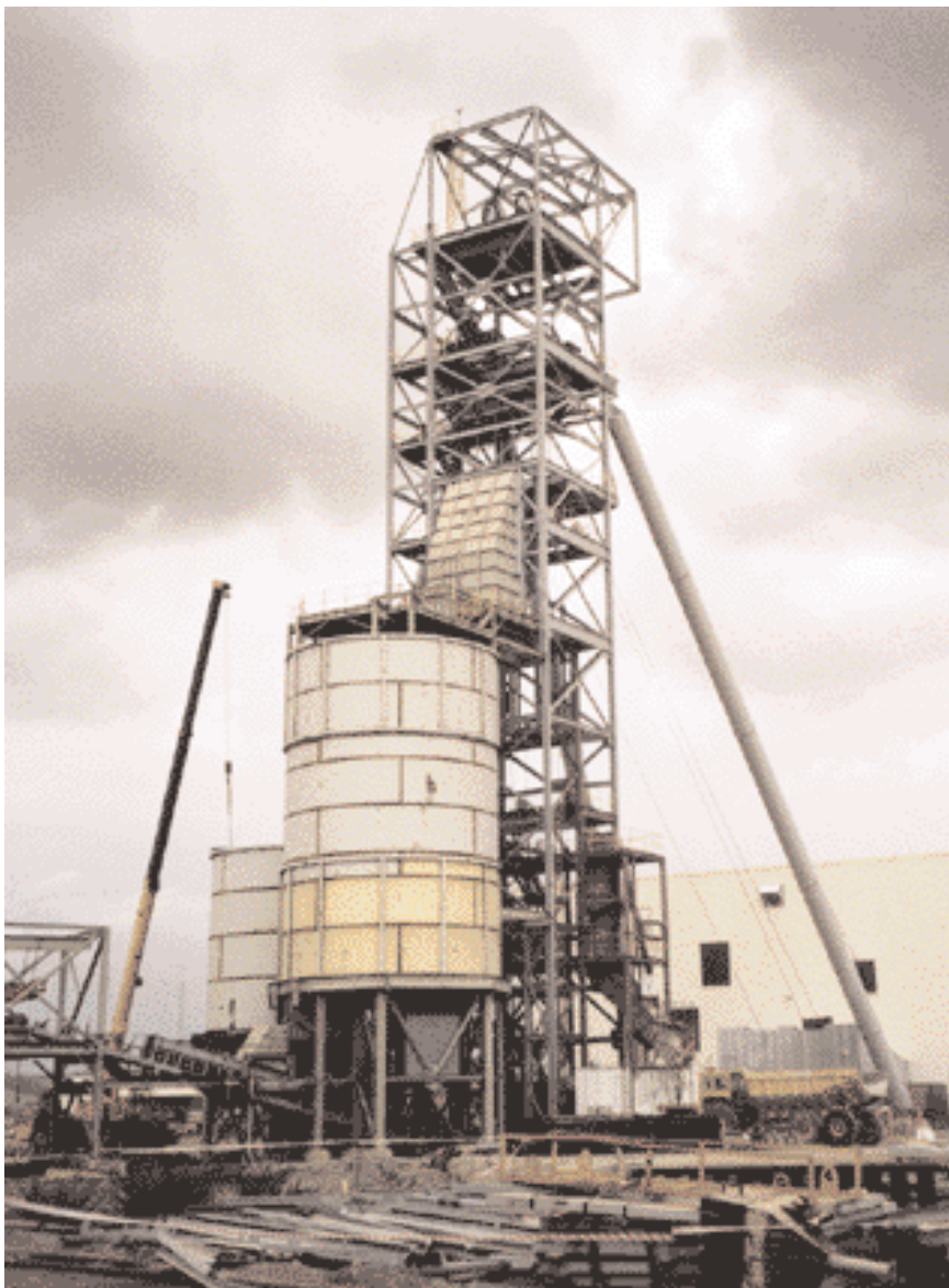
Shaft headframe with ore bunker
