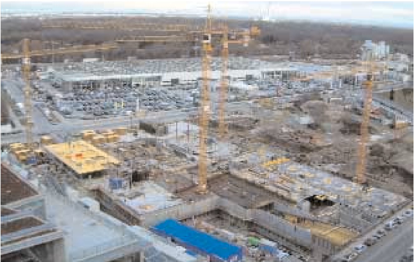
View of the construction site
