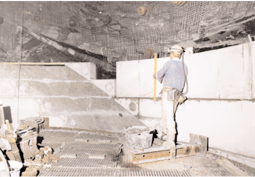
Installing the precast segments
