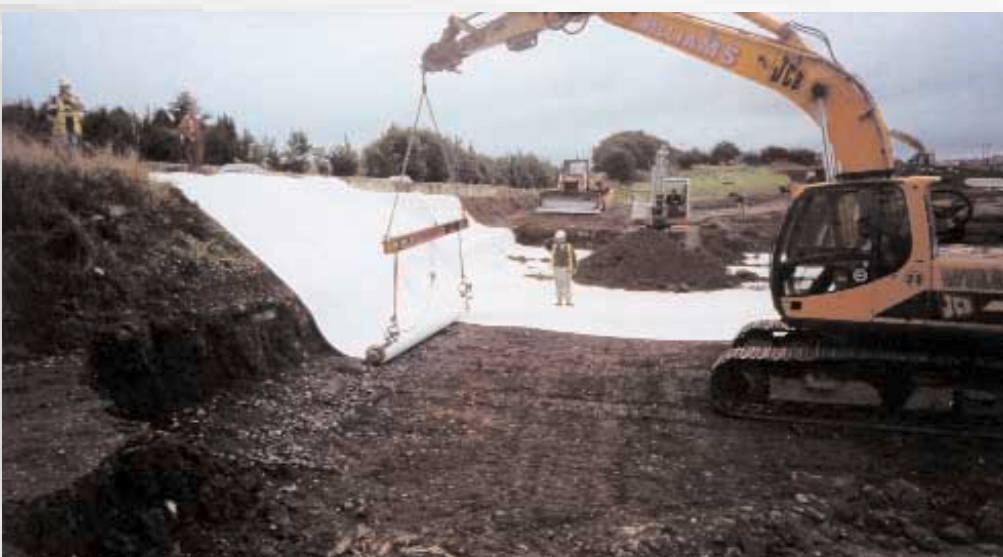
Placing geotextile reinforcement in the peat-bog area
