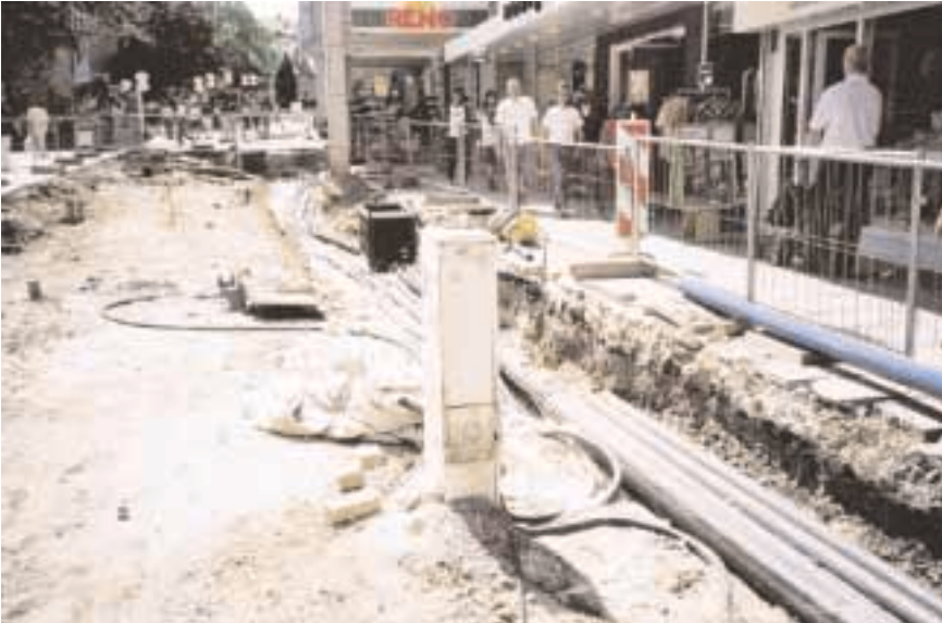
Segregated construction zones ...
