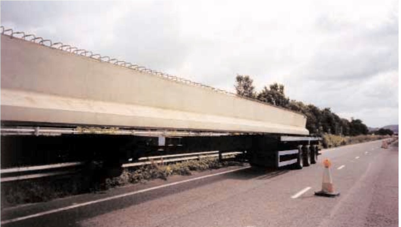
Main bridge girder being delivered
