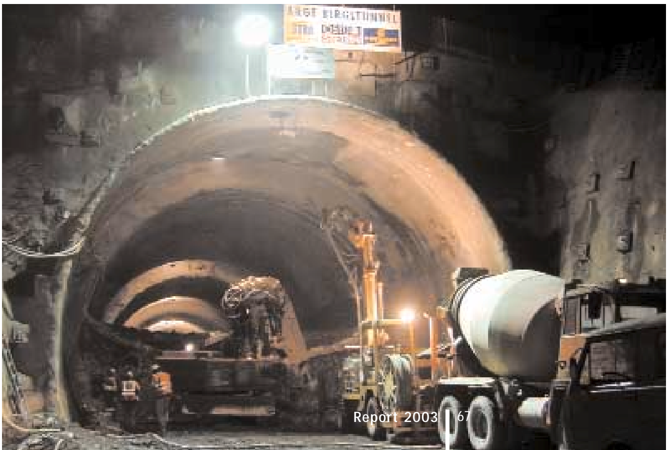
Bench drive in the west-portal area of the Birgl tunnel
