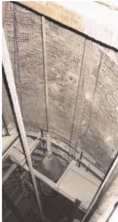
Manwinning shaft and alighting platform beneath Borth No. 1 shaft decking level
