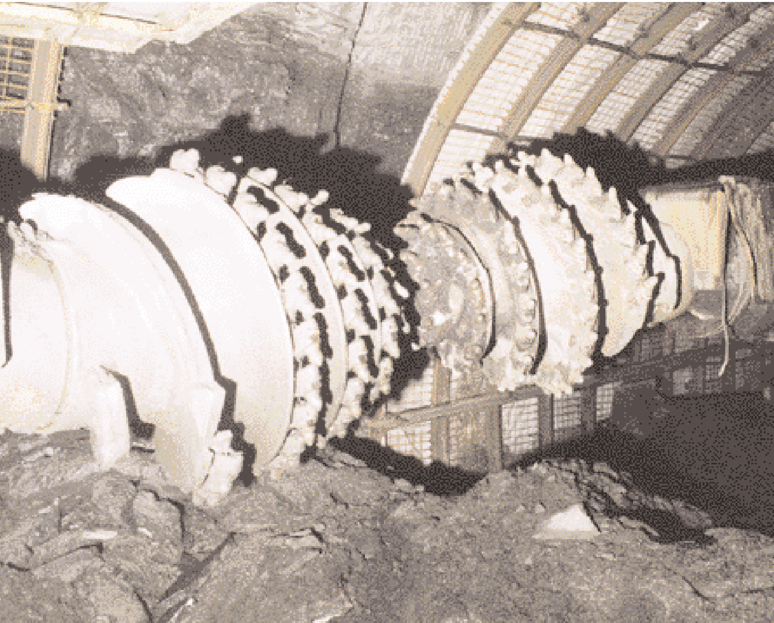
Roadheader drivages meet up
