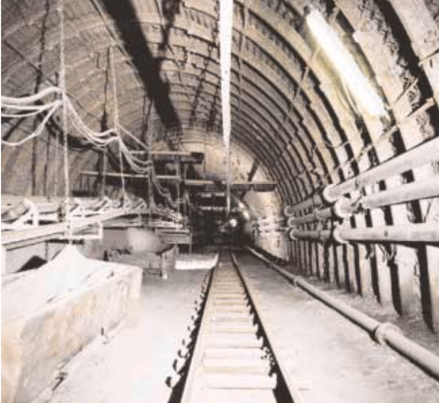
View of completed roadway
