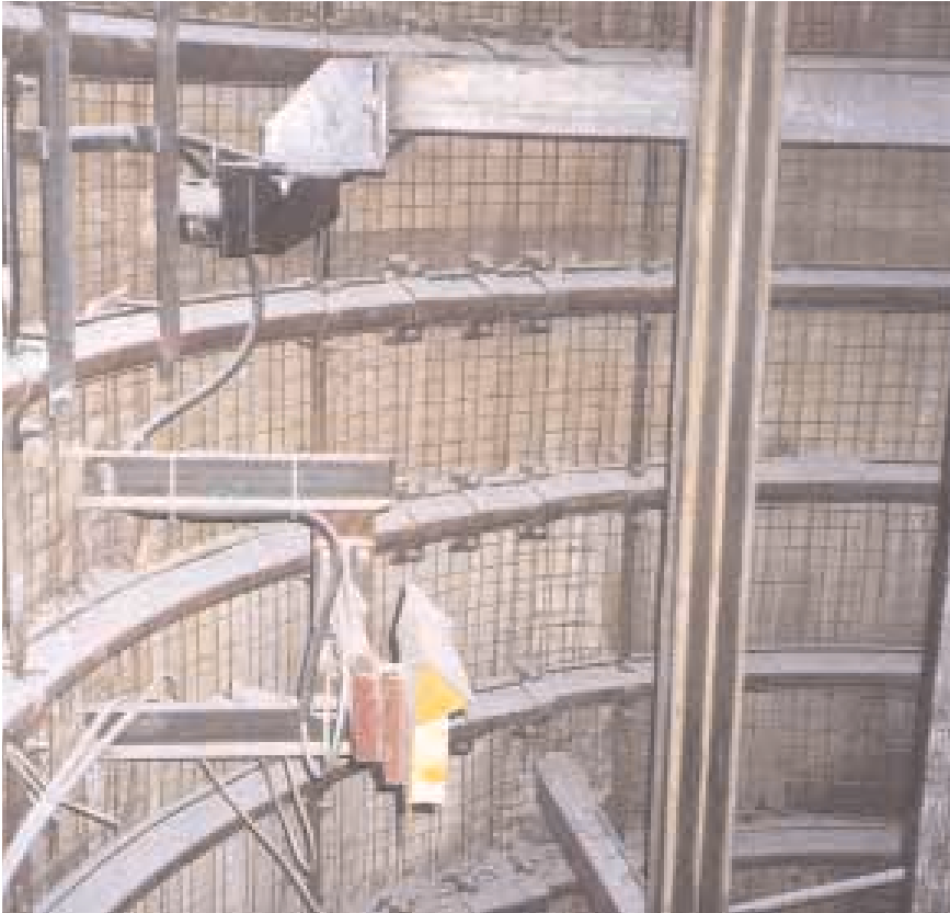
Steel support rings in Borth No. 2 shaft
