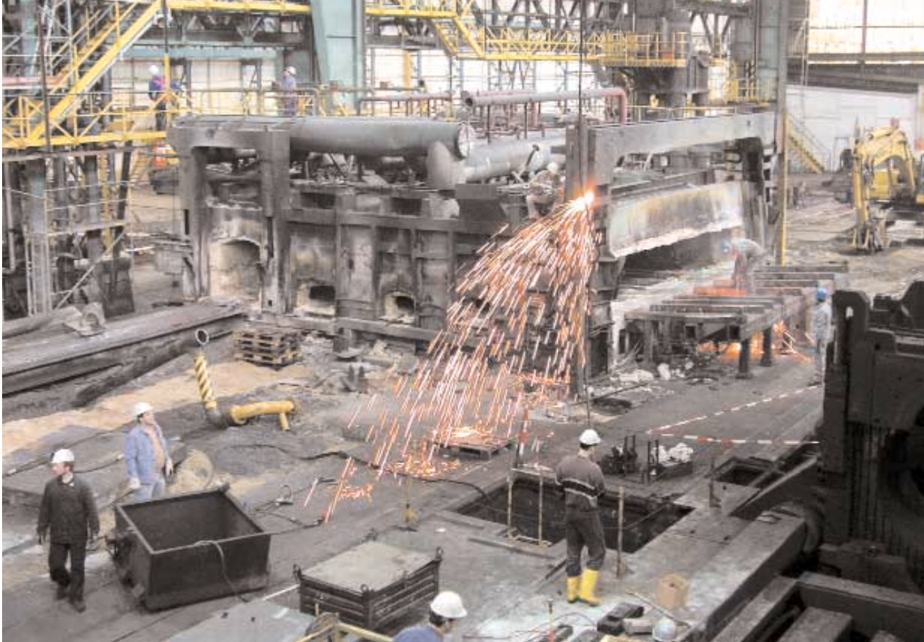
Dismantling the old roller furnace
