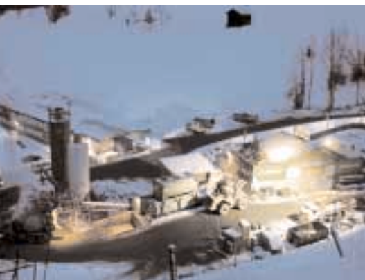
Site equipping stage
