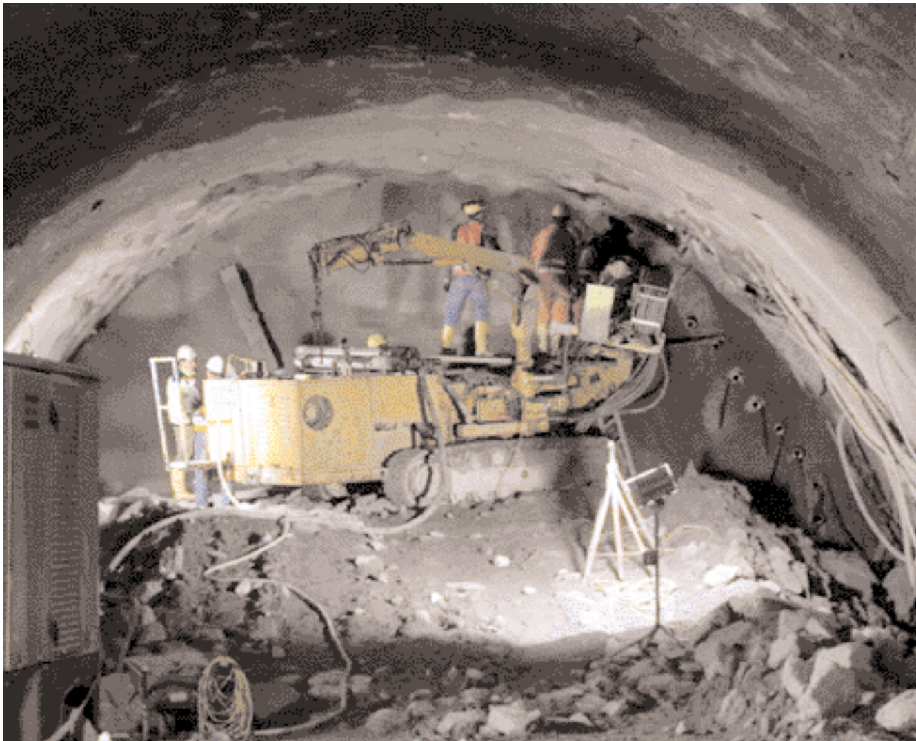
Erecting a tunnel screen pipe
