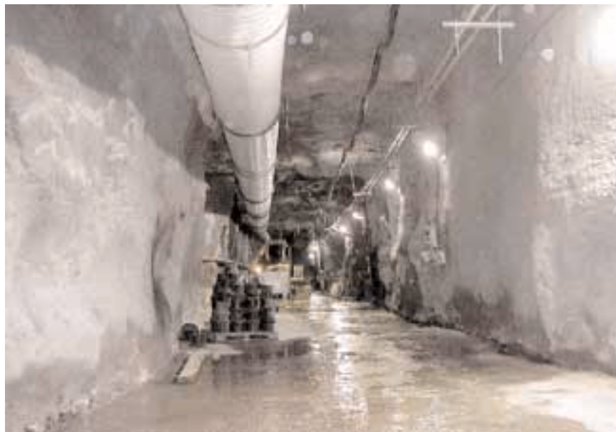
Typical haulage road (with full shotcrete lining and concreted floor)
