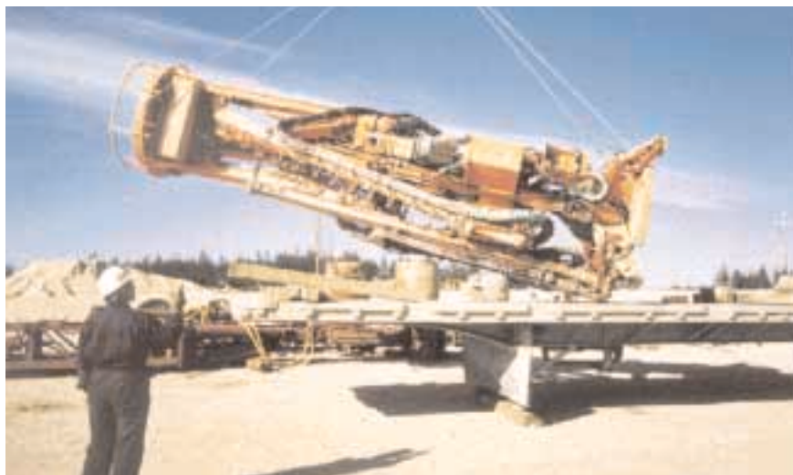
Deployment of a shaft drilling jumbo
