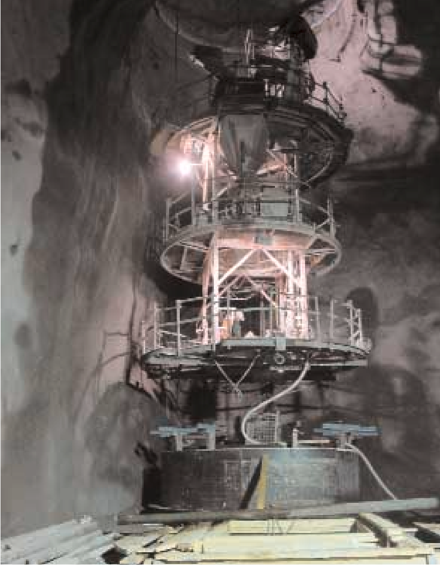
Sliding scaffold with multi-deck sinking platform
