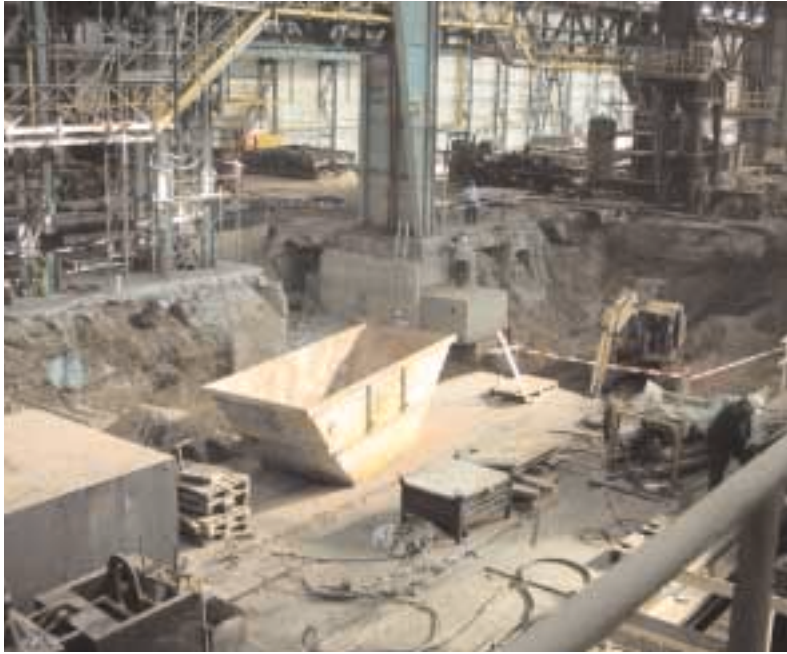
Not much room for the excavators
