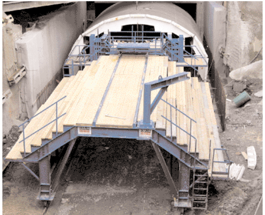
Formwork car with up-front reinforcement car in the pre-cut assembly chamber
