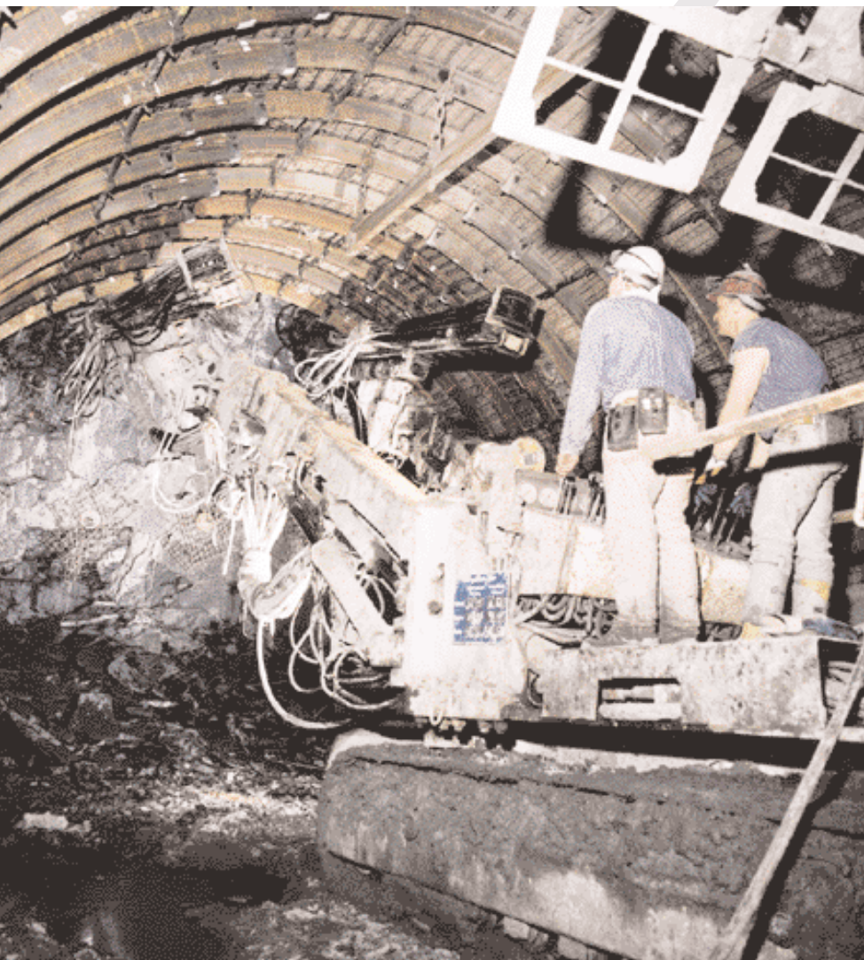
Twin-boom drill jumbo in action
