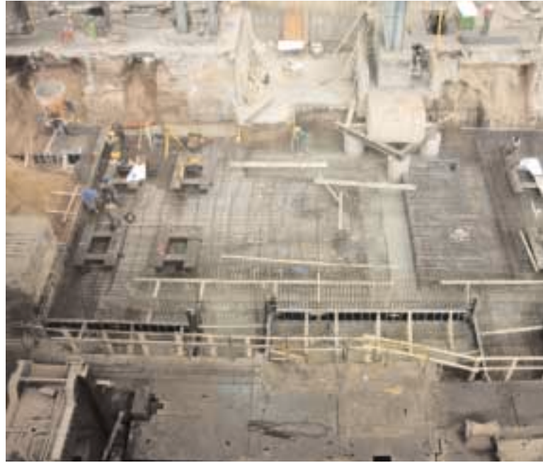
Securing the foundations and arming the bed-plate
