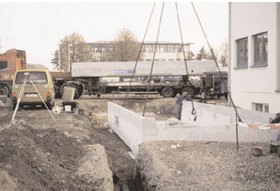
Erecting the vehicle weighbridge
