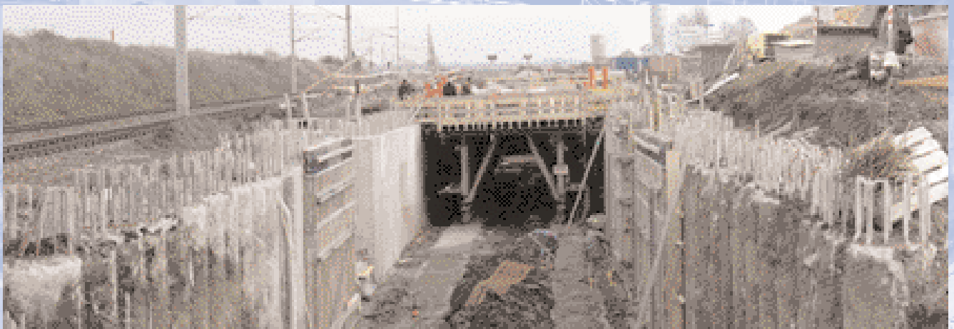
Östu-Stettin formwork car in operation
