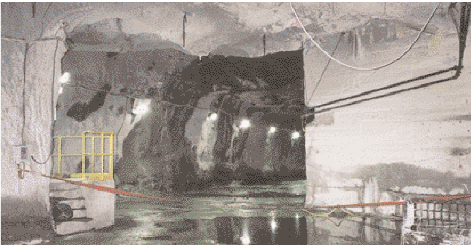
Haulage road on 640-metre level close to filled roadway
