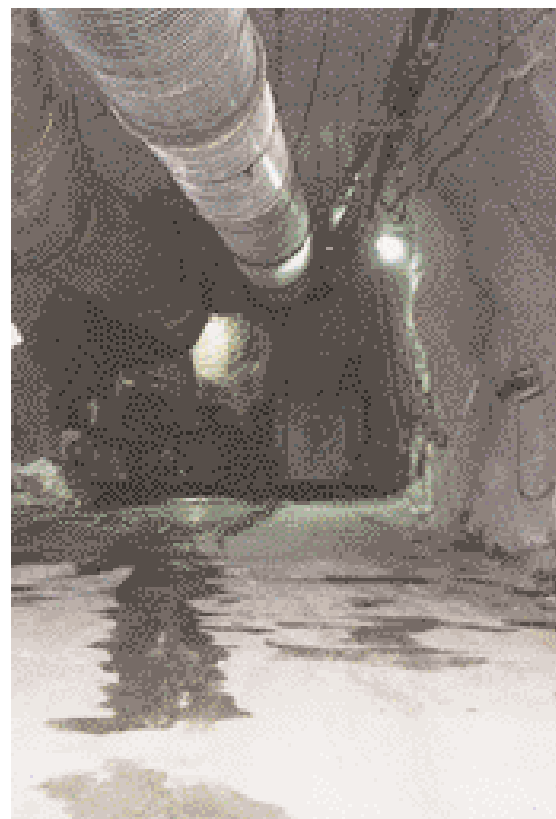
Access ramp to raisebore drill chambers with shotcrete fillings and concrete floor
