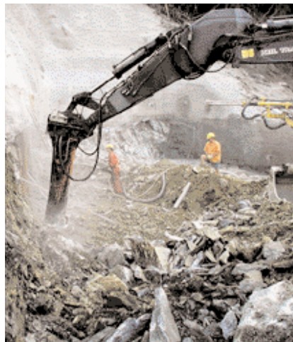
Preliminary trenchwork at Maiskogel
