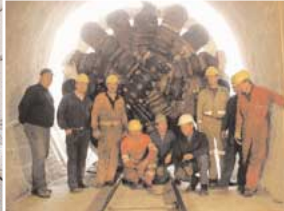
Photo bottom: Boring head ready assembled with drill crew
