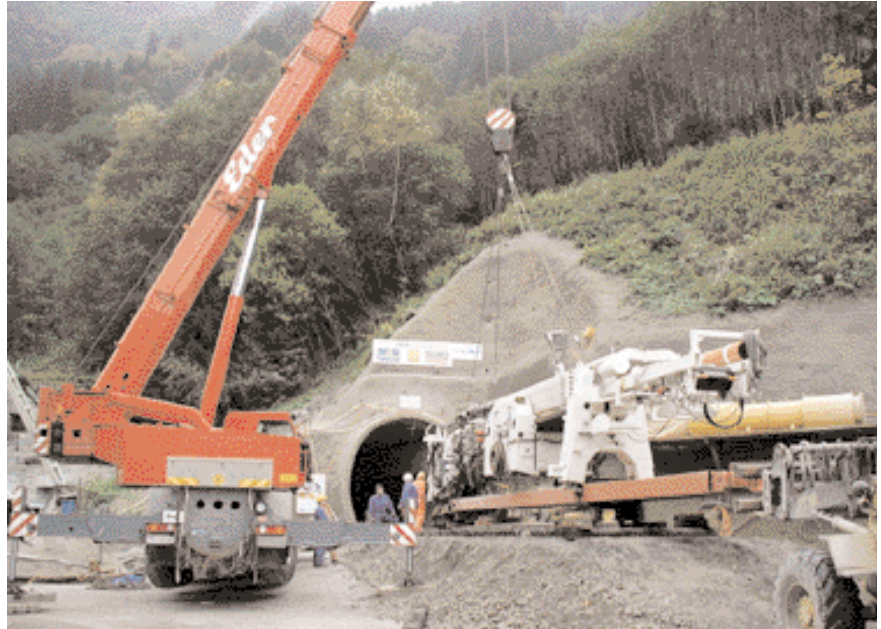
Assembly work on the tunnel boring machine
