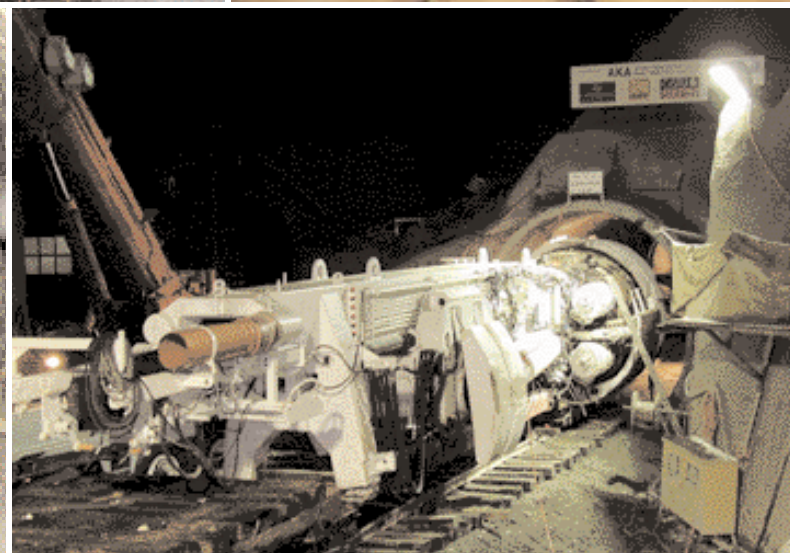
Tunnel boring machine being assembled on a shift system
