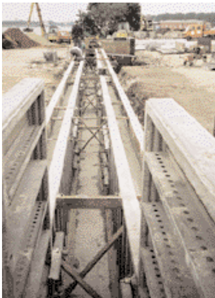
Formwork for the drainage runways
