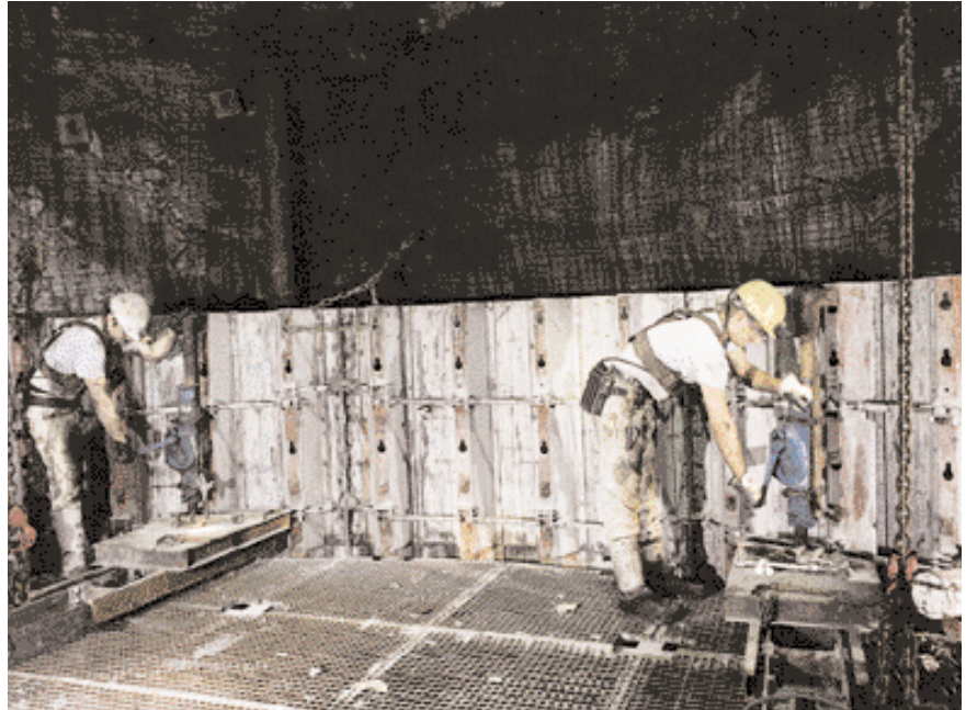
Moving the formwork to a new position
