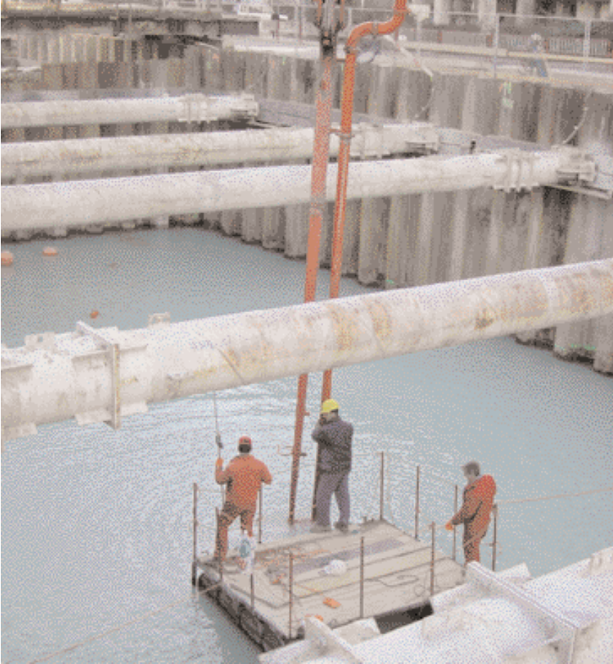
Concreting the submerged concrete floor
