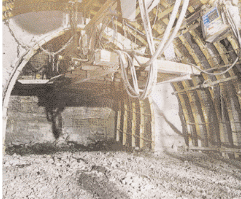
Reducing the breakthrough from the south pass-by to shaft 8
