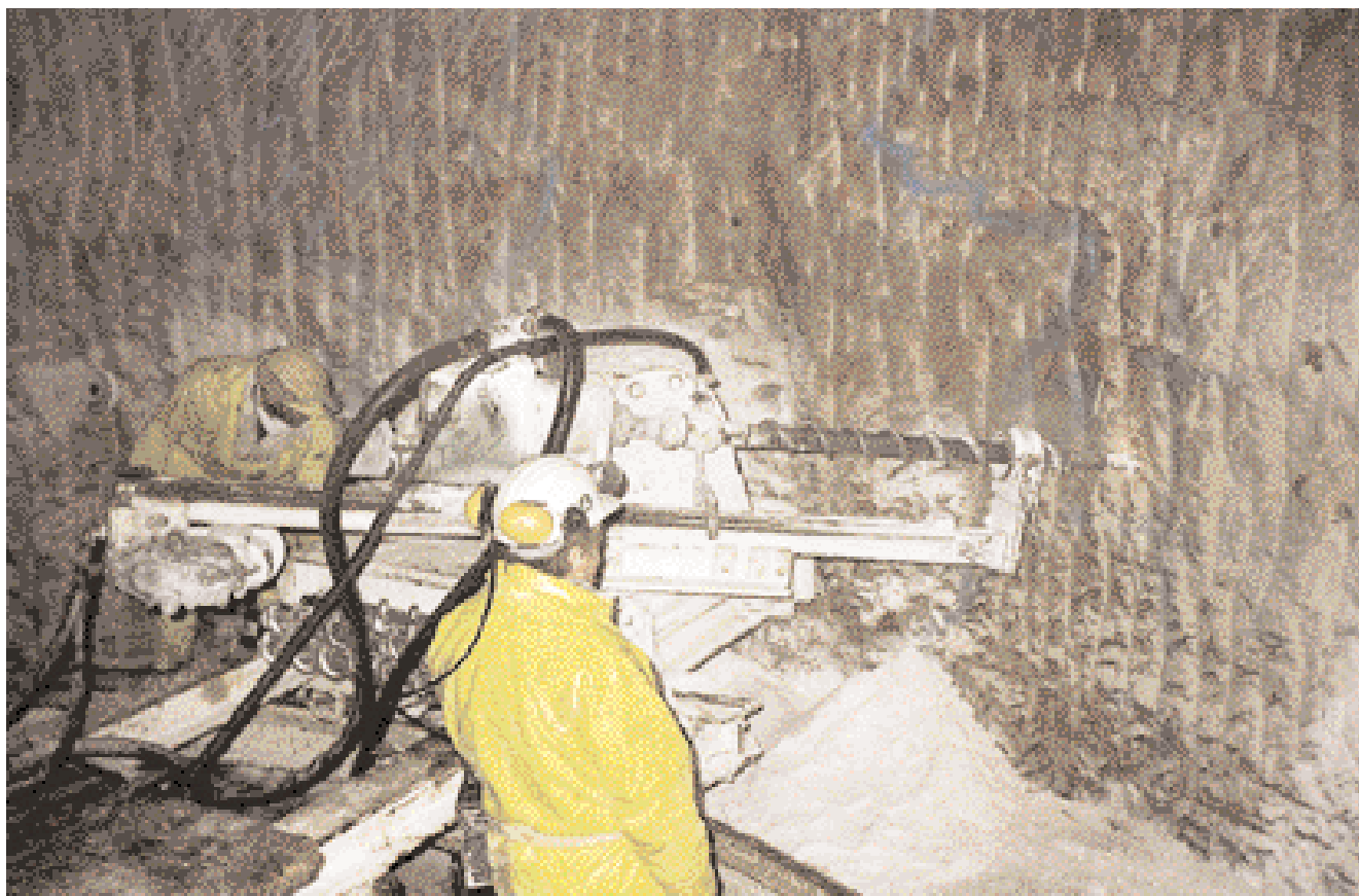
Drilling of horizontal injection boreholes
