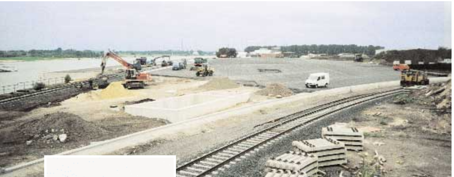
Asphalting in progress
