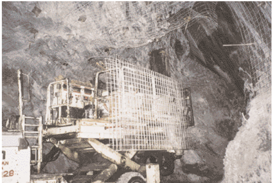
Drill jumbo engaged in setting 4.8-metre resin-grouted bolts
