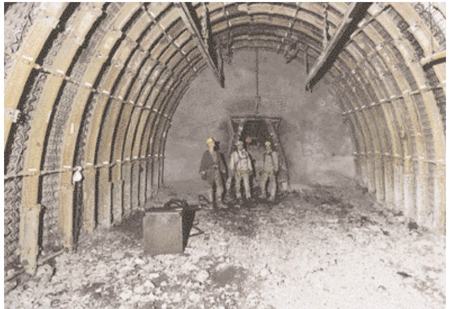
Cutting through to shaft with porch-set support system
