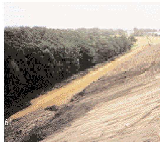
Photo bottom: Lower zone of north slope after surface levelling work
