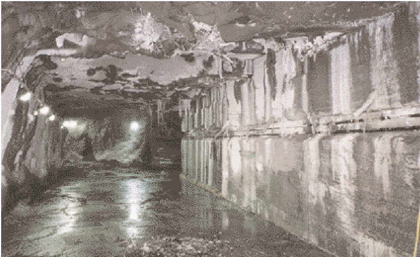
Haulage road alongside dismantled and filled roadway
