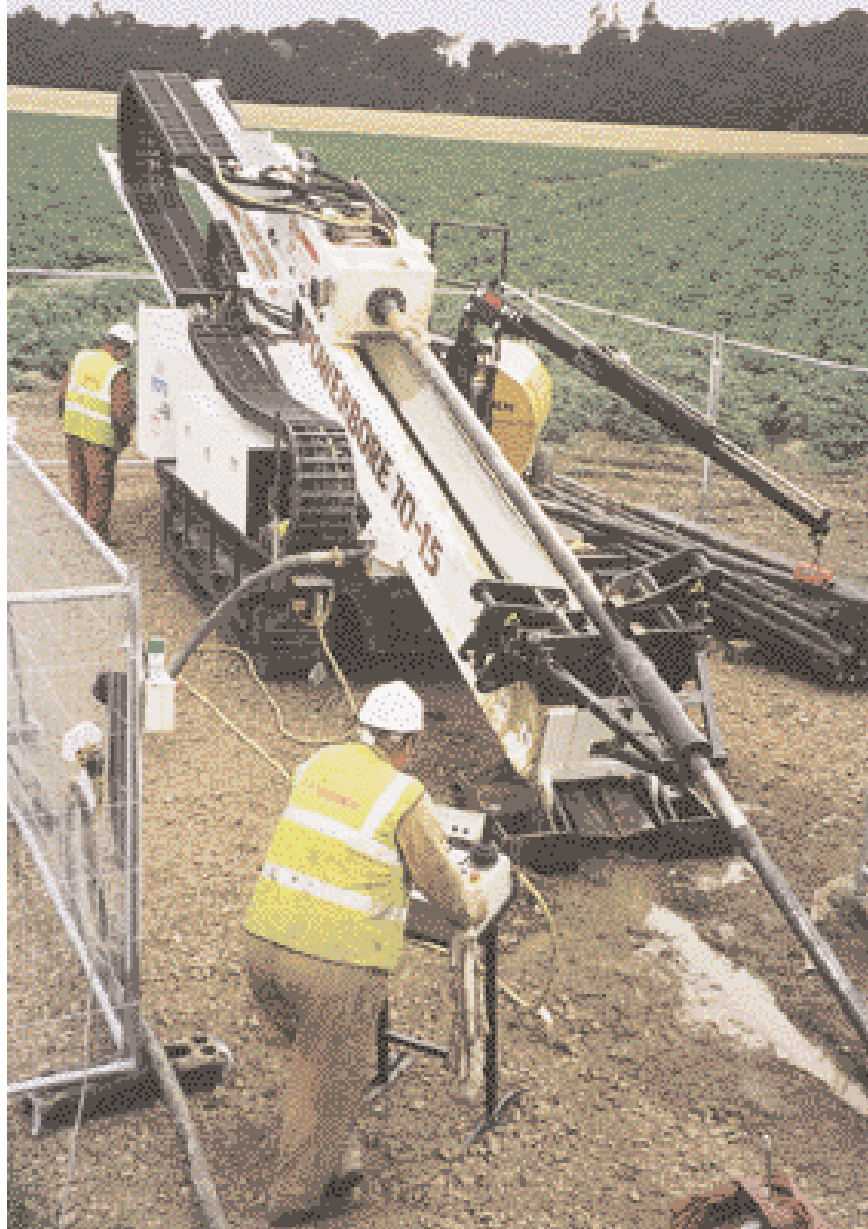
The APPS 70/15 during borehole widening operation
