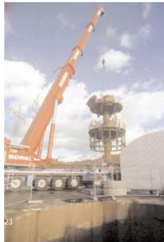
Pre-assembly of the support platform
