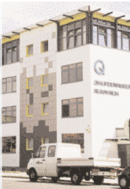
The completed training centre, seen from the Allee Strasse, shortly before the start of term
