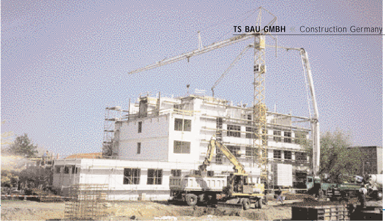
Concreting work for the third-storey floor of the education building (September 2000)
