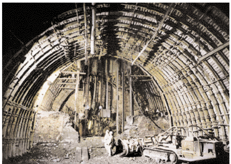
Picture left: Shaft cross-section with ramp, relocated shotfiring platform
