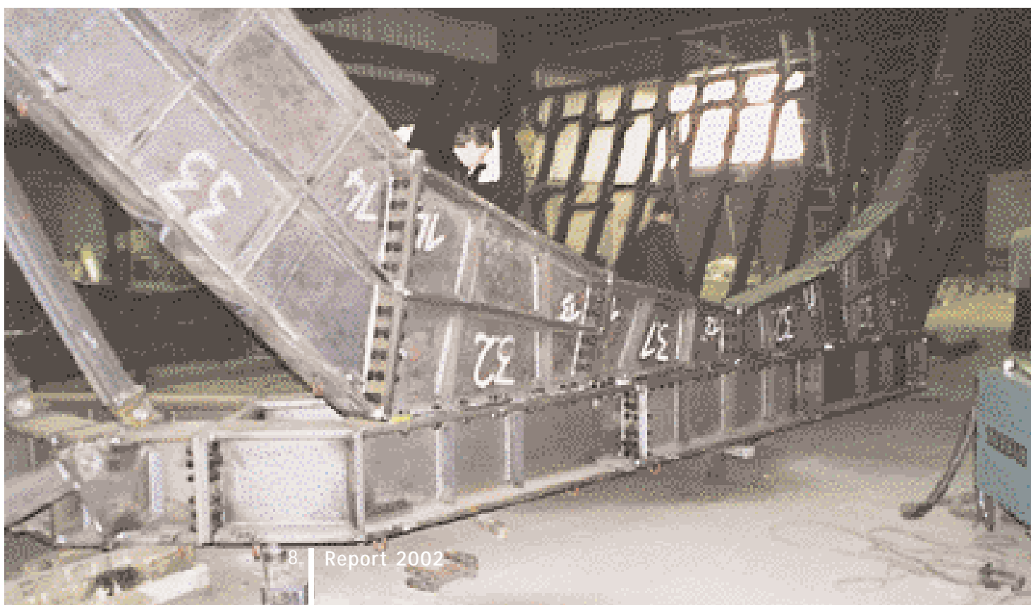
Head frame, polygon and bell inset supports
