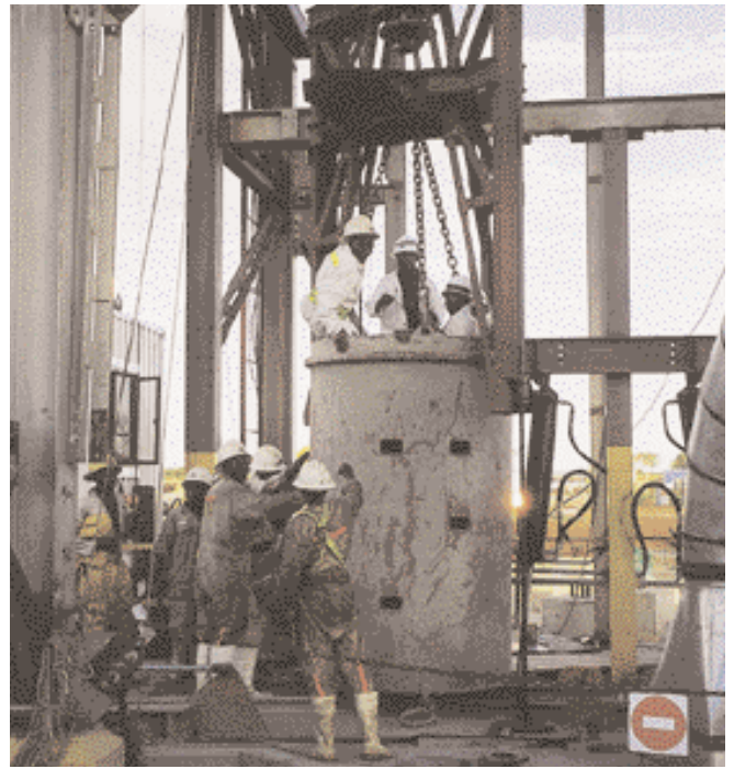
Shaft sinking crew ready to descend
