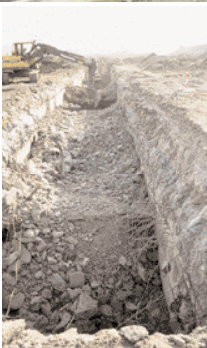
Uncovering an old furnace vault
