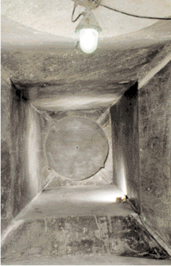
Overall view of finished abutment and sealing contours of the EU-1 roadway dam
