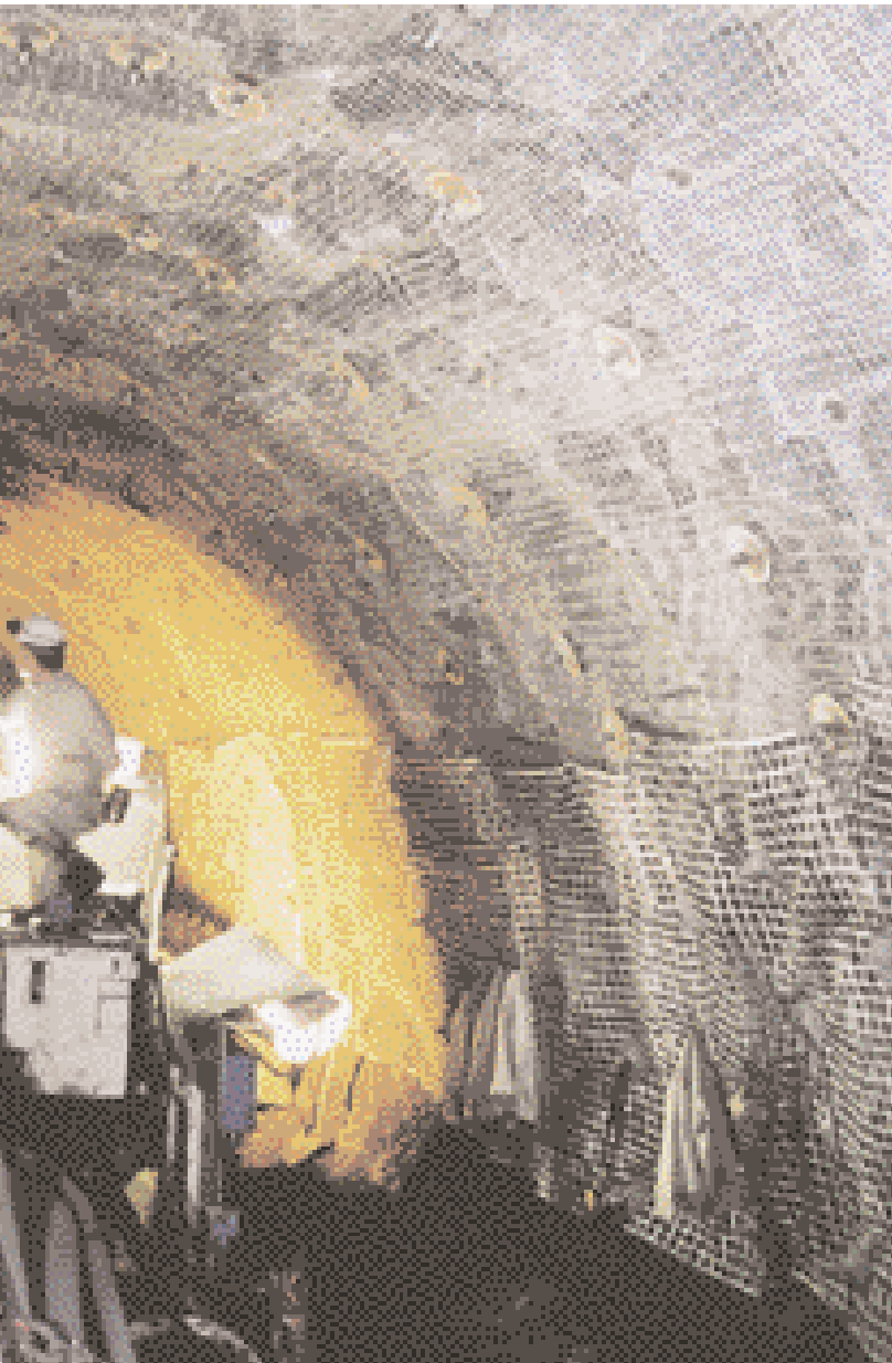
Roofbolting with wire-mesh lagging in heading-machine zone
