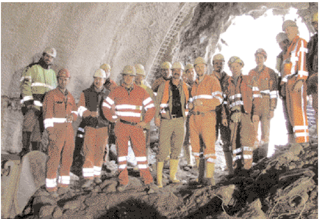
Östu-Stettin GmbH: ÖBB Tunnel, Unterwald. Breakthrough on 21st February 2002
