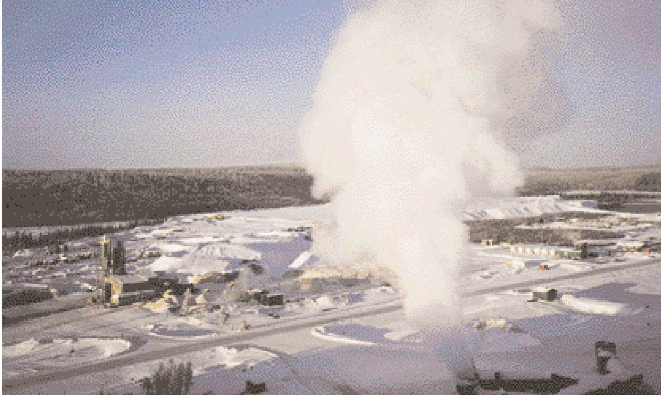
Surface installations in winter with condensation smoke from upcast shaft
