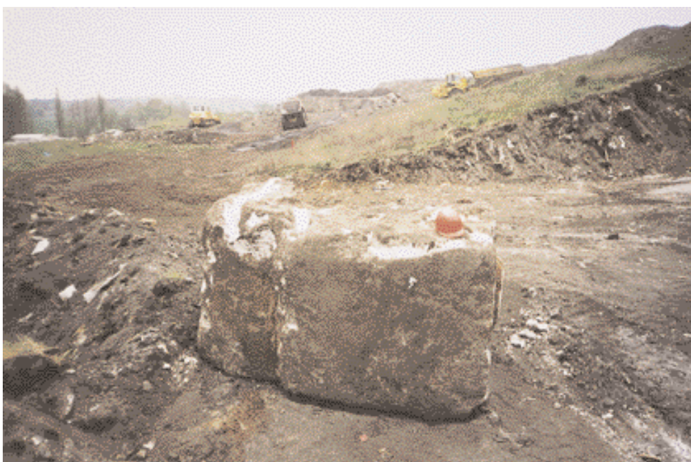
Photo left: Steel-concrete block found during surface profiling work, which had to be broken up at great expense before being ploughed back in
