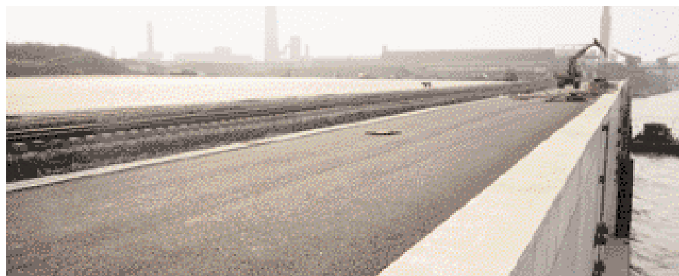
View of the quayside wall
