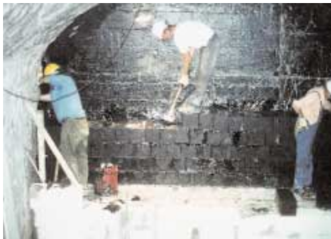
The Hope dam: installing the inner asphalt-sand seal
