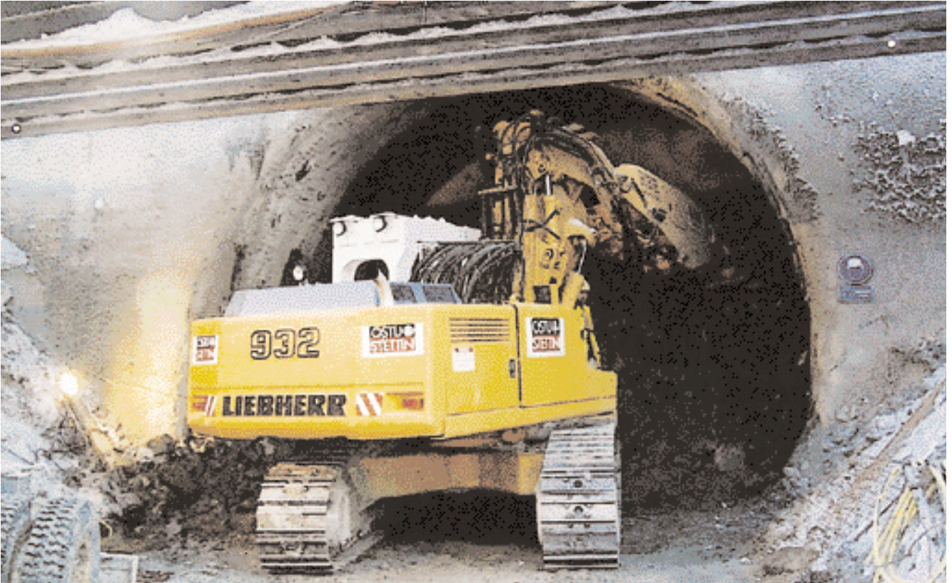
Excavator at the access-tunnel portal/beneath the existing rail embankment
