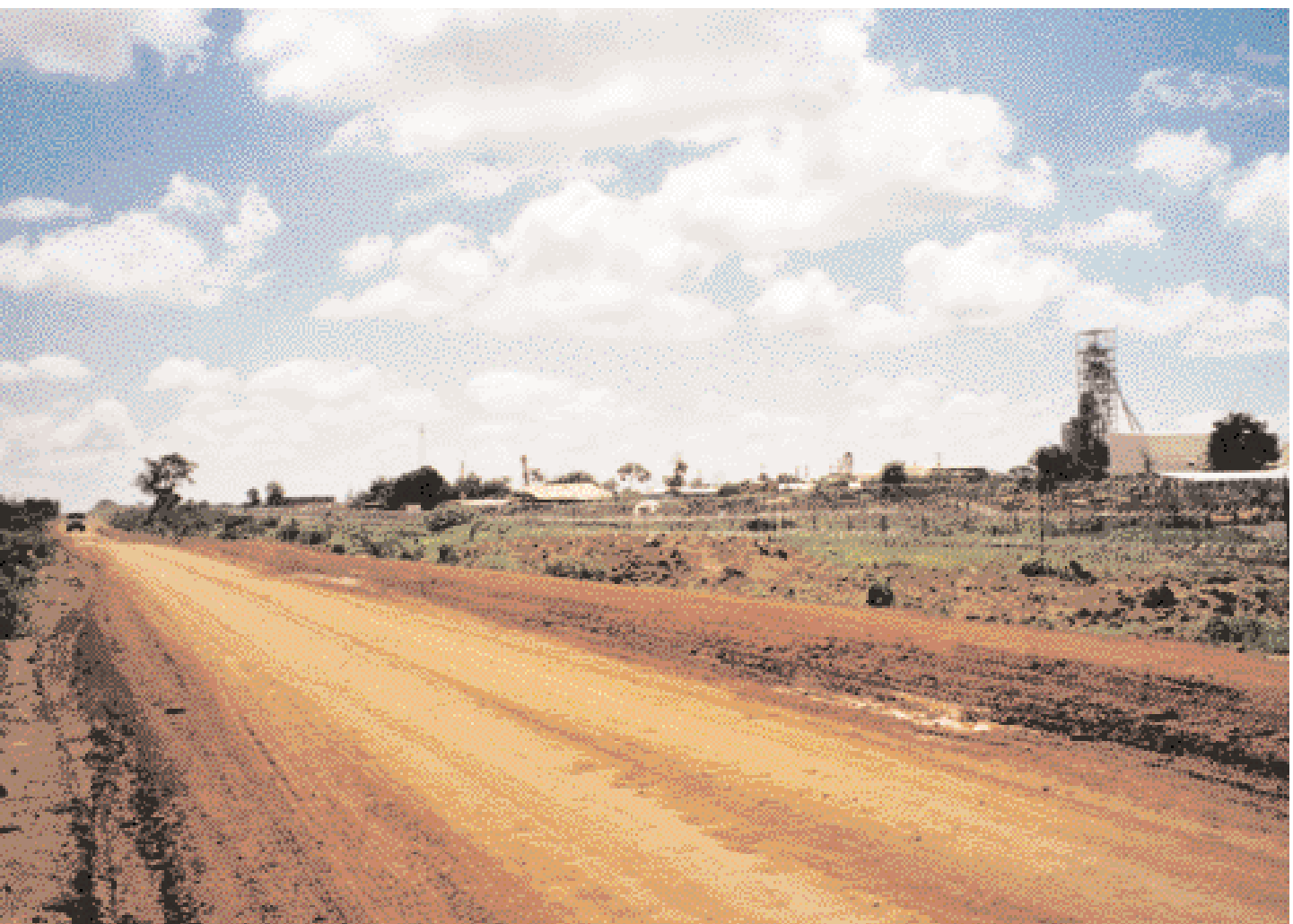
Shaft site with access road
