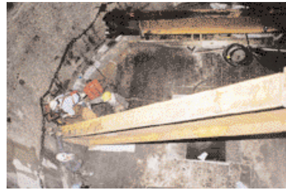
Installation of support beams for working platform
