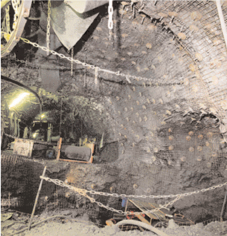
Belt trench excavated to create headroom for the belt transfer station
