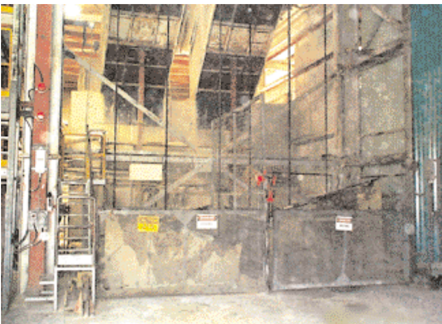
Shaft landing at mine surface
