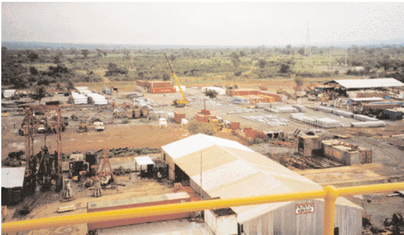
View of shaft site
