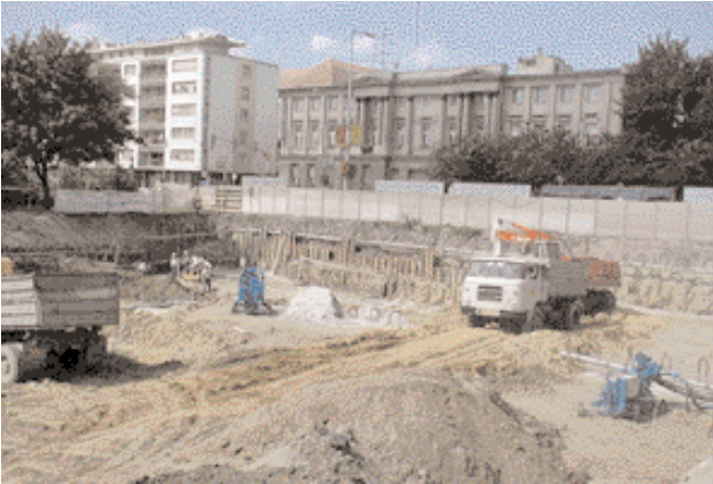
Finishing work for foundations
