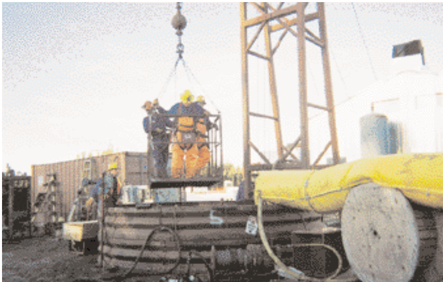
Man winding cage transports workmen down the shaft to help grouting
