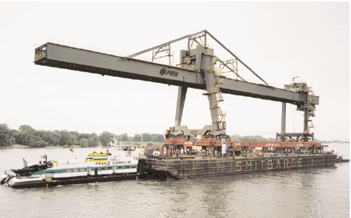
Travelling cranes on tour
