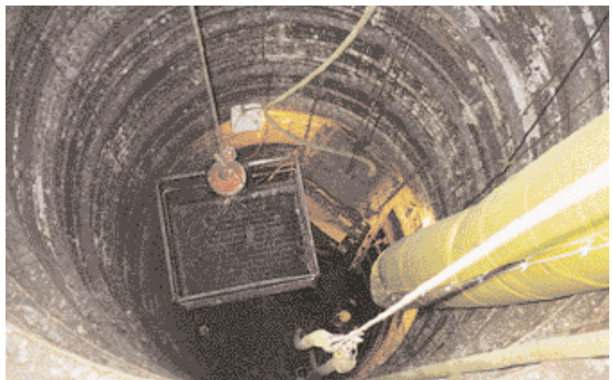
Interior of the shaft with lining system, ring beams and Cryderman-clam
