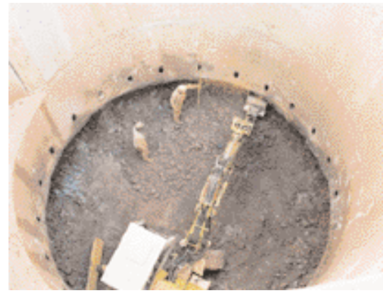
Sinking commences below the shaft collar
