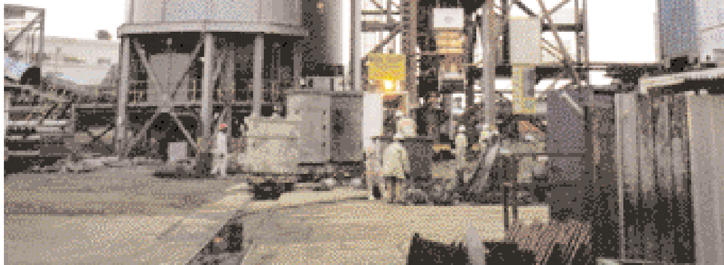
Headgear with ore bunker
