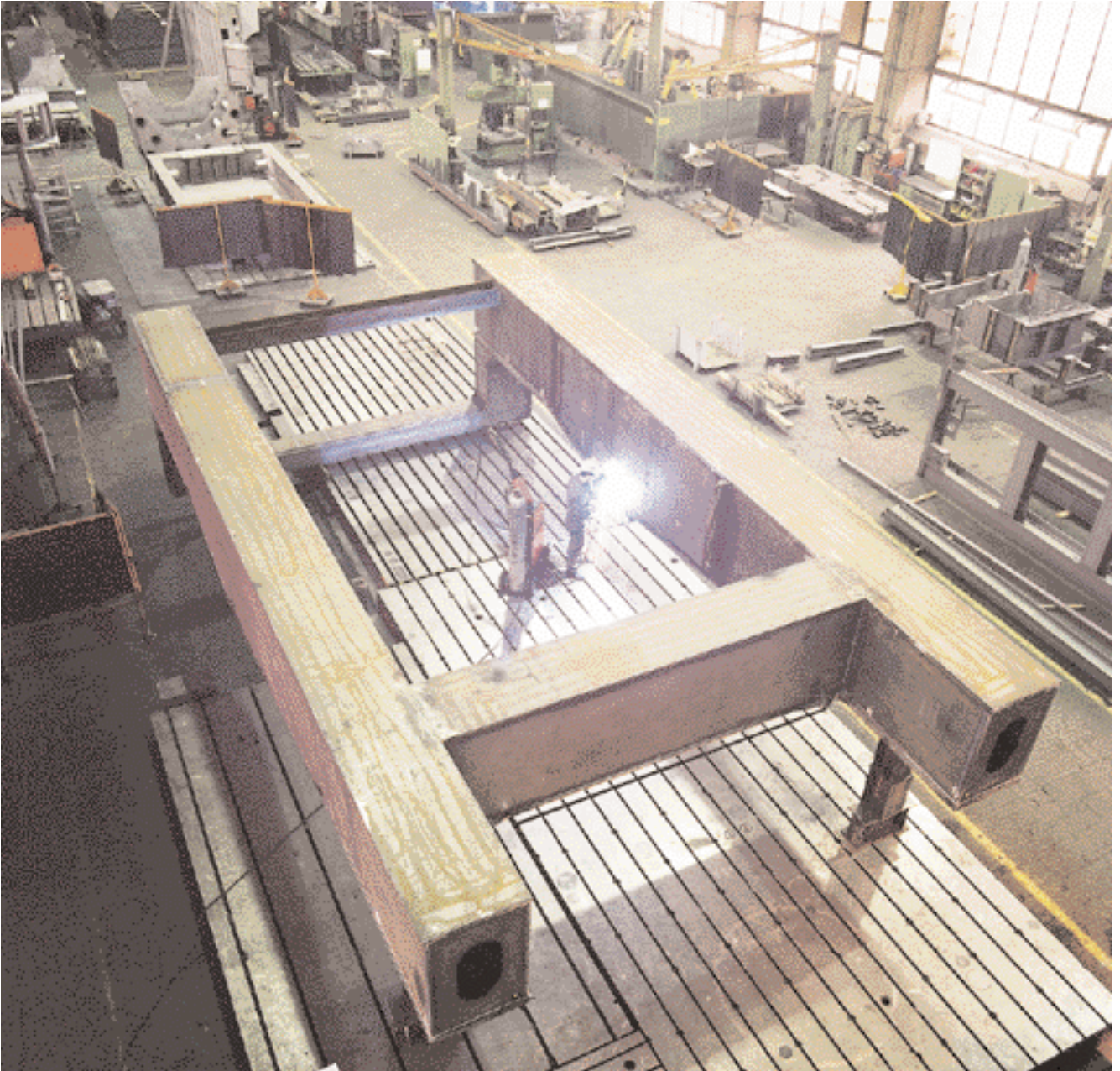
The new ladle car already partly assembled in TS Technology + Service's assembly department
