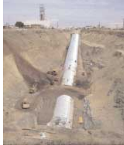
Open-trench working in unstable overburden
