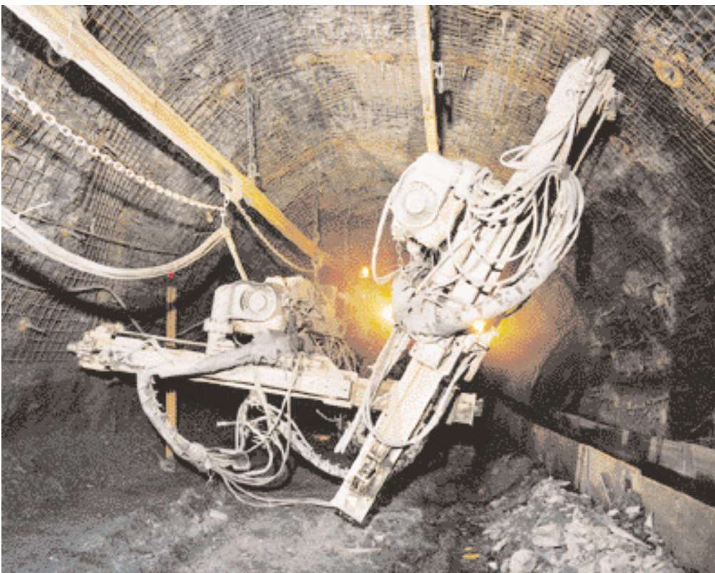
Twin-boom rockbolting jumbo operating in roadway
