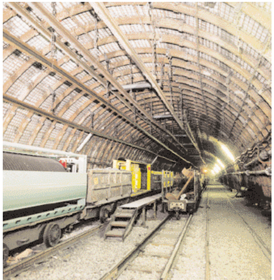
Station 0521 materials transloading point for 07's district, excavated by Thyssen Schachtbau
