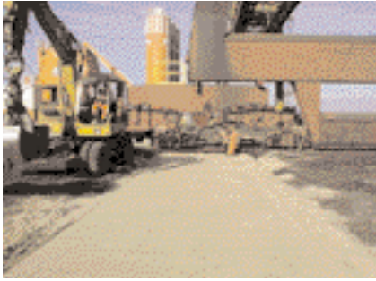
Constructing the transfer ramps
