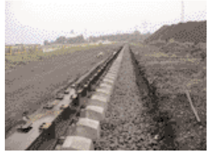
New tracks for overhead travelling crane Formation work
