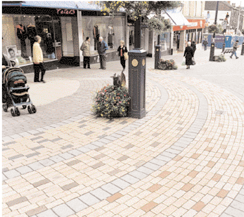
Photograph showing intricate block paving to pedestrianised area.
