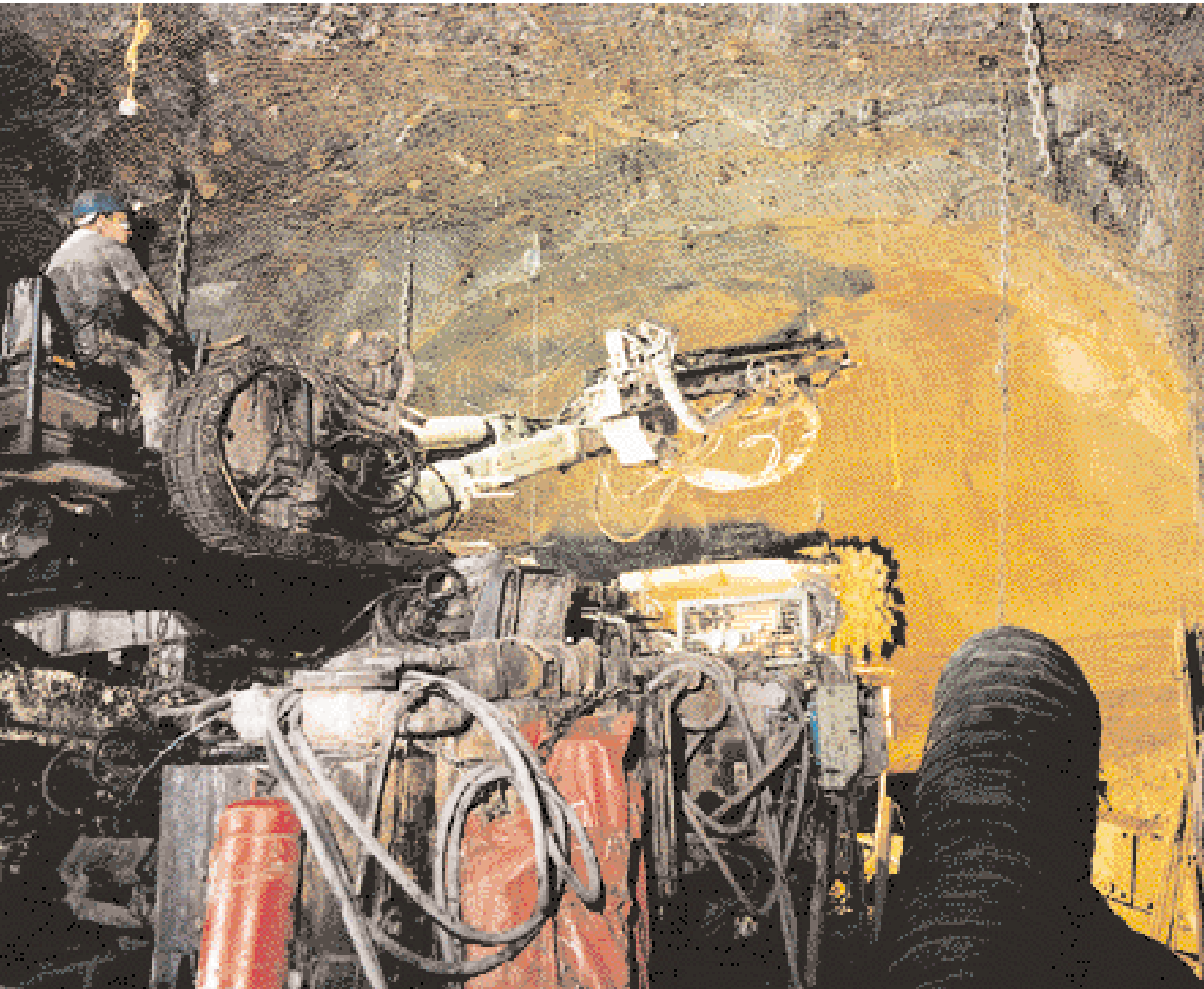
Full roofbolting at the roadhead
