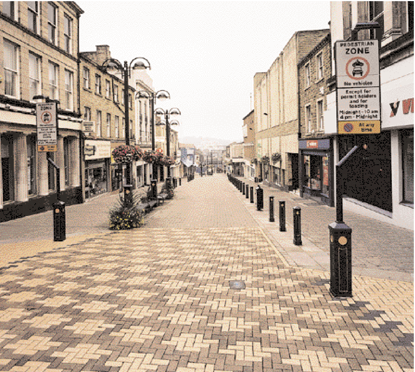
Photograph showing block paving and feature lighting to pedestrianised area.
