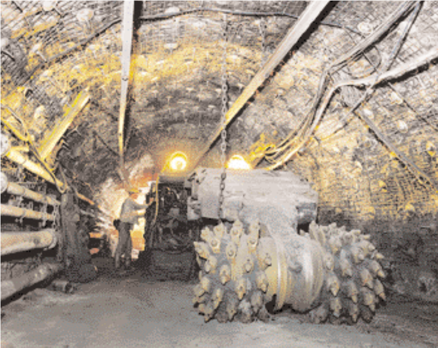
The AM 85 takes a "well-earned break" after completing the loader-gate drivage
