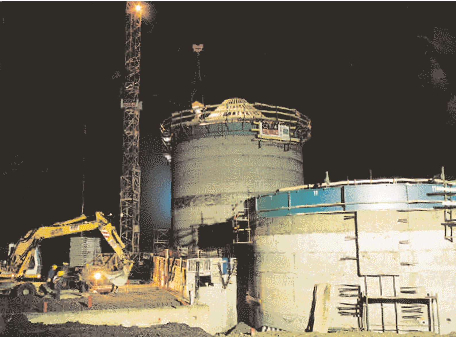
Digestion chamber with roof casing, thickener and foundation for tower block
