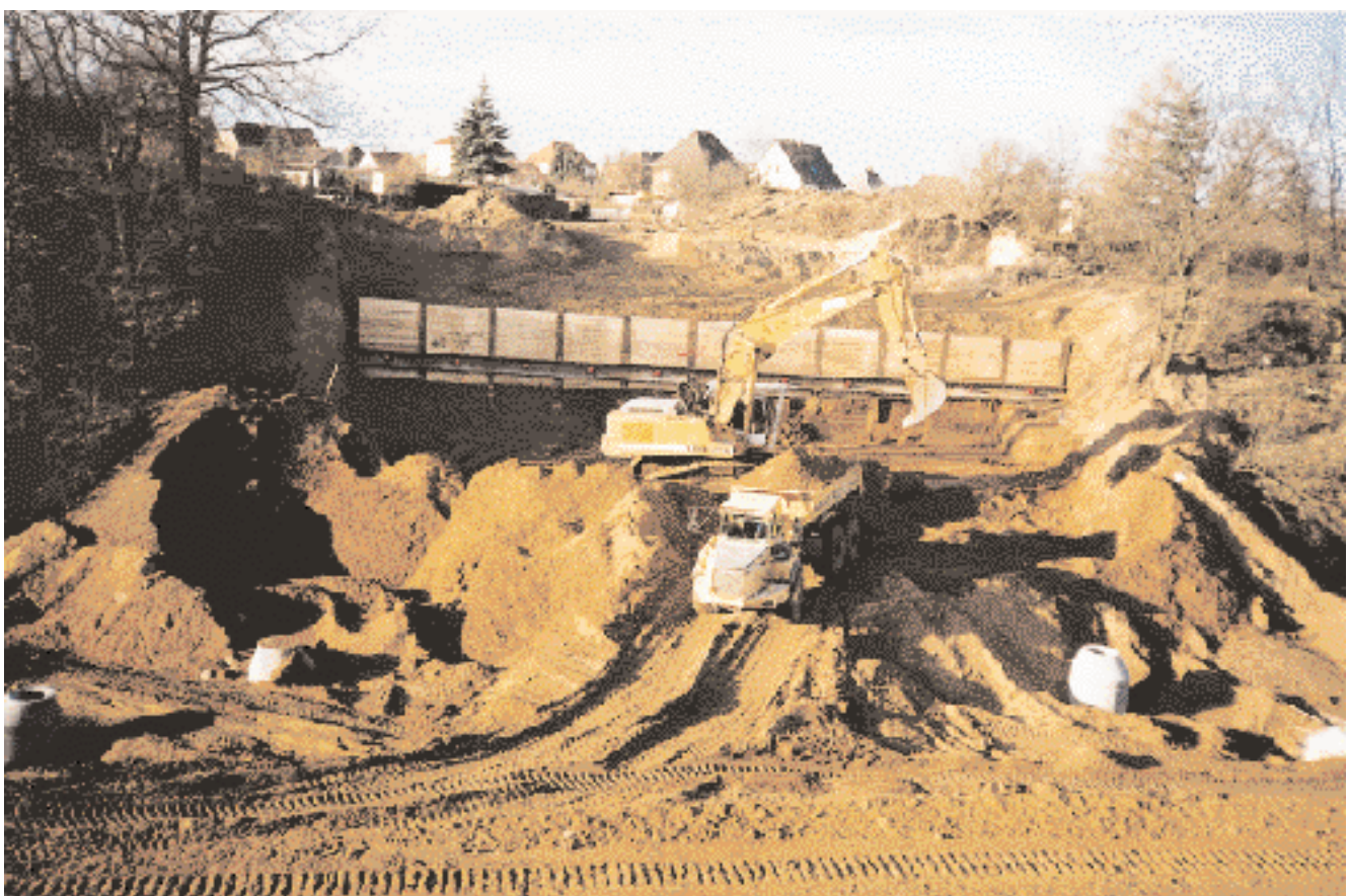
Earth-moving operations for bridge construction work
