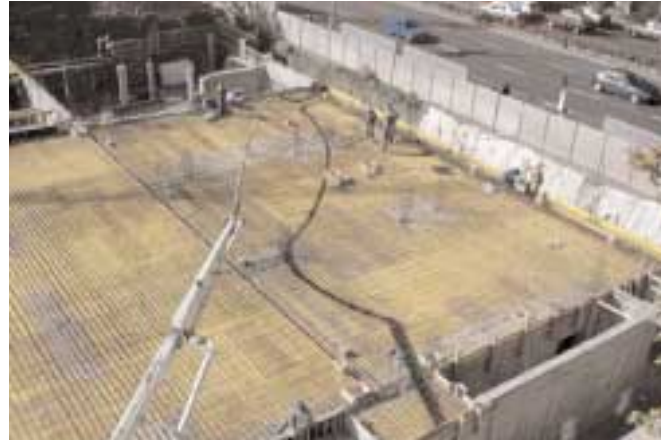
Concreting the ceiling above cellar level
