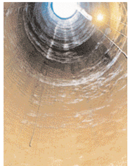
Temporary shaft lining comprising rockbolts, steel mesh and shotcrete
