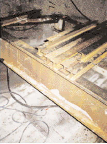
Stage support beams with working platform below
