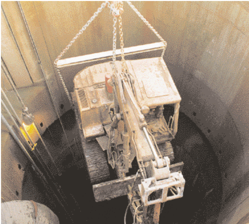
Excavator being lowered to the shaft floor
