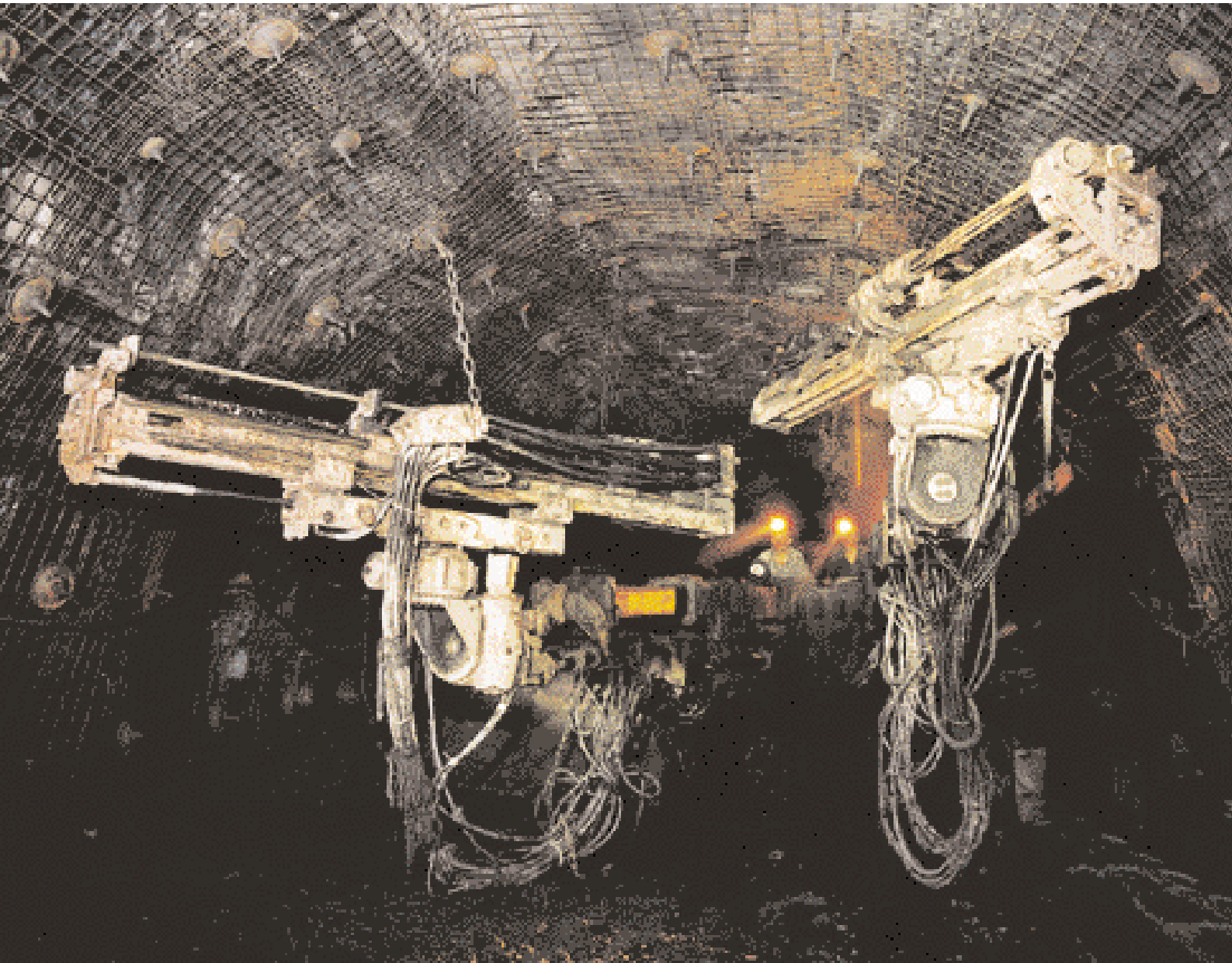
Twin-boom drill jumbo for rotary boring of rockbolting holes
