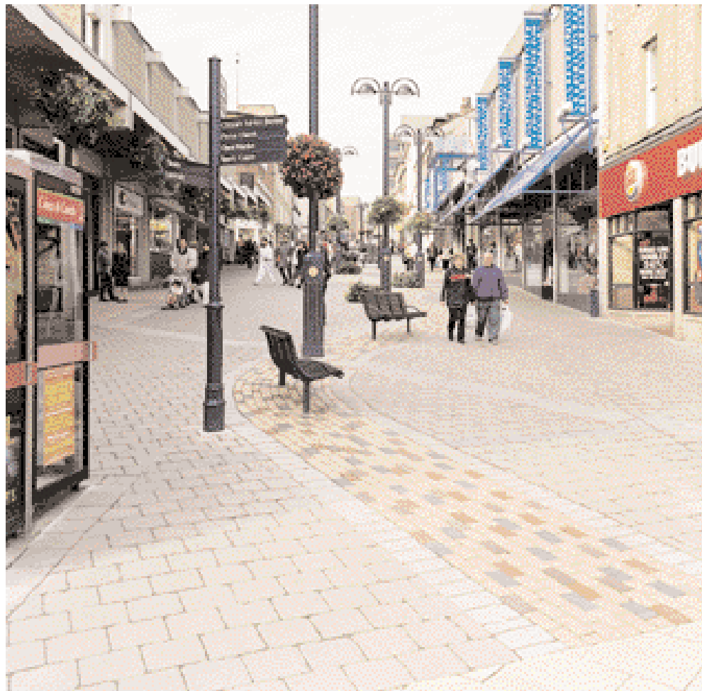
Photograph showing intricate block paving to pedestrianised area.
