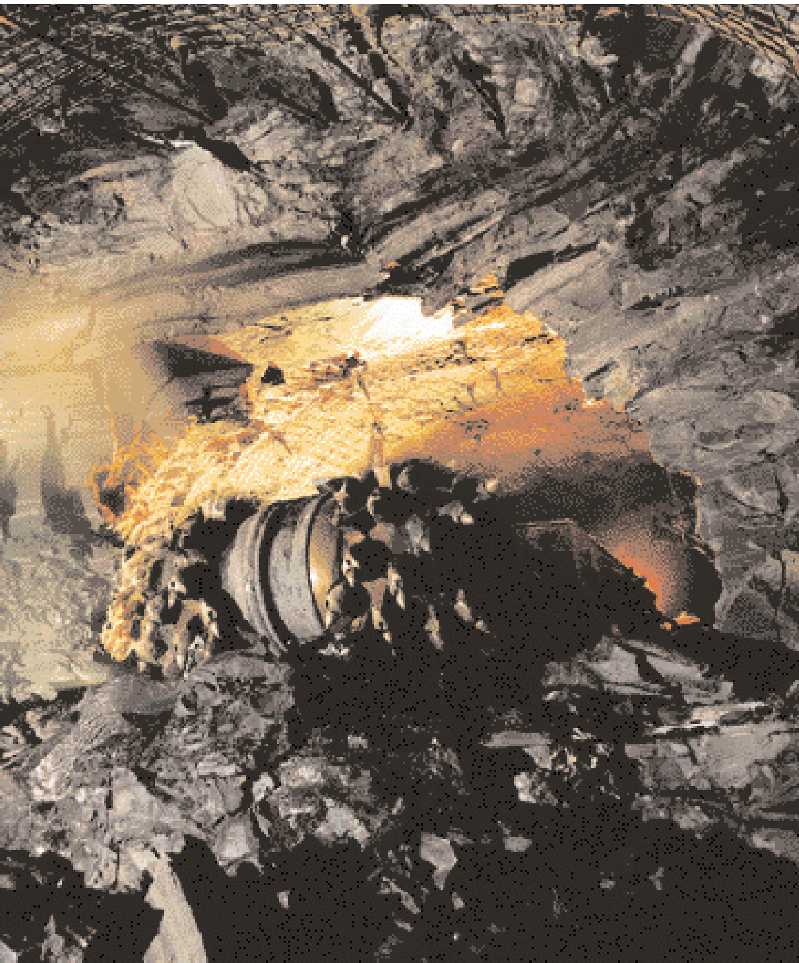
AM 85 roadheading machine breaks through into roadway 4641
