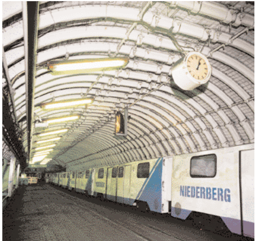
Picture above: Access passage leading from shaft to high-speed manriding station
