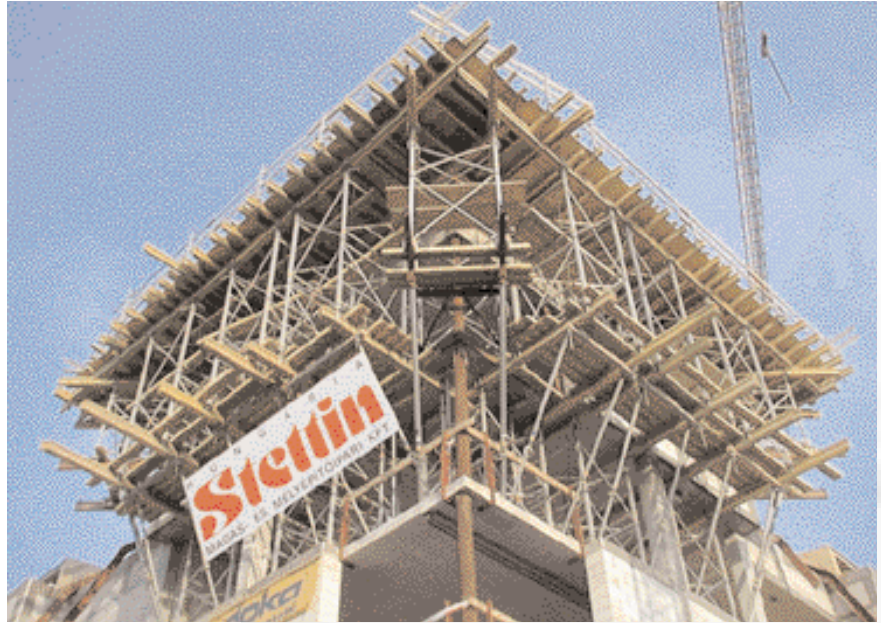
Shuttering of main cornice
