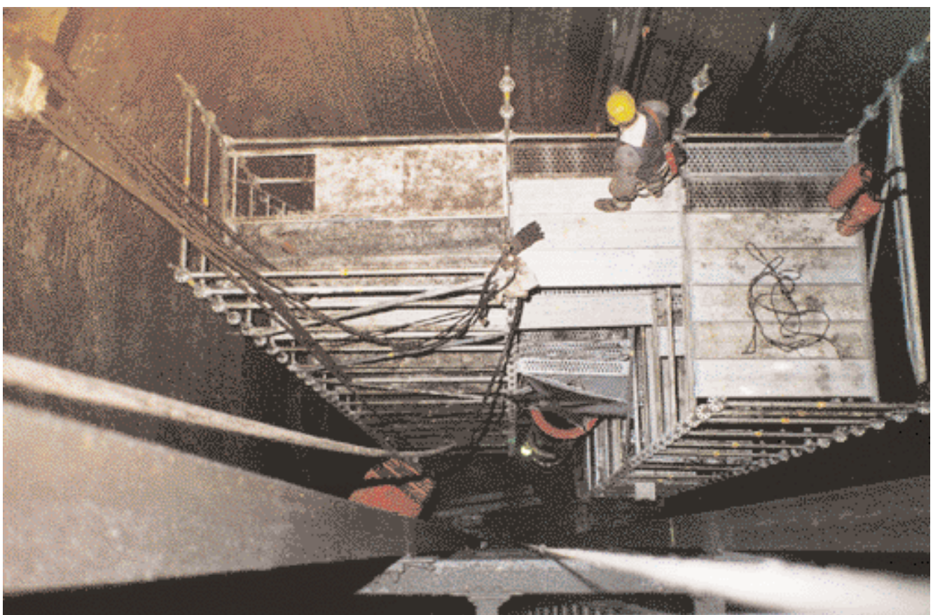
Completed construction scaffold
