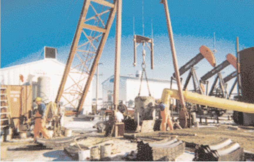
The headframe is elevated to the right position
