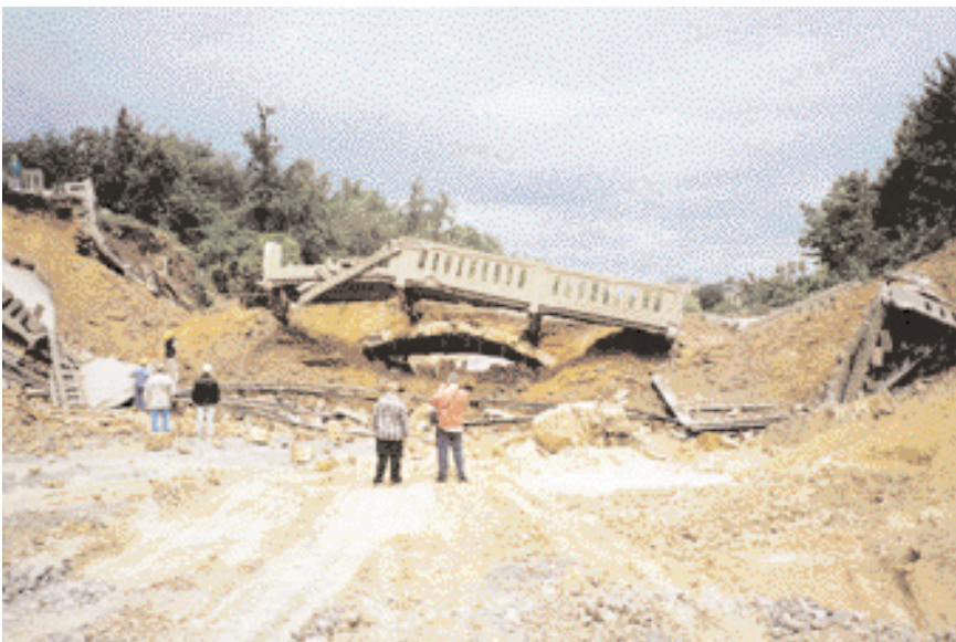
Demolition of existing bridges on Breitscheidstrasse
