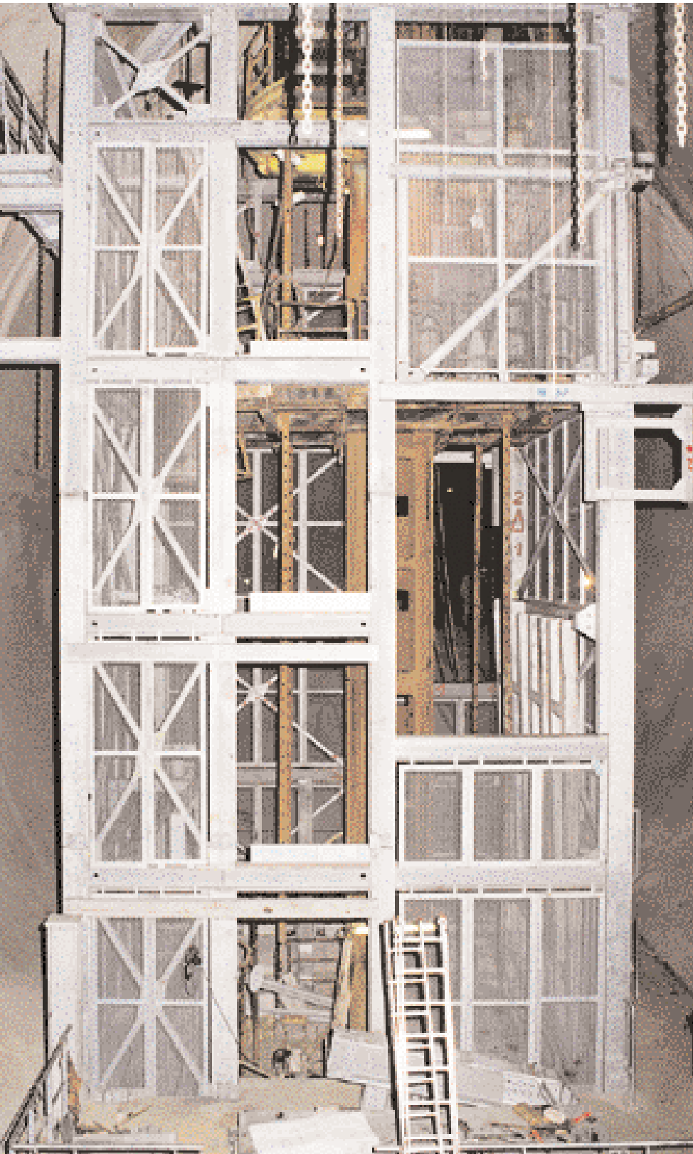
160-tonne bottom frame is assembled from the Mega-platform
