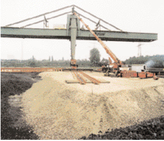
Transfer ramp at Walsum south dockyard
