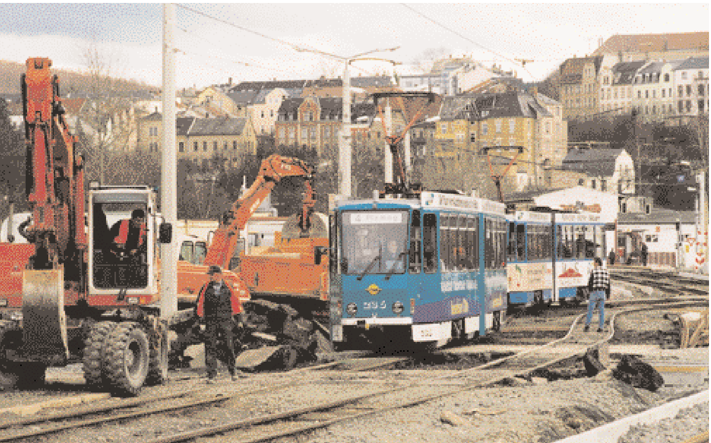
Working space is confined by ongoing tramcar services
