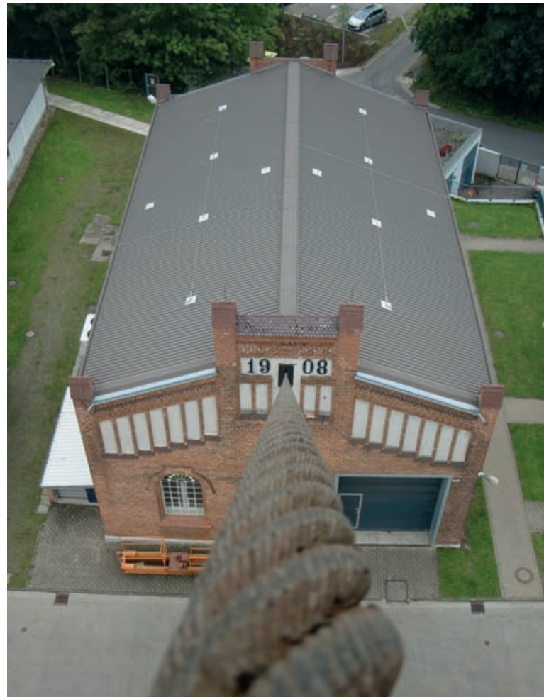
A heritage protected winch house from the Asse II mine (built in 1908)
