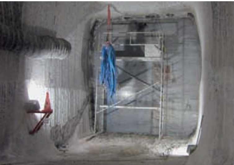
“Air-side“ of the infal dam construction
