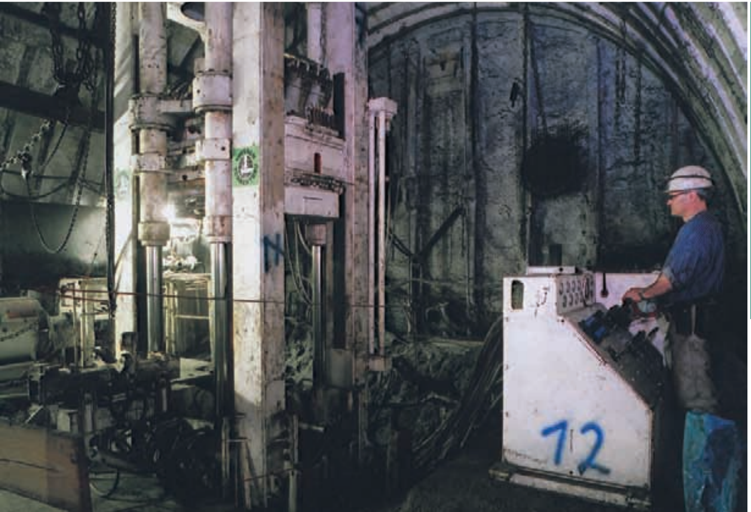
Raise boring HG250 while drilling
