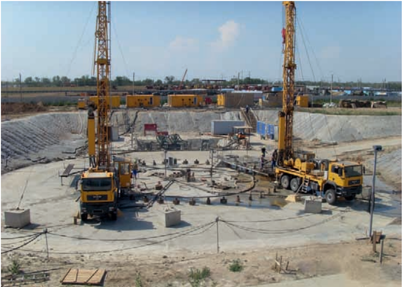
Drilling operation for freezing holes with both drilling rigs RB50
