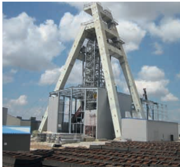
Head frame of shaft 2
