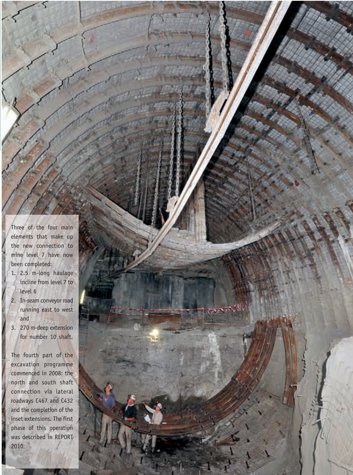
Steel support assembly with systematic bolts at the bottom
