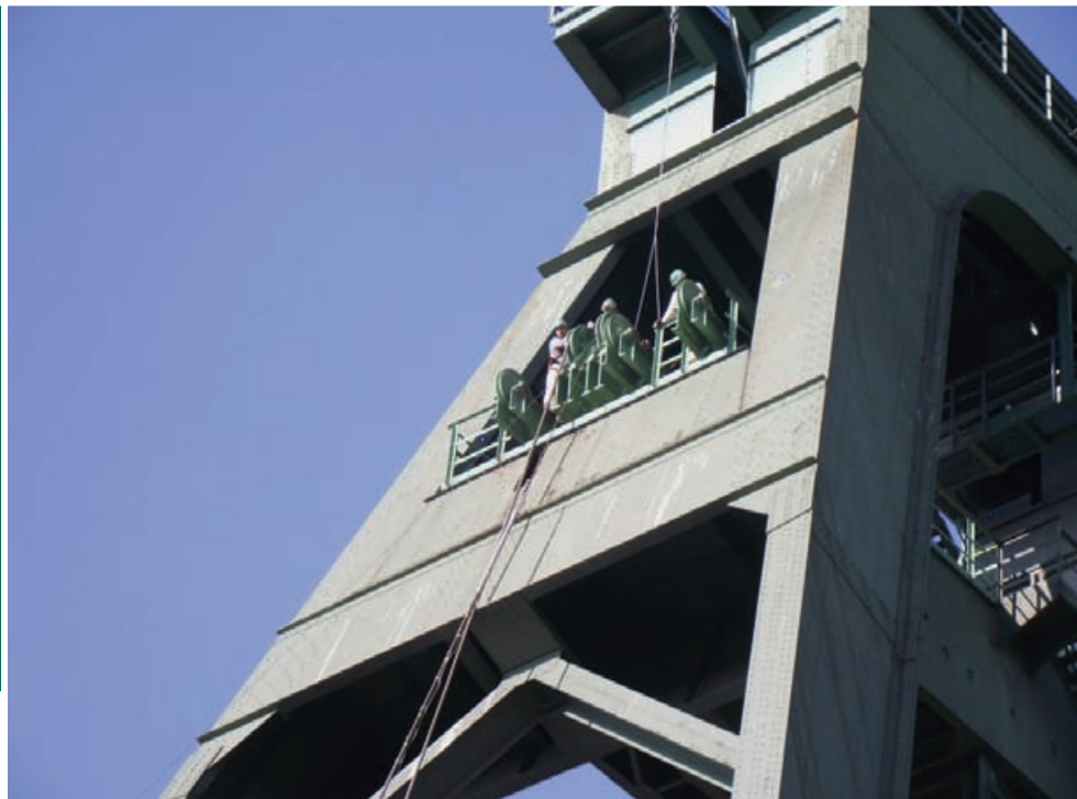
Rope assembling at shaft K1
