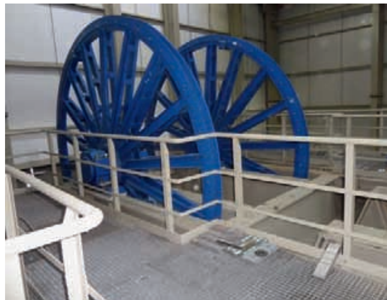
Working stage on the rope pulley WS-10
