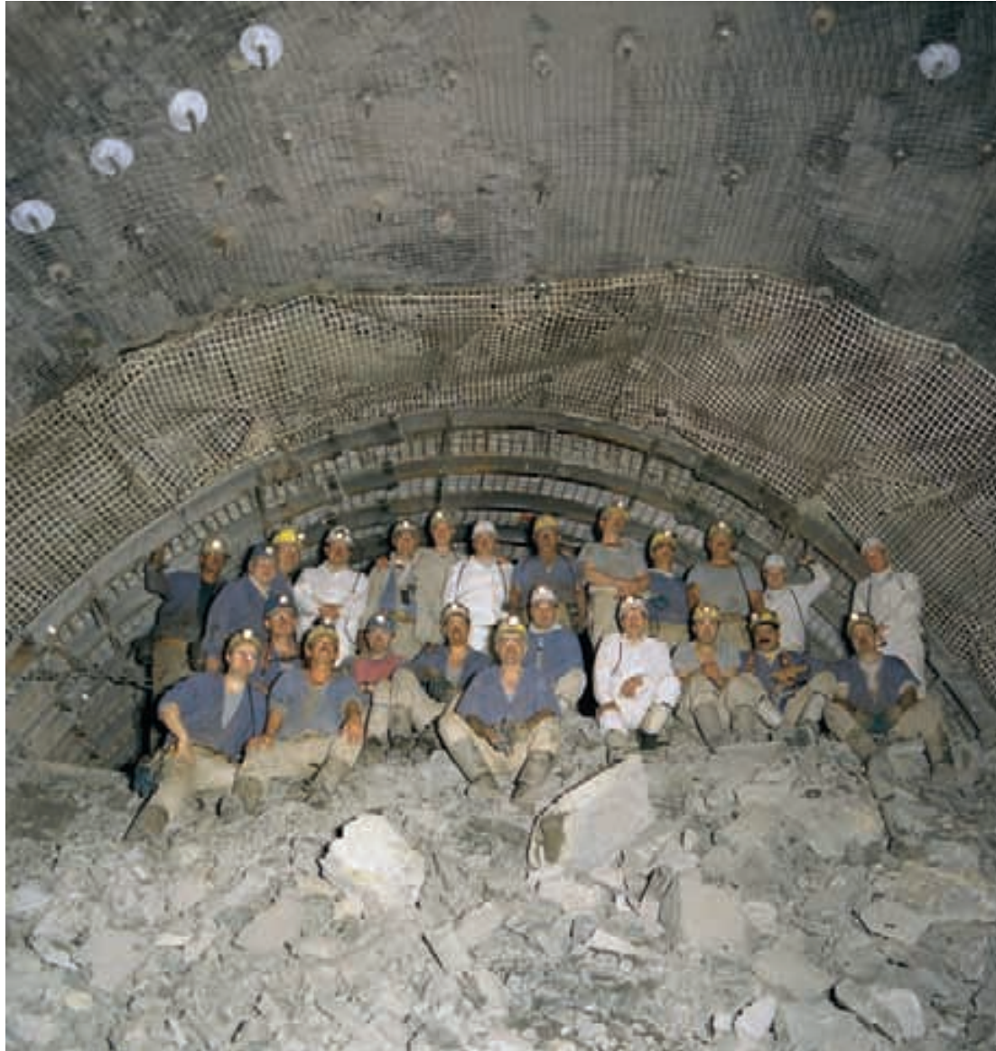
The final breakthrough C432 for the southern shaft-landing
