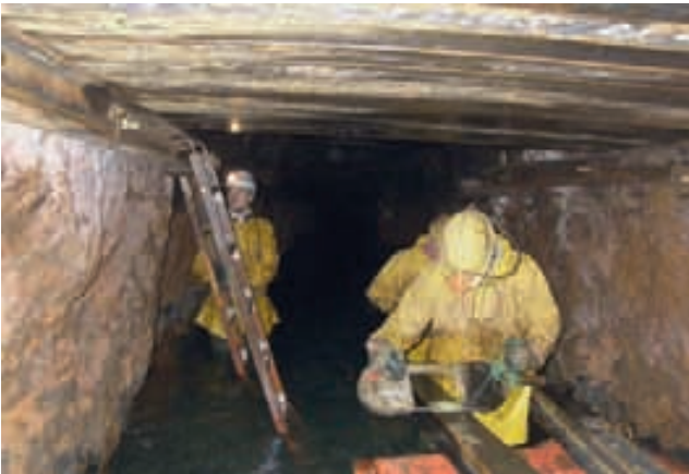
Inset at Rothschönberger adit
