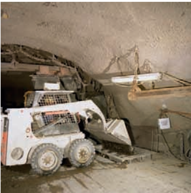
Bobcat next to the tipping area
