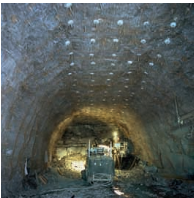
Tunnelling C432 in combined support type
