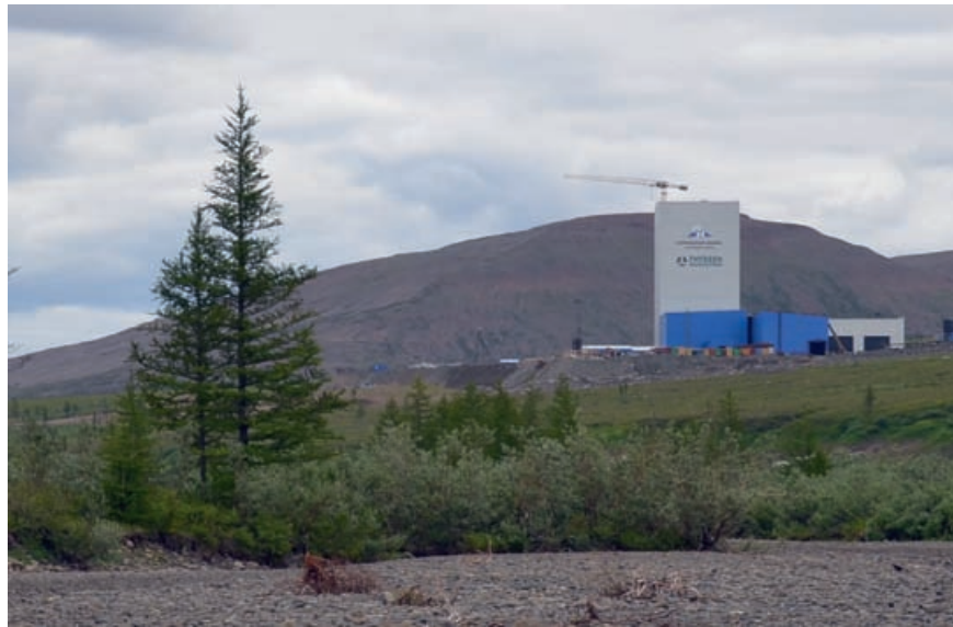
Shaft sinking in impressive nature
