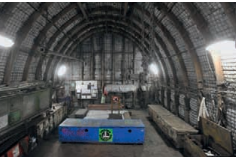
Drilling chamber, access to ventilation borehole
