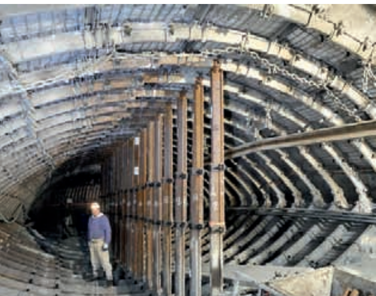
Steel support in section I with props
