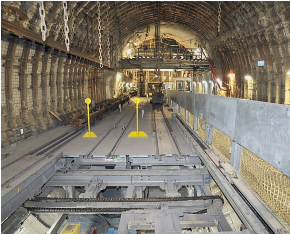
Southern shaft-landing with railway track
