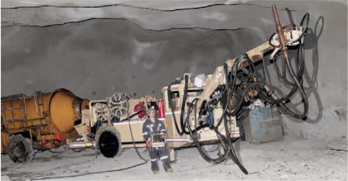
Shotcrete vehicle with silo truck
