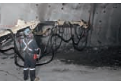
Shotcrete vehicle while grouting a concrete layer
