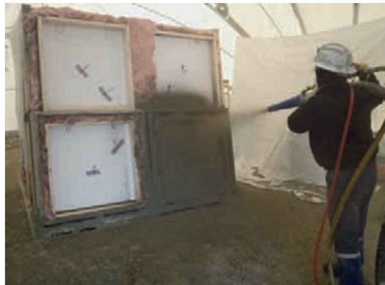
Shooting shotcrete onto test panels
