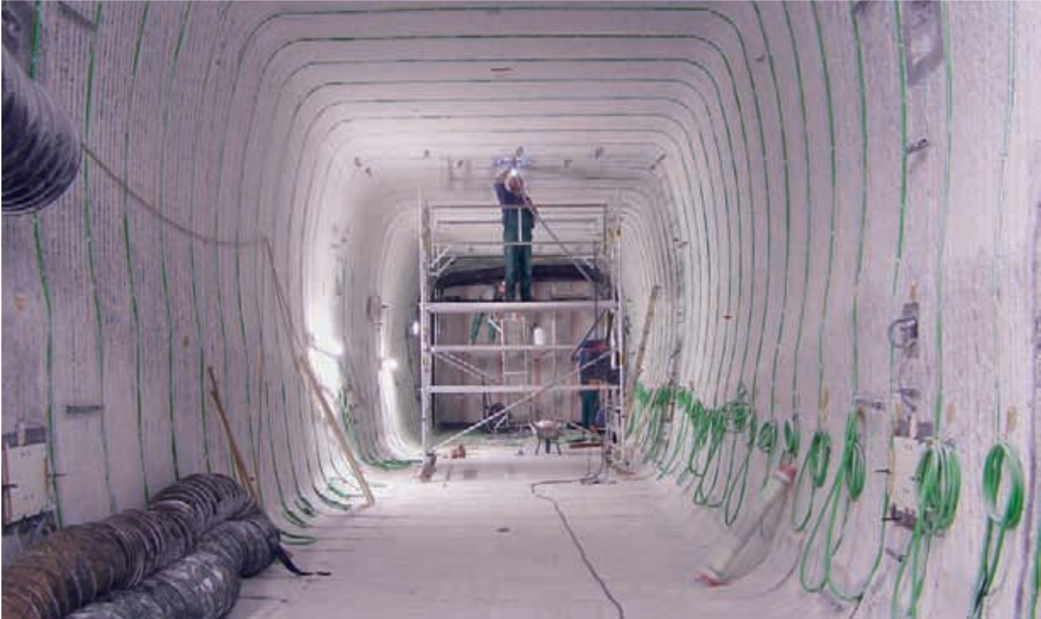
Assembling of the measurement system and cementation technology
