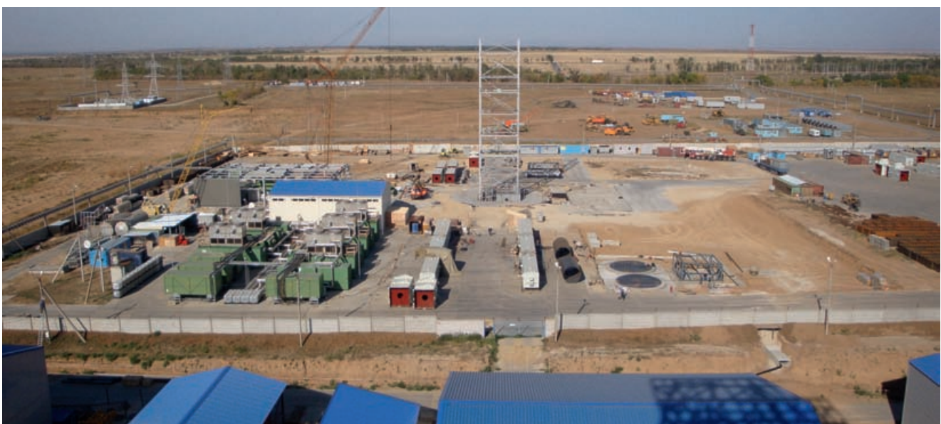
View of the shaft construction site
