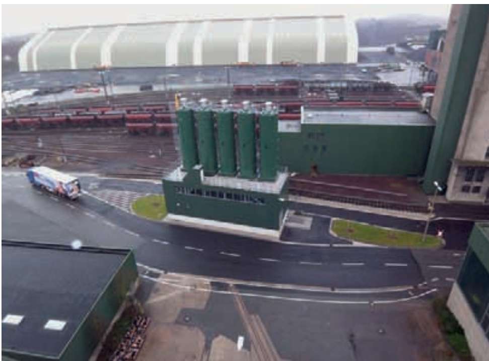
Building materials plant at RAG Anthrazit Ibbenbüren GmbH
