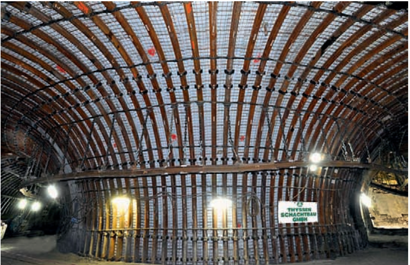
Curve C432 in direction southern pit bottom
