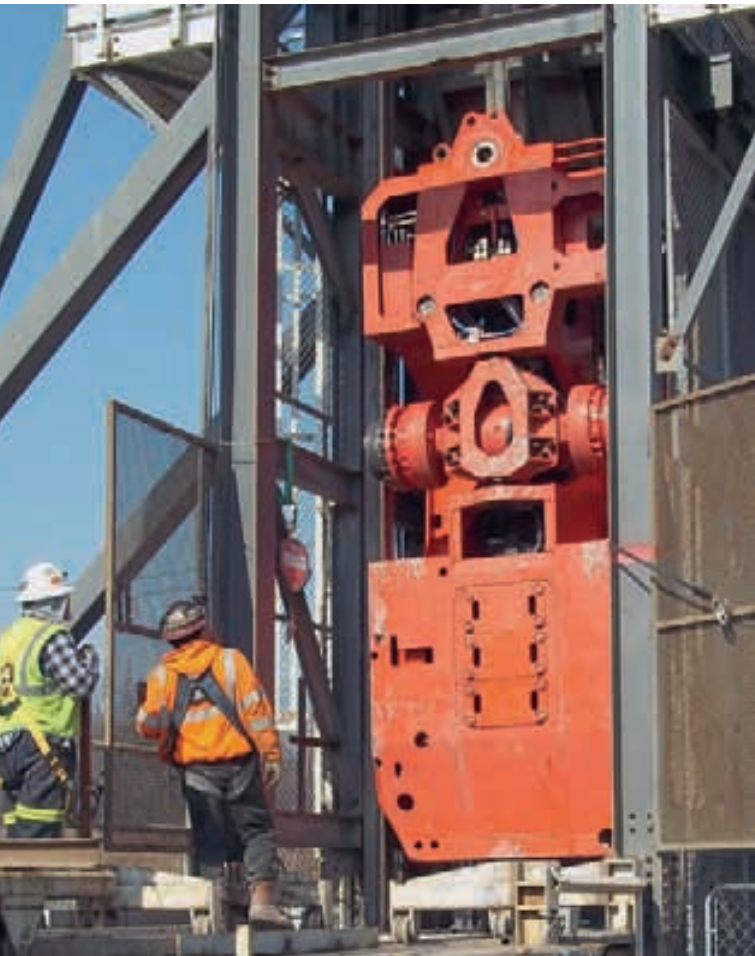
Transport of a wheel loader into the underground
