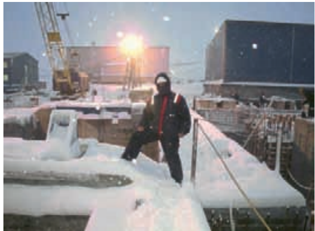
Extreme climatic working conditions
