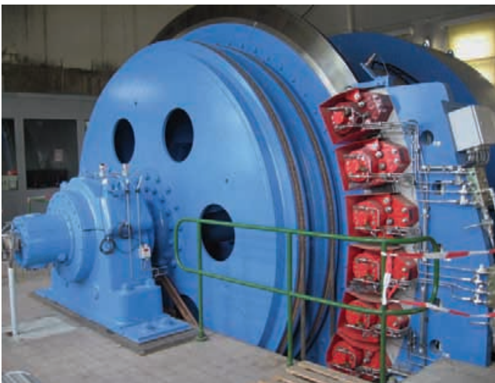
Shaft winders – Borth 2 (right) and Borth 1 (left)
