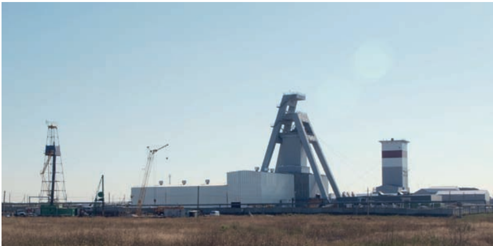
Figure 1: View of the three shaft sites at the EuroChem-VolgaKali mine; from left: second skip winding shaft, first skip shaft, service shaft
