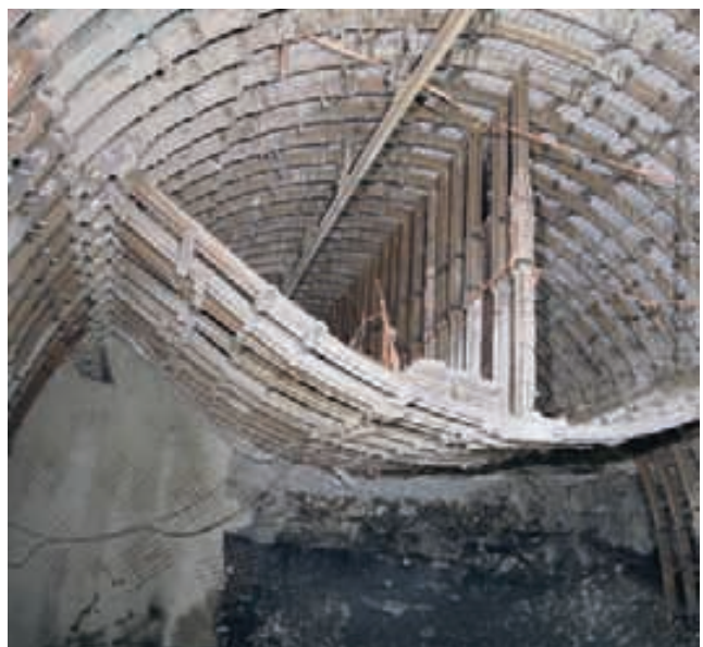
Tunnelling in section 2a and 2b
