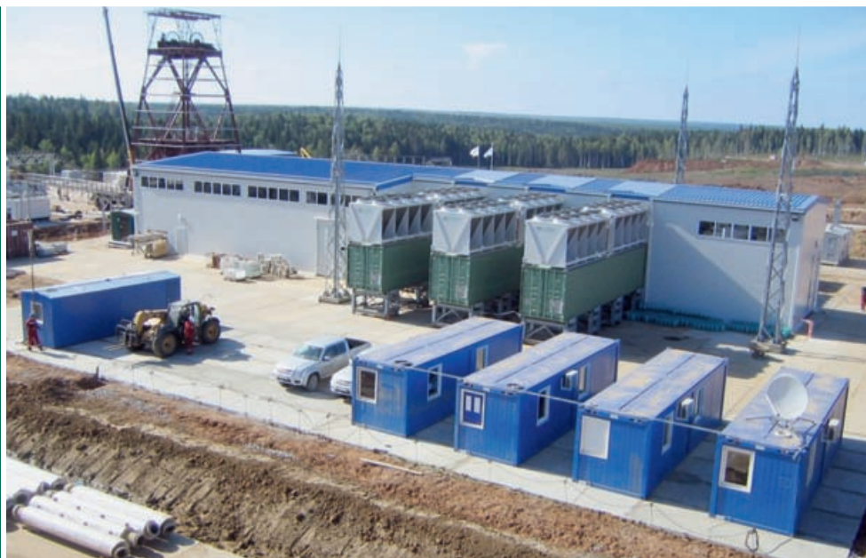
View of freeze plant and headgear for shaft number 1
