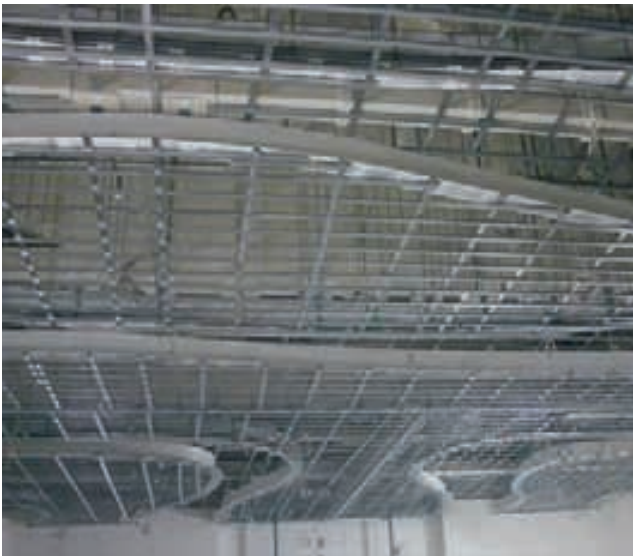
Ballroom ceiling Hilton hotel during construction phases
