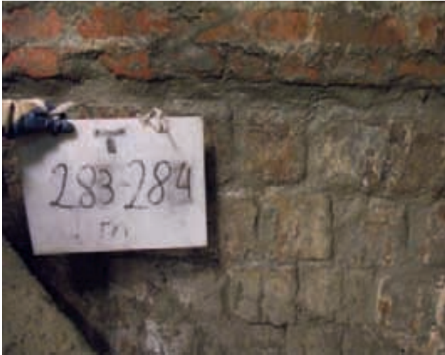
Cleaned and grouted shaft wall
