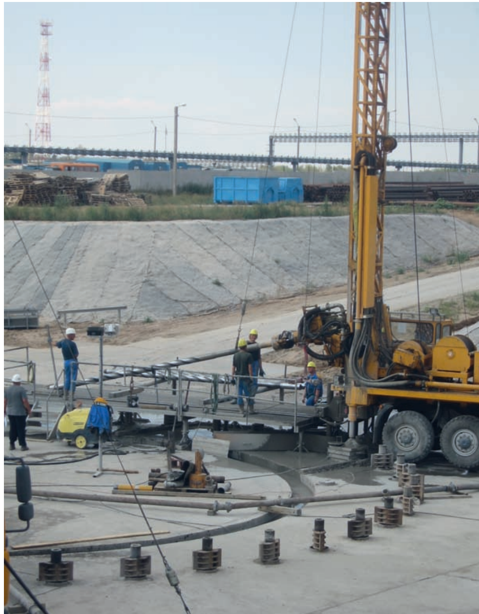
Drilling of the freezing holes
